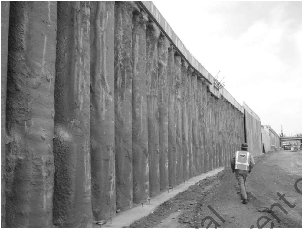
Photo 1. Example of a drilled shaft wall.
