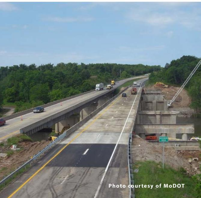
**Quality.** The use of a pre-constructed superstructure can improve quality by eliminating deck construction joints and girder camber problems associated with phased construction. In addition, it is possible to get a better concrete cure when the superstructure is constructed off-line.
