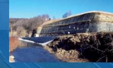
he Mae West Bend Project improved a sharp bend on Route 8 in Etna, PA. Due to its urban setting, the contractor was presented with a number of design and construction challenges including the restriction of blasting and realigning a road between a 100-foot high rock slope and a trout-stocked recreational stream in a commercial setting. Using a T-Wall (an interlocking retaining wall system), the contractor was able to minimize cost and time. This project met or exceeded all of PennDOT's needs,
