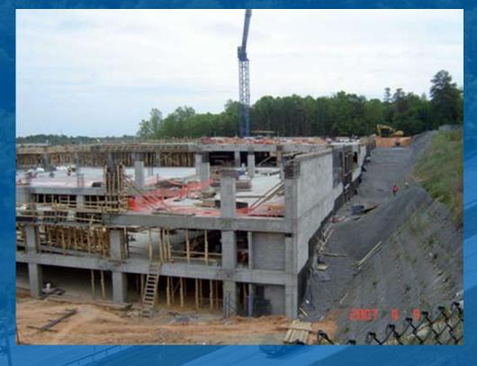
School. CATS proposed a win-win solution: a joint-use facility on the site. CATS would construct a 1,100-space parking deck that would be capped by a playing field on the deck's rooftop for the school's students. This design blends the deck into the environment, and eases congestion by taking more than 1,100 vehicles off of I-77 during rush hour.
