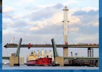
all four sides. This was one of the first two installations of a new cradle system developed for cablestayed bridges. The bridge also is the first in the world to utilize stainless steel cable-stay, sheathing, and internally lit glass pylon, and has the largest stays with 156 strands.
