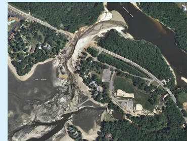
Devastation of washed out Trunk Highway A and empty lake
