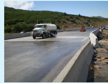
New bridge deck on Interstate 80
