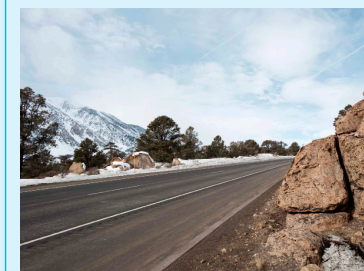
U.S. Route 395, Sherwin Summit Rehabilitation
