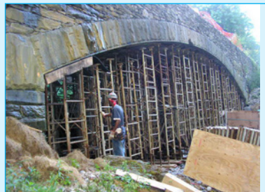
Installation of supports under masonry arch
