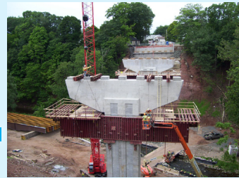
Construction of 400-foot tall bridge pier
