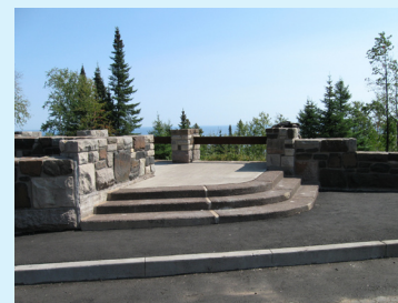
Rehabilitated overlook terrace with a view of Lake Superior
