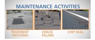
Maintenance activities to keep facilities in good repair do not require accessibility modifications. Examples of pavement maintenance treatments are chip seals, crack filling, and pavement patching.
