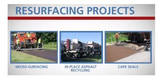
Resurfacing projects are not always simple asphalt overlays. Micro-surfacing, in-place asphalt recycling, and cape seals are resurfacing treatments that trigger the ADA requirements for curb ramp accessibility.
