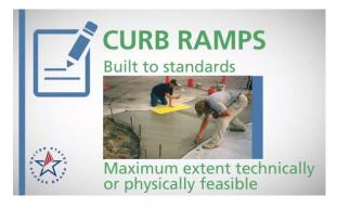
A curb ramp must be built in accordance with the standards to the maximum extent technically or physically feasible. Sometimes curb ramps cannot be fully compliant because of existing infrastructure, terrain characteristics, or environmentally sensitive areas. Agencies must document deviations from the standards, including the reasons why full compliance is not feasible.
