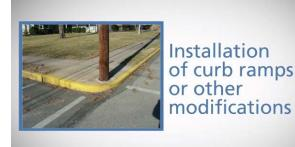
Accessibility laws and guidance require the installation of curb ramps or other modifications when a project alters a roadway. An alteration is a change that affects or could affect the usability of all or a part of a building or a facility. Alteration of roadways may include reconstruction, rehabilitation, and the widening of streets.
