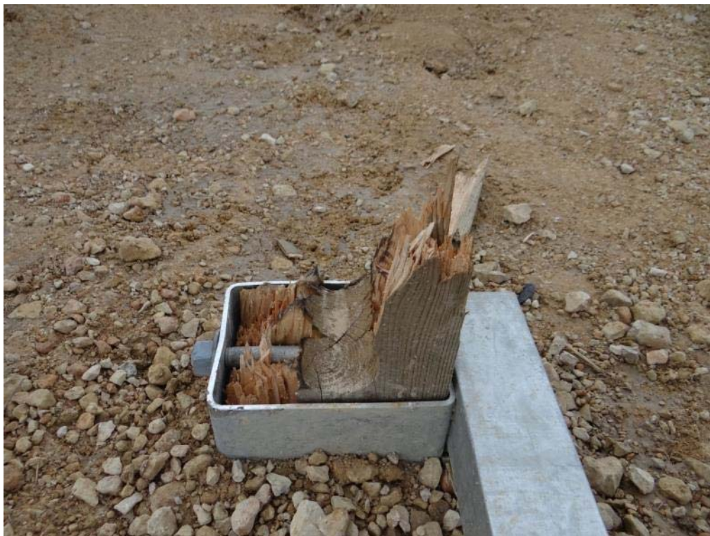
Figure 3.12: Post Test – Foundation Sleeve at Post 2
