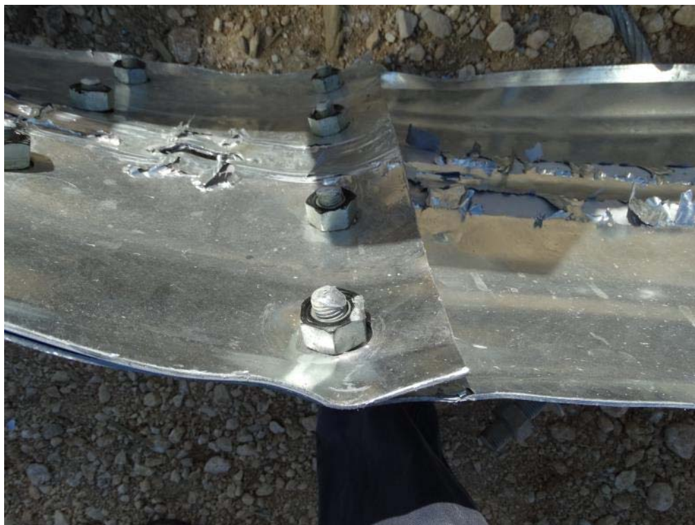
Figure 3.19: Post Test – Extruded Guardrail Splice
