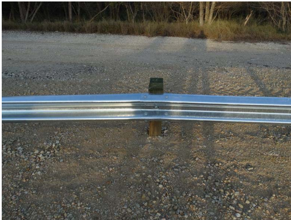
Figure 2.17: Post 22 Immediately Preceding Downstream Turndown Anchor
