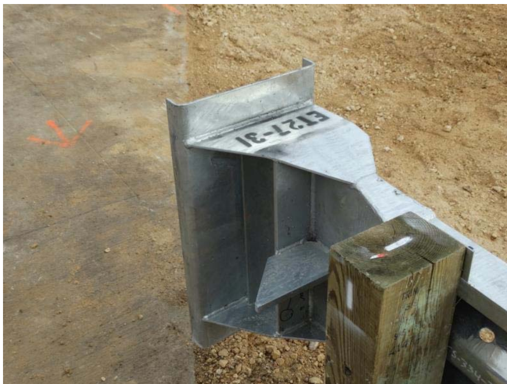
Figure 2.18: ET Plus Head Extruder Exit (see Appendix B for Dimensions)
