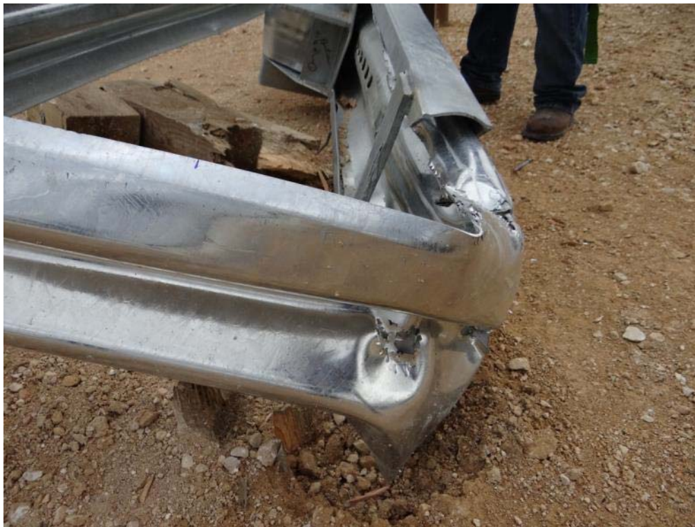
Figure 3.26: Post Test – ET Plus Head Guide Chute Entrance
