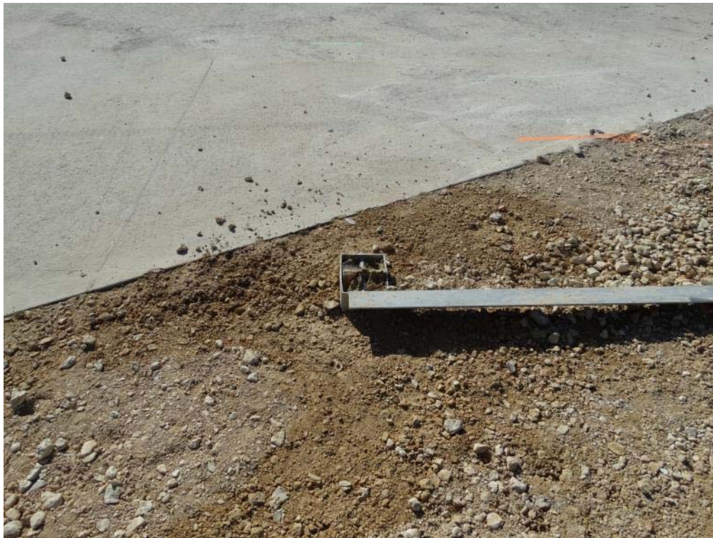
Figure 3.8: Post Test – Foundation Sleeve at Post 1
