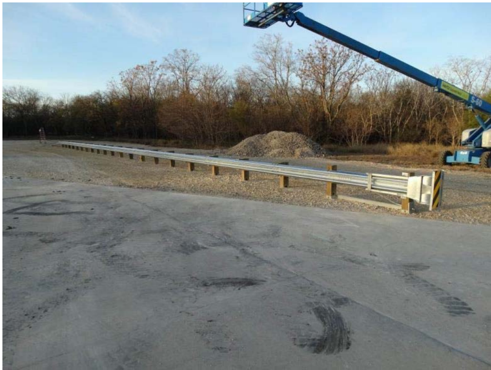
Figure 2.3: Test Installation for ET Plus Test ET27-30
