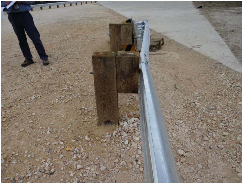
Figure 3.19: Post Test – Downstream View of Post 5
