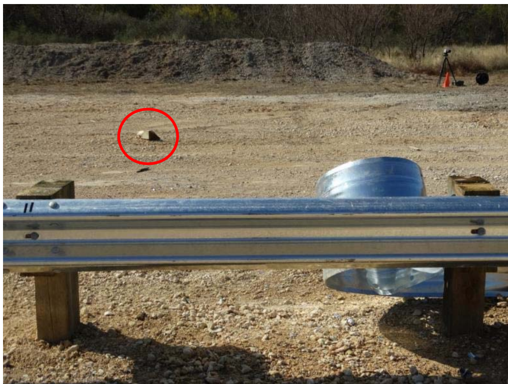
Figure 3.31: Post Test – Line Posts 10 & 11 and Debris
