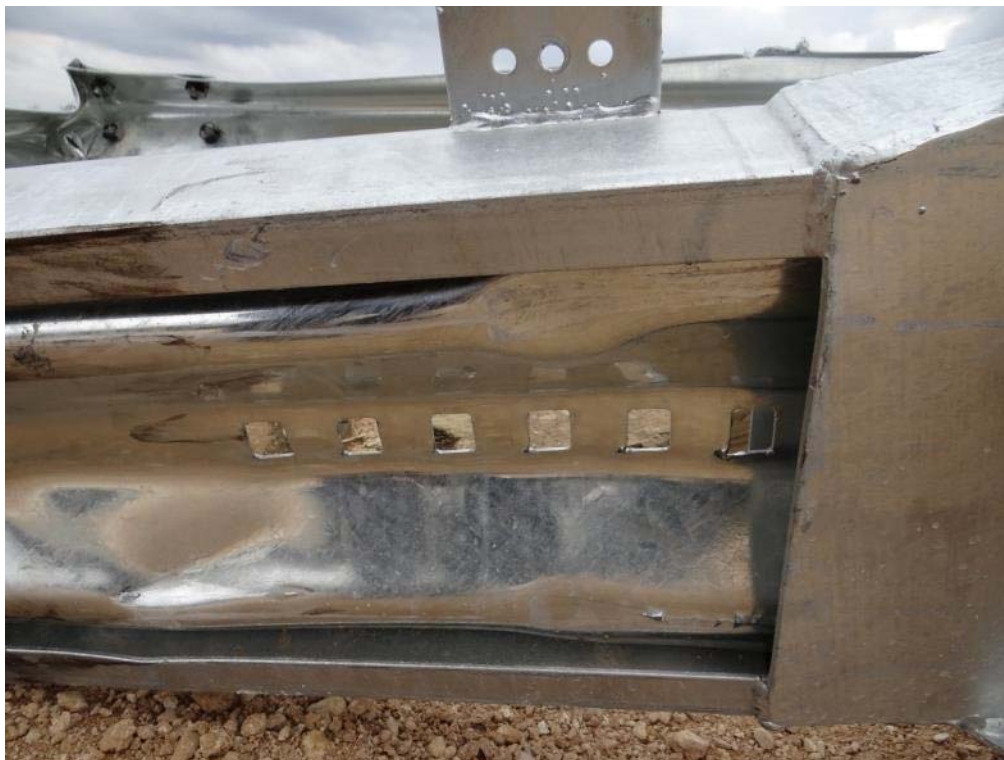
Figure 3.32: Post Test – ET Plus Head Guide Chute Exit, Traffic Side
