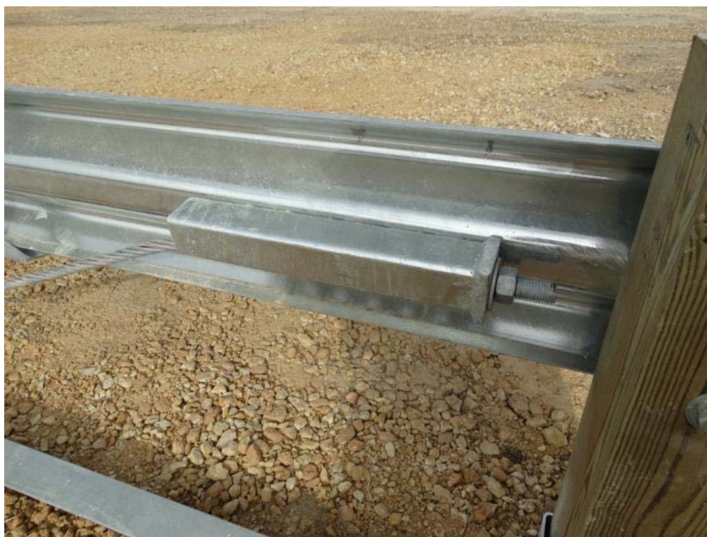
Figure 2.10: End Terminal Cable Anchor
