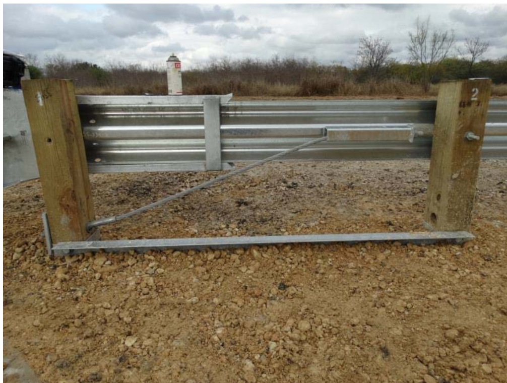
Figure 2.8: ET Plus Head and Anchor Cable Assembly
