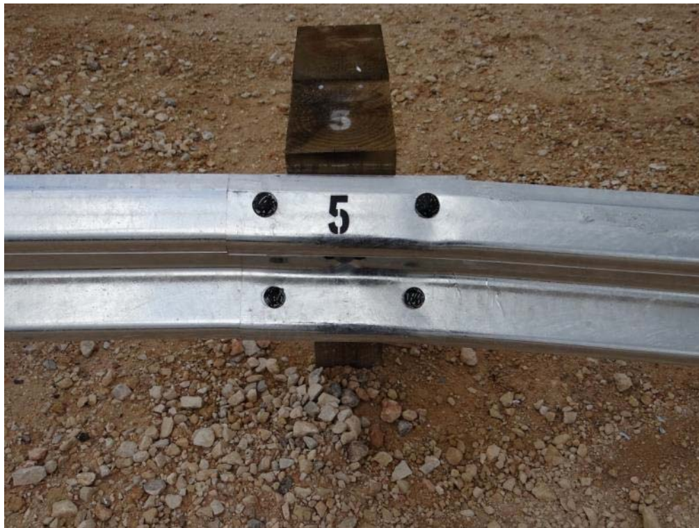
Figure 3.17: Post-Test – Traffic Side View of Splice at Post 5
