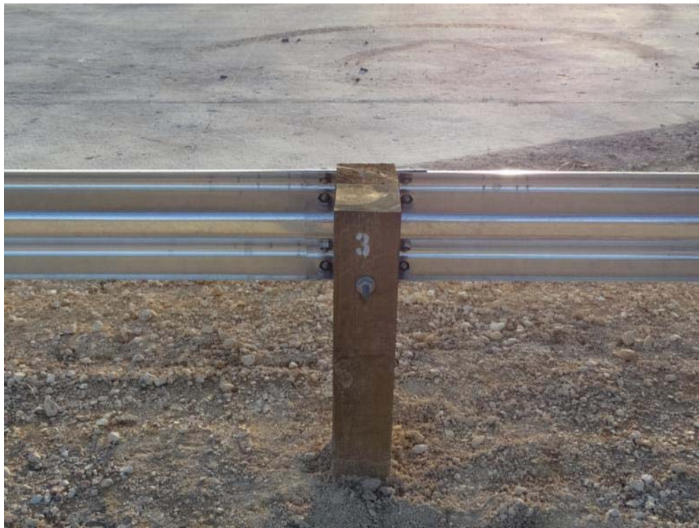
Figure 2.12: First Guardrail Panel Splice Joint – Non-Traffic Side
