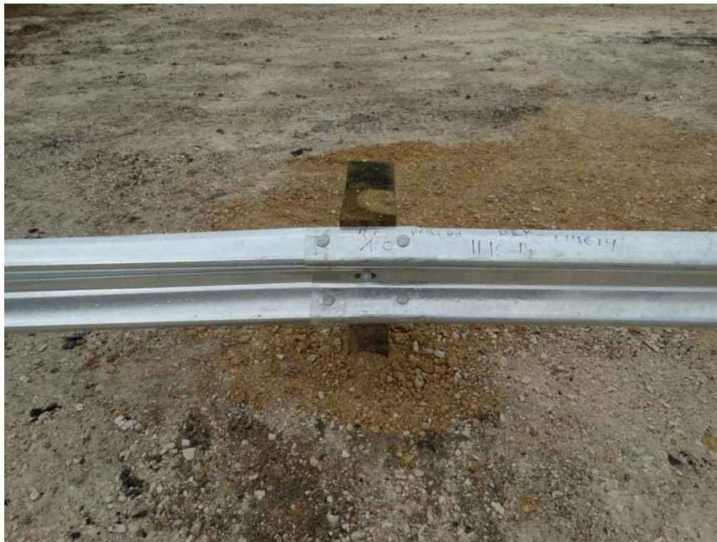
Figure 2.19: Post 22 Immediately Preceding Downstream Turndown Anchor
