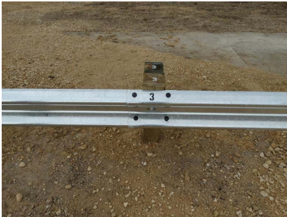
Figure 2.11: First Guardrail Panel Splice Joint – Traffic Side (Bolts Painted for Visibility in Video)
