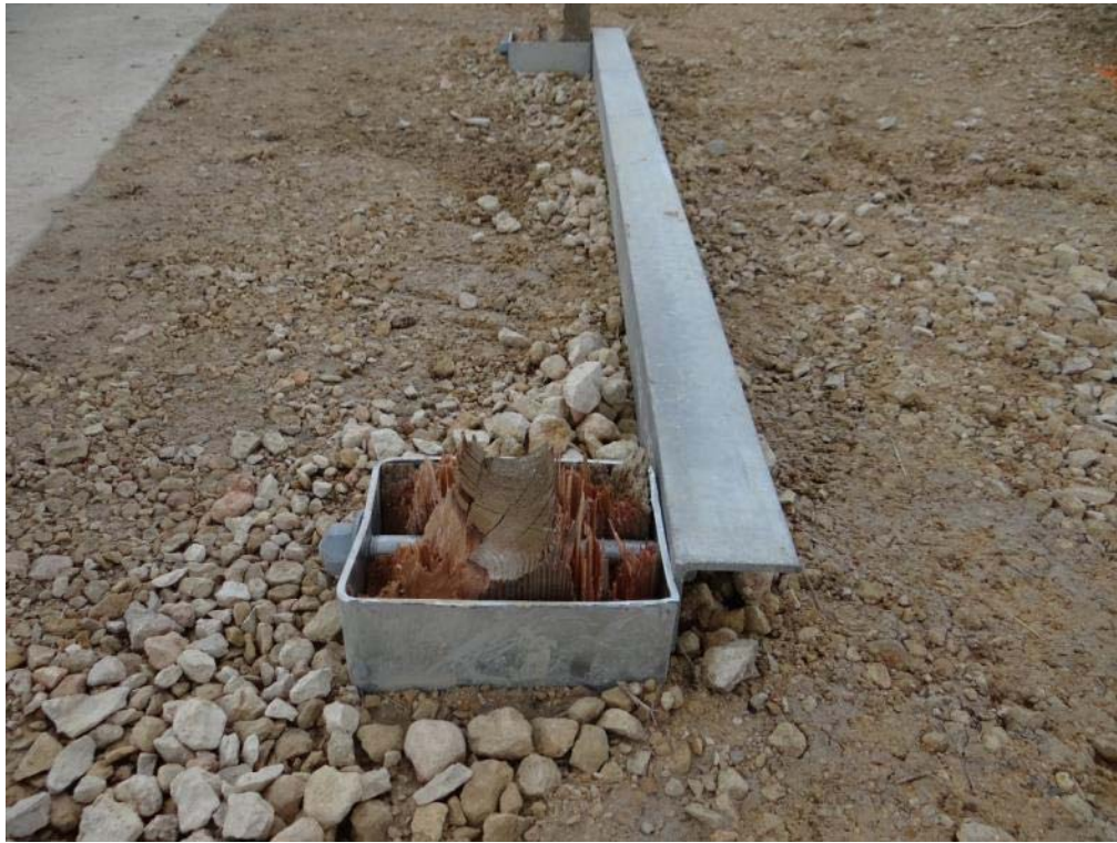
Figure 3.11: Post Test – Foundation Sleeve at Post 1
