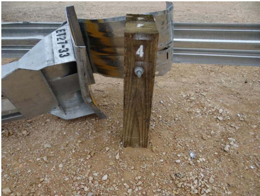
Figure 3.15: Post Test – View of Post 4 from Non-Traffic Side
