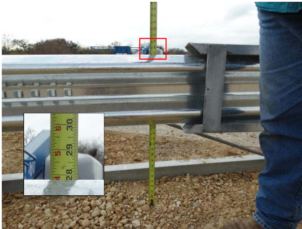
Figure 2.7: Measurement of Guardrail Installation Height
