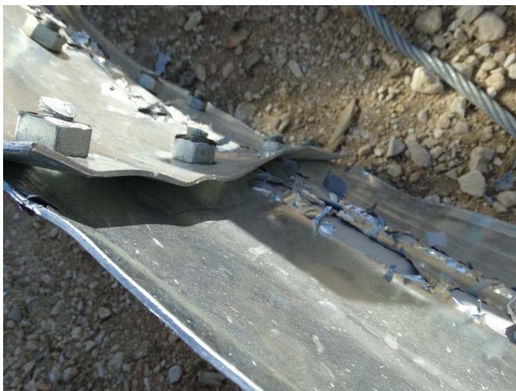
Figure 3.20: Post Test – Extruded Guardrail Splice
