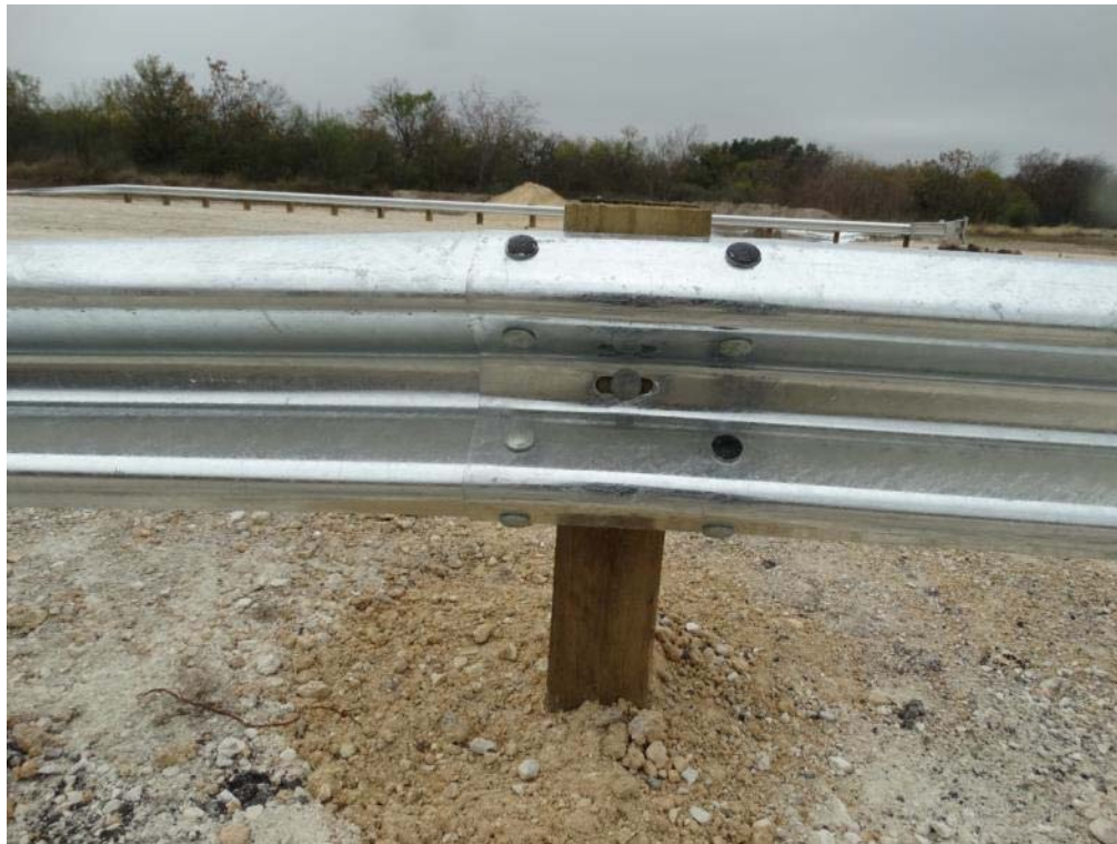
Figure 2.17: Post 22 Immediately Preceding Downstream Turndown Anchor
