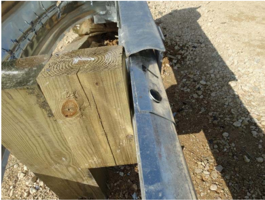
Figure 3.20: Post Test – Extruder Head at Post 7, Top View
