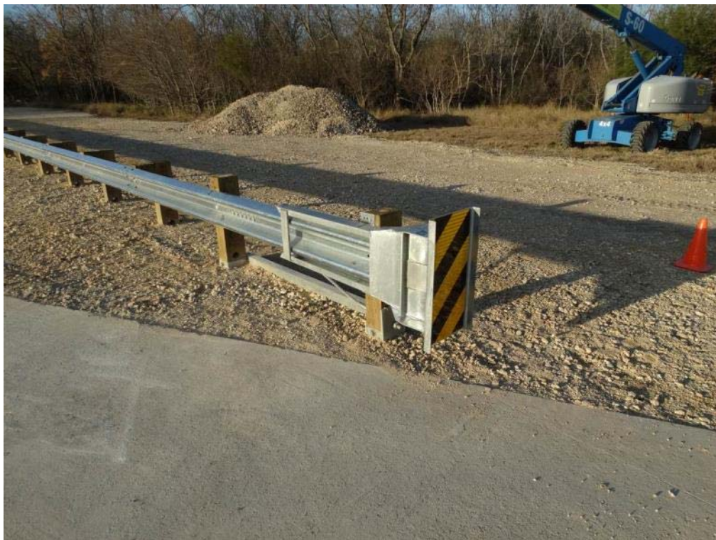
Figure 2.4: ET Plus End Terminal
