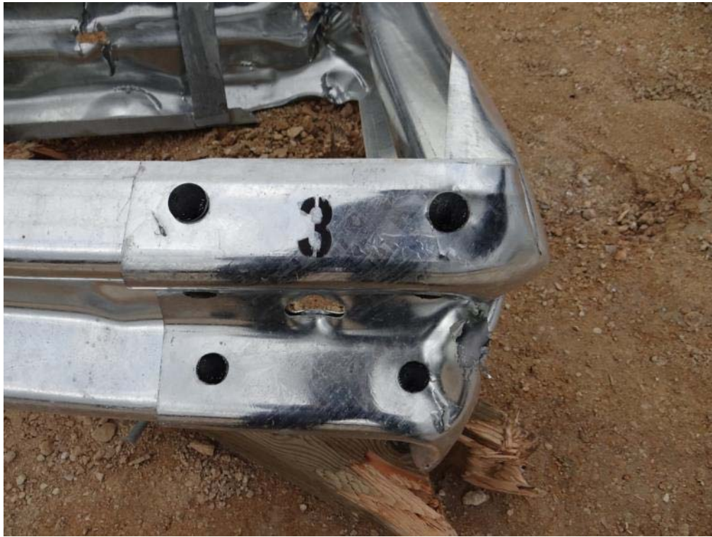
Figure 3.13: Post Test – First Splice at Post 3 (Splice Bolts Painted for Visibility in Video)
