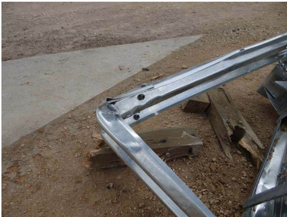
Figure 3.22: Post Test – First Splice at Post 3 from Non-Traffic Side
