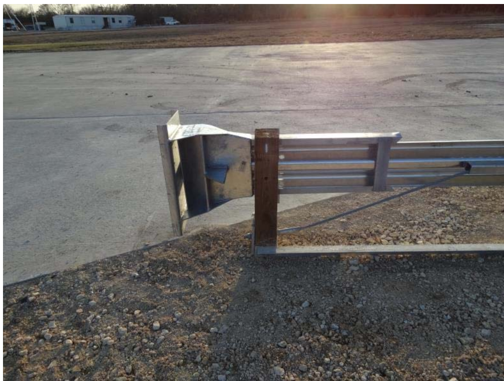
Figure 2.14: ET Plus Head and Post 1 – Non-Traffic Side
