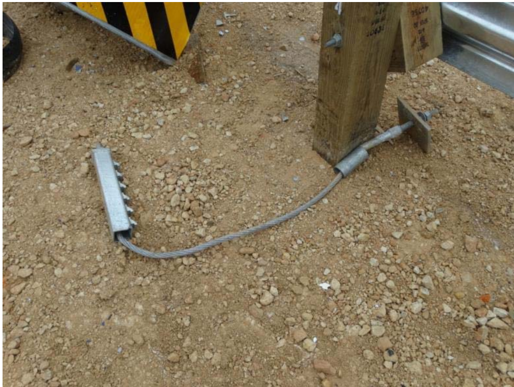
Figure 3.26: Post Test Location of Anchor Cable at Post 4
