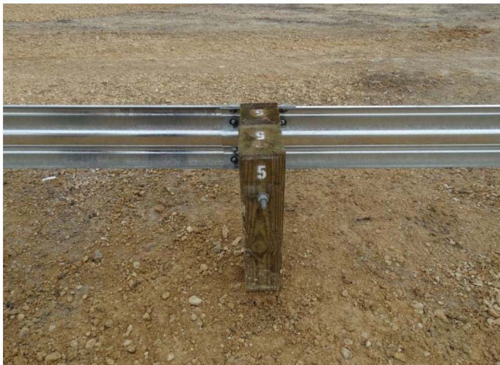
Figure 2.14: Second Guardrail Panel Splice Joint – Back Side (Nuts Painted for Visibility in Video)
