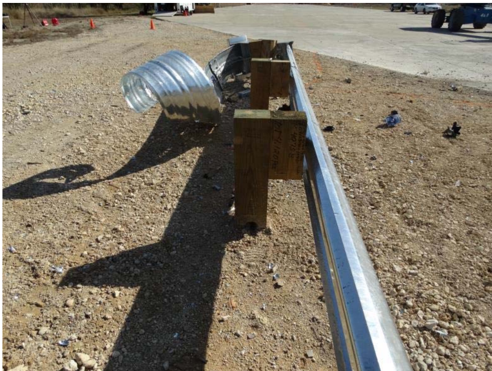
Figure 3.22: Post Test – Upstream of Posts 4, 5 and 6
