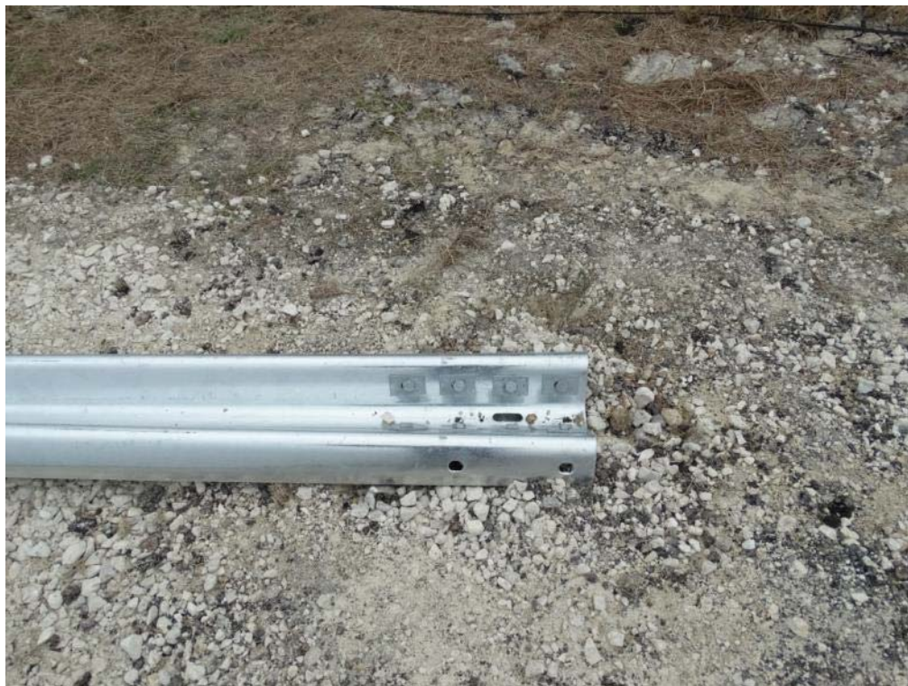
Figure 2.18: Downstream Turndown Anchor
