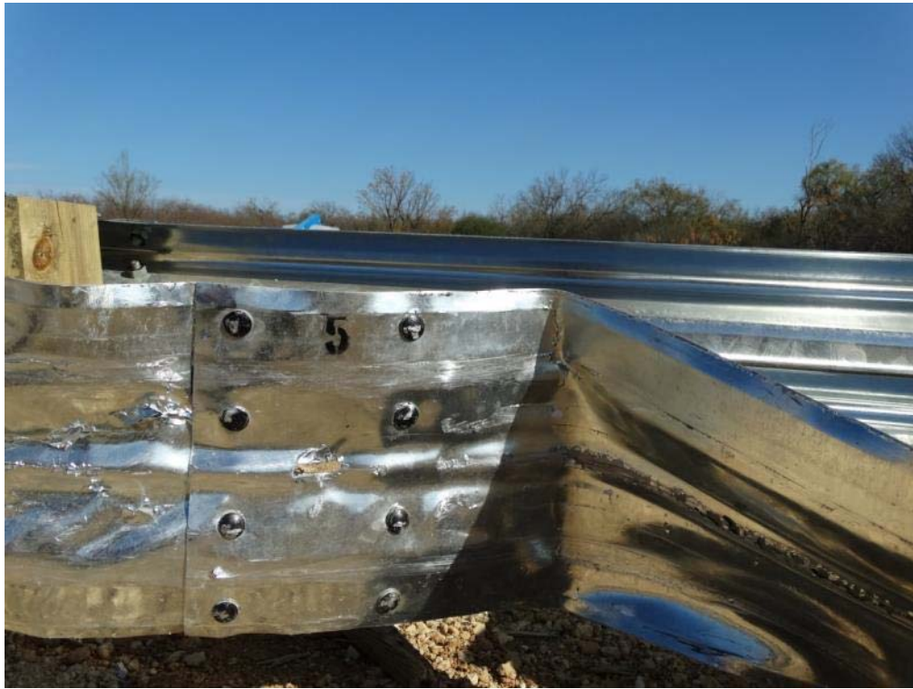
Figure 3.28: Post Test – Extruded Guardrail Splice from Post 5, Splice Bolts
