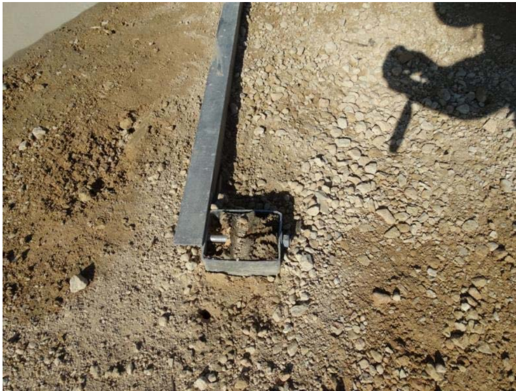
Figure 3.10: Post Test – Post 2 Foundation Sleeve
