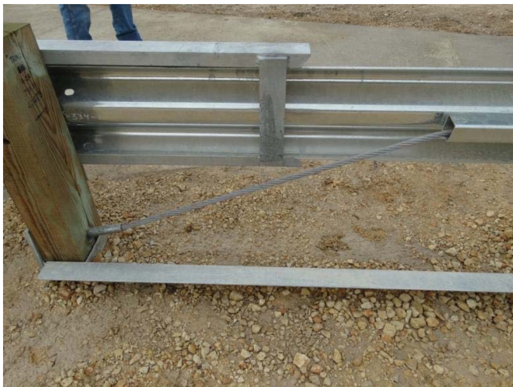
Figure 2.8: ET Plus Head and Anchor Cable Assembly
