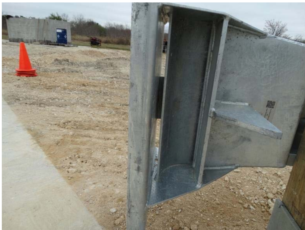
Figure 2.16: ET Plus Head Extruder Exit (see Appendix B for Dimensions)
