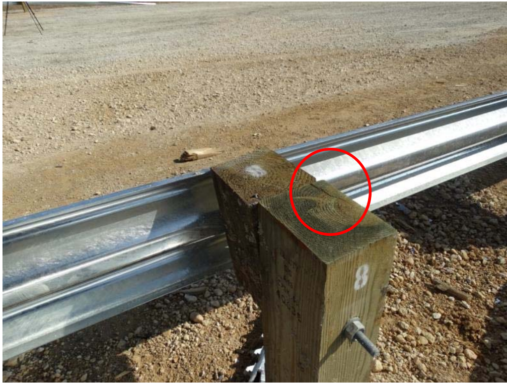
Figure 3.14: Post Test – Post 8 Cracked, Blockout Twisted
