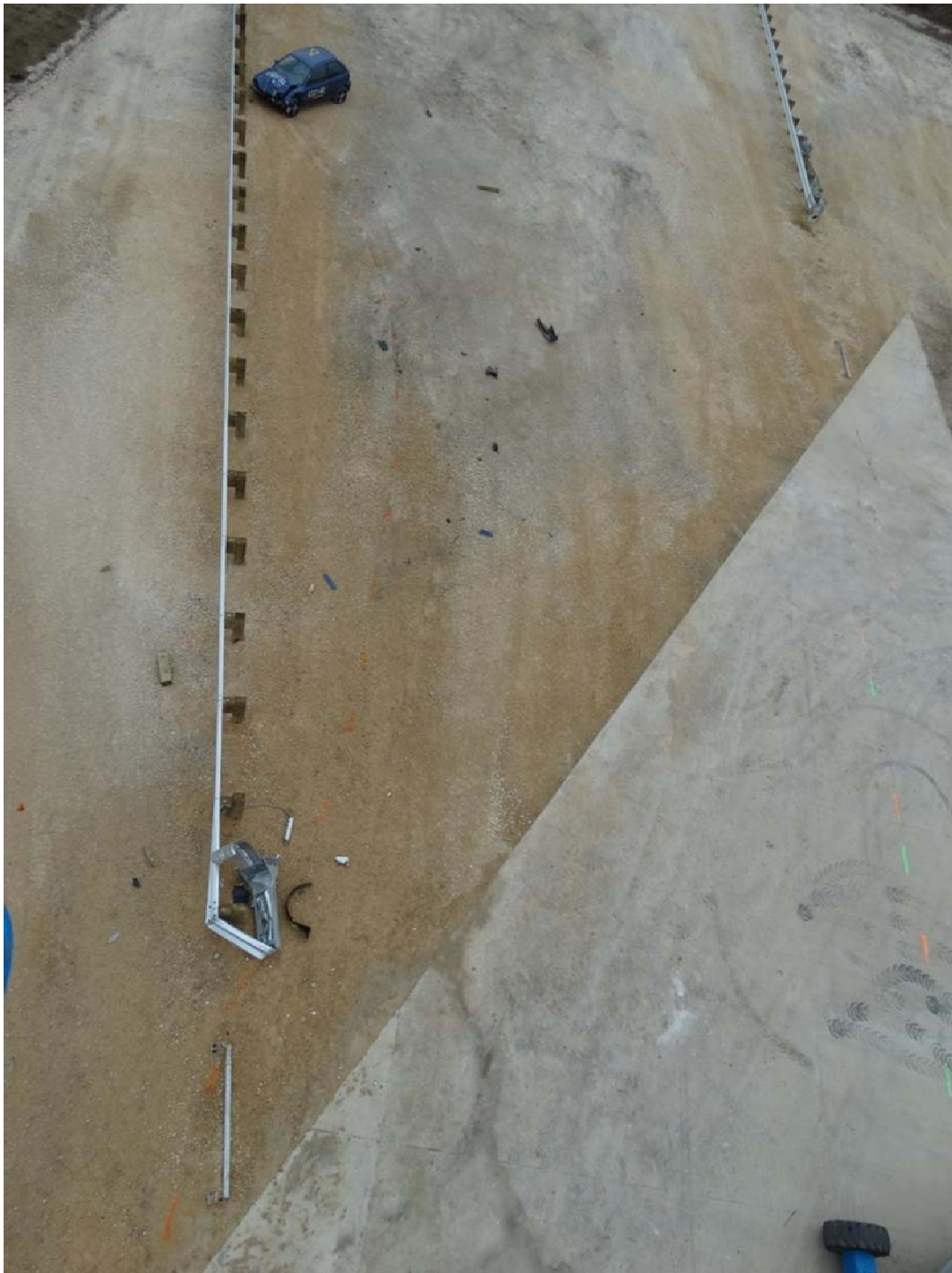
Figure 3.2: Post-Impact Condition of the Test Article and Vehicle
