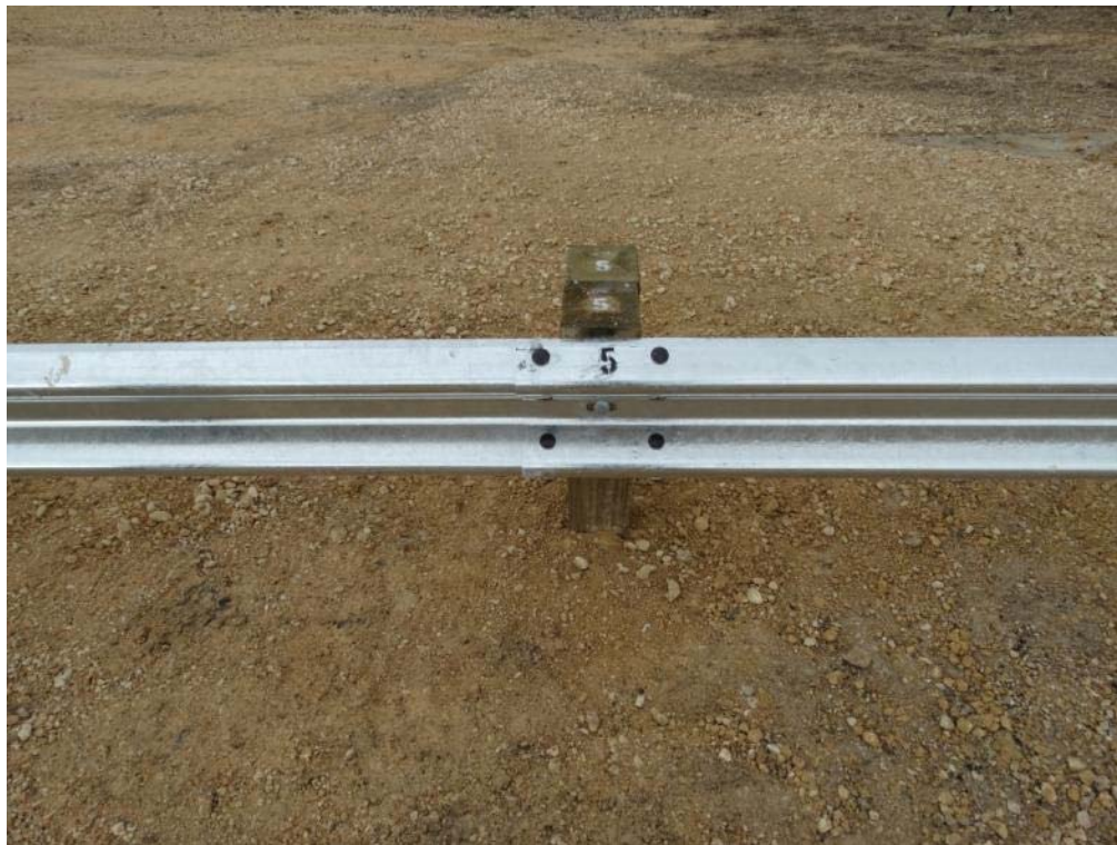
Figure 2.13: Second Guardrail Panel Splice Joint – Traffic Side (Bolts Painted for Visibility in Video)
