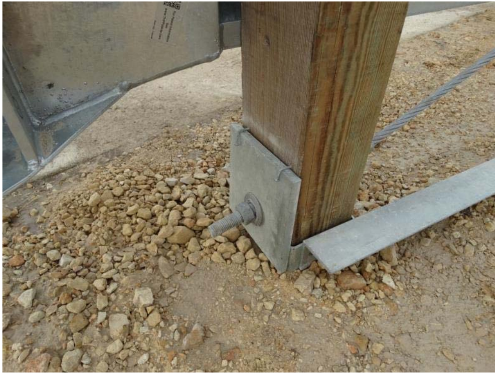
Figure 2.9: End Terminal Anchor Cable Mount – Post 1
