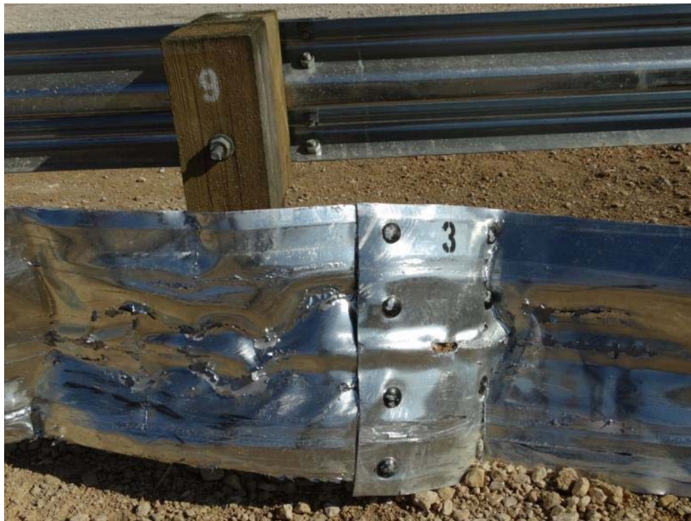
Figure 3.26: Post Test – Extruded Guardrail Splice from Post 3, Splice Bolts
