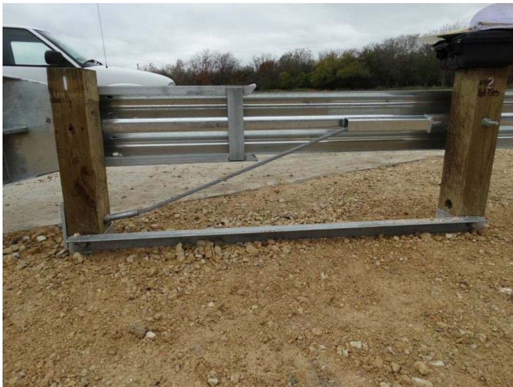
Figure 2.8: ET Plus Head and Anchor Cable Assembly
