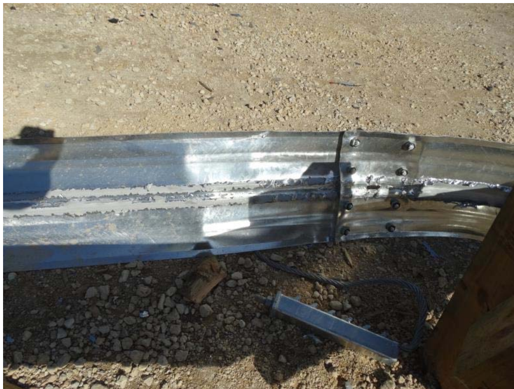
Figure 3.18: Post Test – Extruded Guardrail Splice
