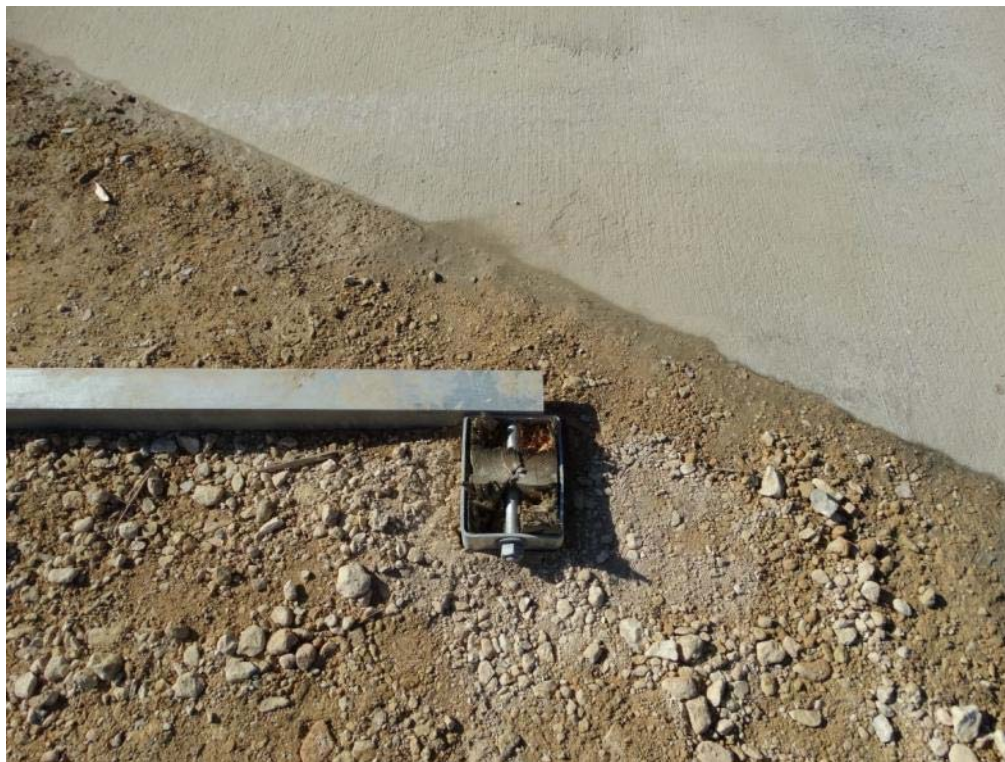
Figure 3.9: Post Test – Post 1 Foundation Sleeve
