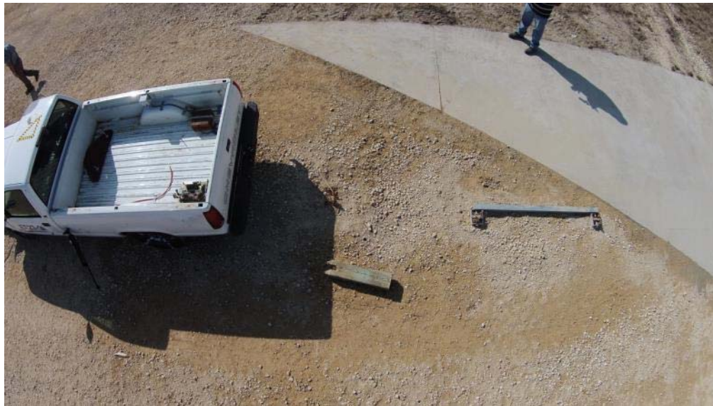
Figure 3.8: Post Test – Post 1 and 2 Foundation Sleeves and Strut
