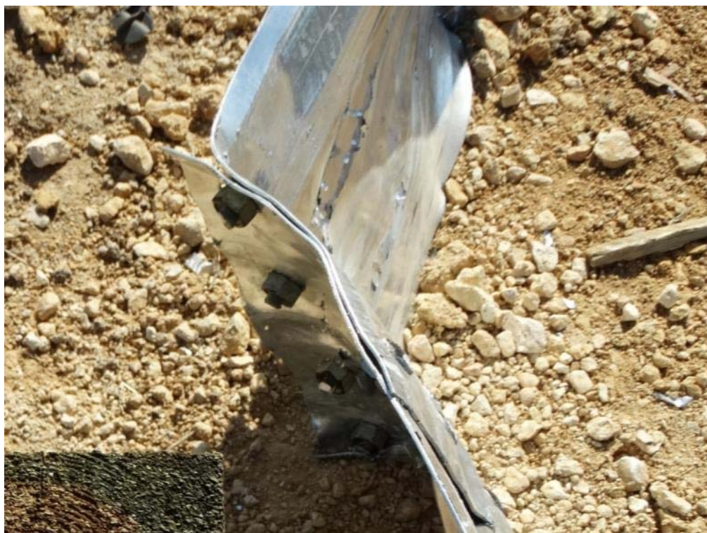
Figure 3.27: Post Test – Extruded Guardrail Splice from Post 3, Splice Nuts
