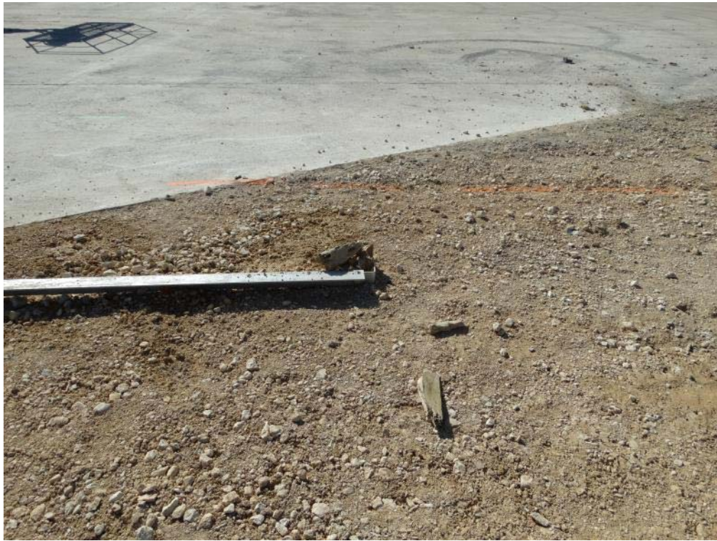
Figure 3.9: Post Test – Foundation Sleeve at Post 2
