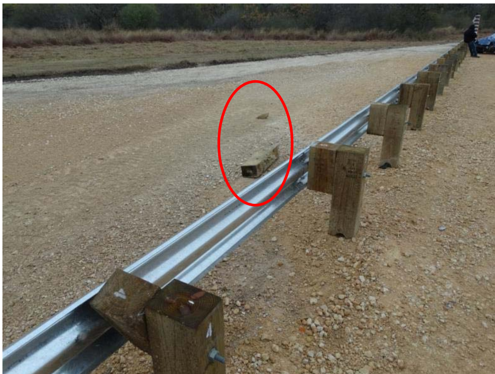
Figure 3.24: Post Test – Debris on Traffic Side
