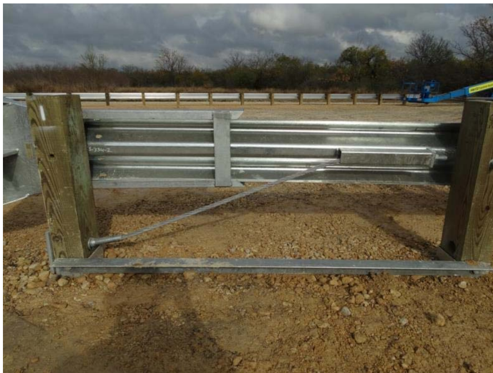
Figure 2.8: ET Plus Head and Anchor Cable Assembly
