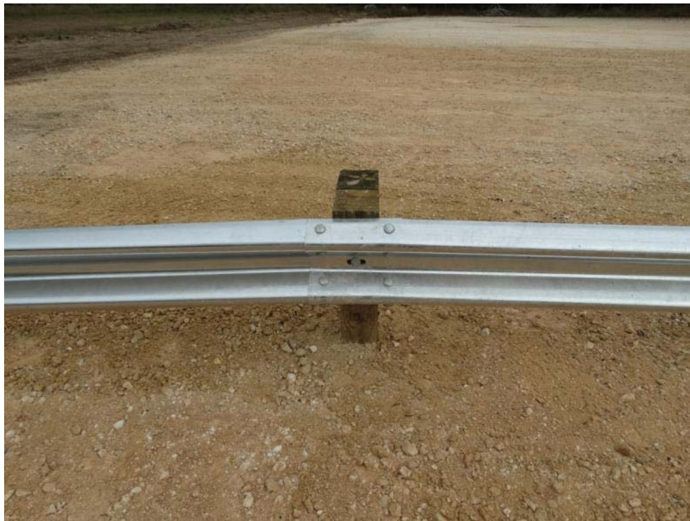
Figure 2.17: Post 22 Immediately Preceding Downstream Turndown Anchor
