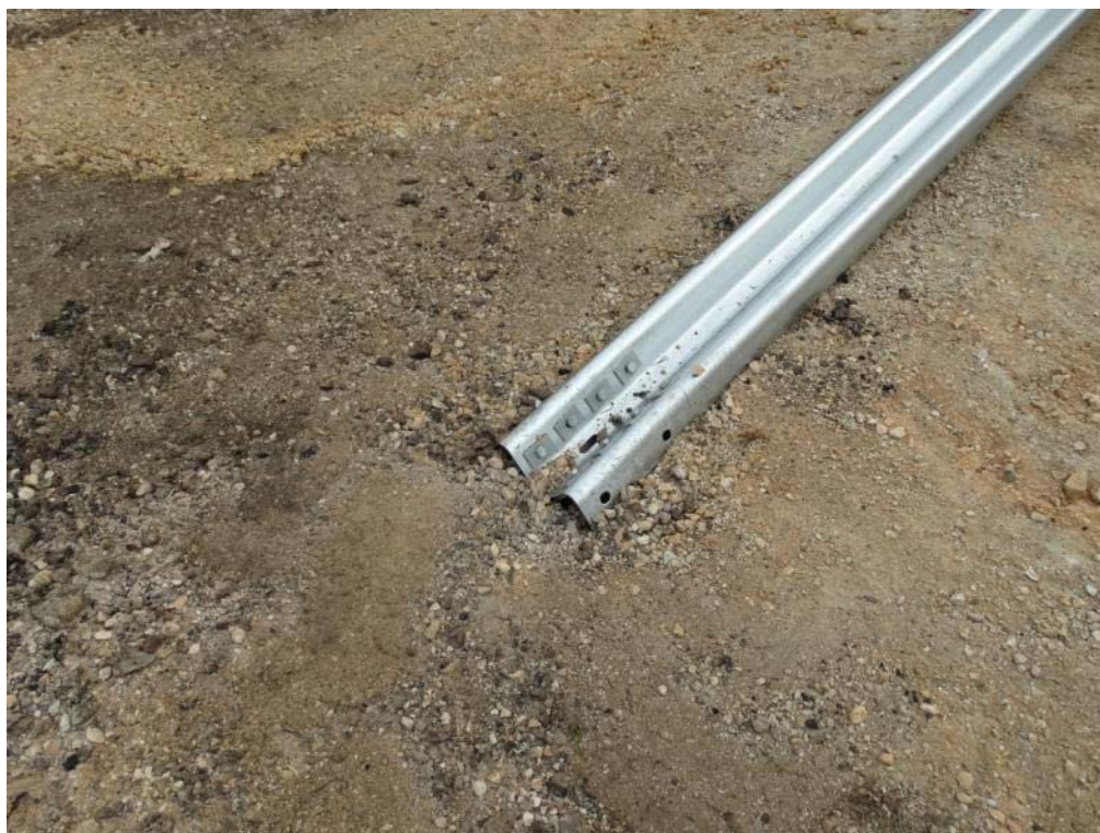
Figure 2.18: Downstream Turndown Anchor
