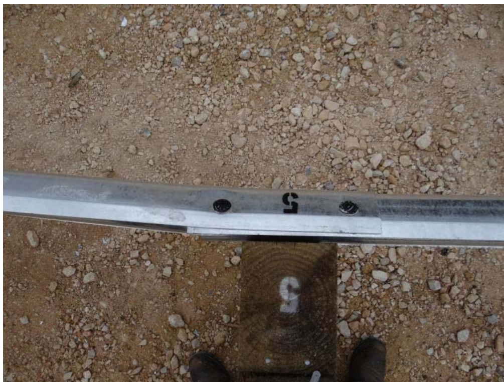
Figure 3.18: Post Test – Top View of Post 5
