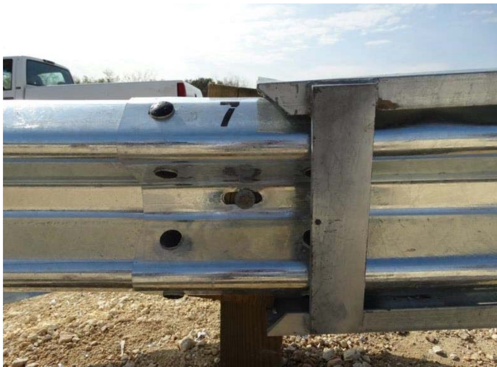
Figure 3.19: Post Test – Extruder Head at Post 7 (Splice Bolts Painted for Visibility in Video)
