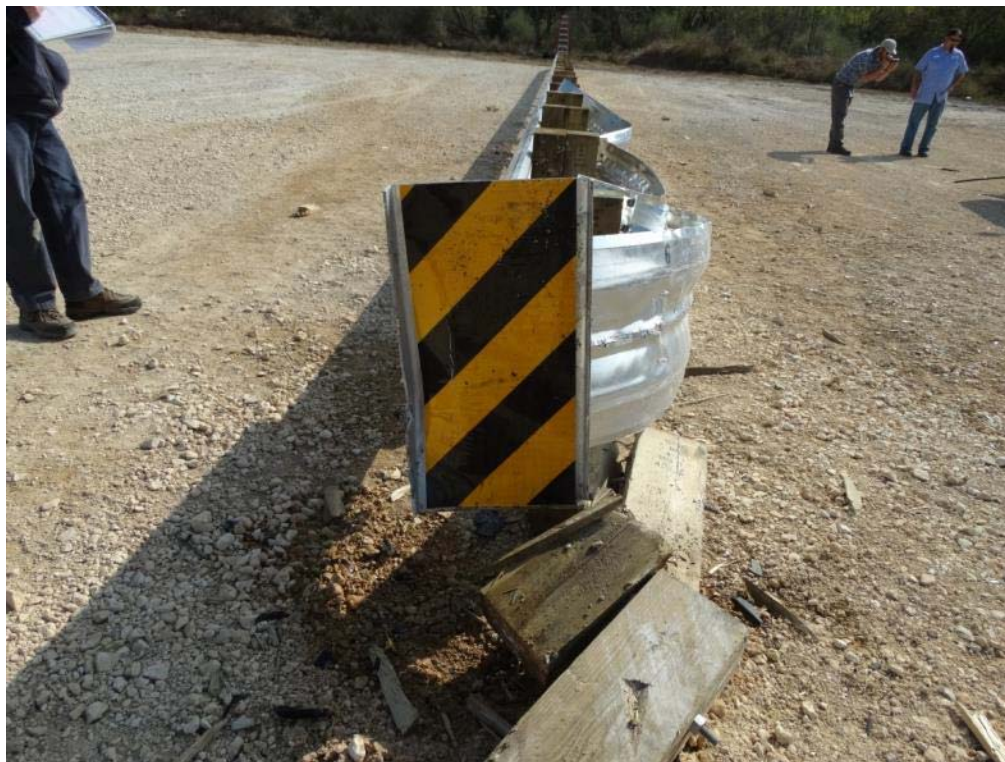
Figure 3.33: Post-Impact Test Article after Vehicle Removed
