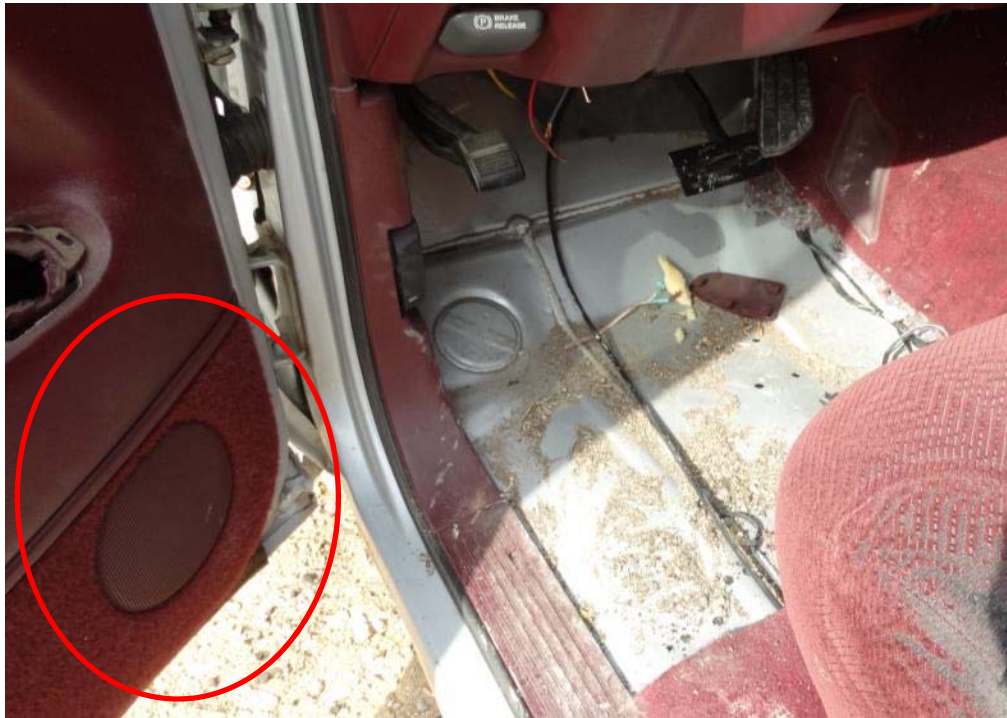
Figure 3.49: Door Panel Intact Behind Tear in Door Skin
