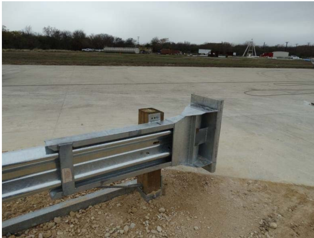
Figure 2.13: ET Plus Head and Post 1 – Traffic Side
