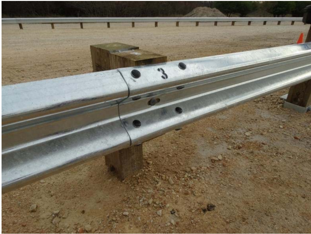
Figure 2.11: First Guardrail Panel Splice Joint – Traffic Side (Splice Bolts Painted for Visibility in Video)
