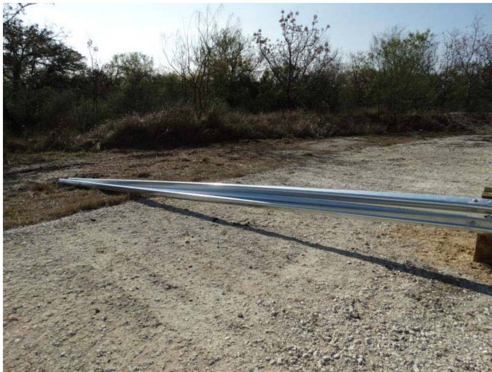
Figure 2.20: Downstream Turndown Anchor
