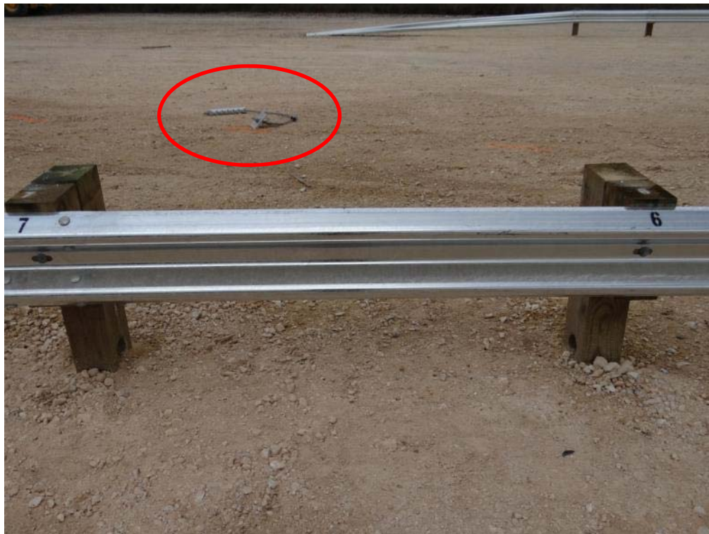
Figure 3.37: Post-Test Location of Anchor Cable
