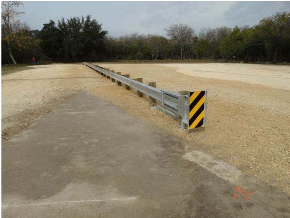
Figure 2.3: Test Installation for ET Plus Test ET27-33
