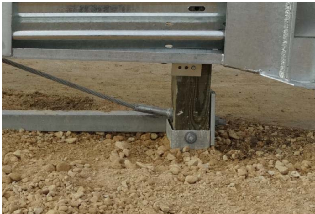
Figure 2.9: End Terminal Anchor Cable Mount – Post 1
