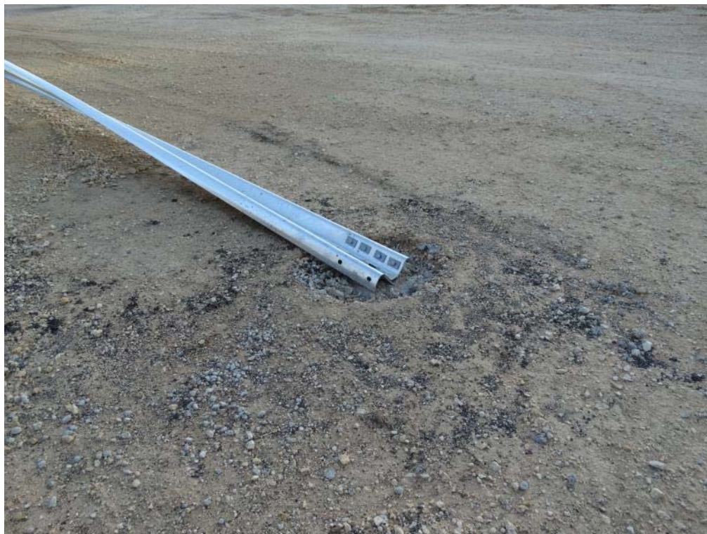
Figure 2.18: Downstream Turndown Anchor
