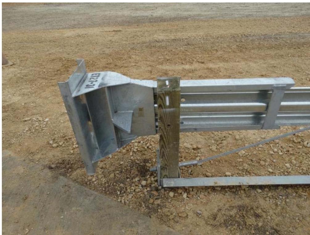
Figure 2.16: ET Plus Head and Post 1 – Back Side
