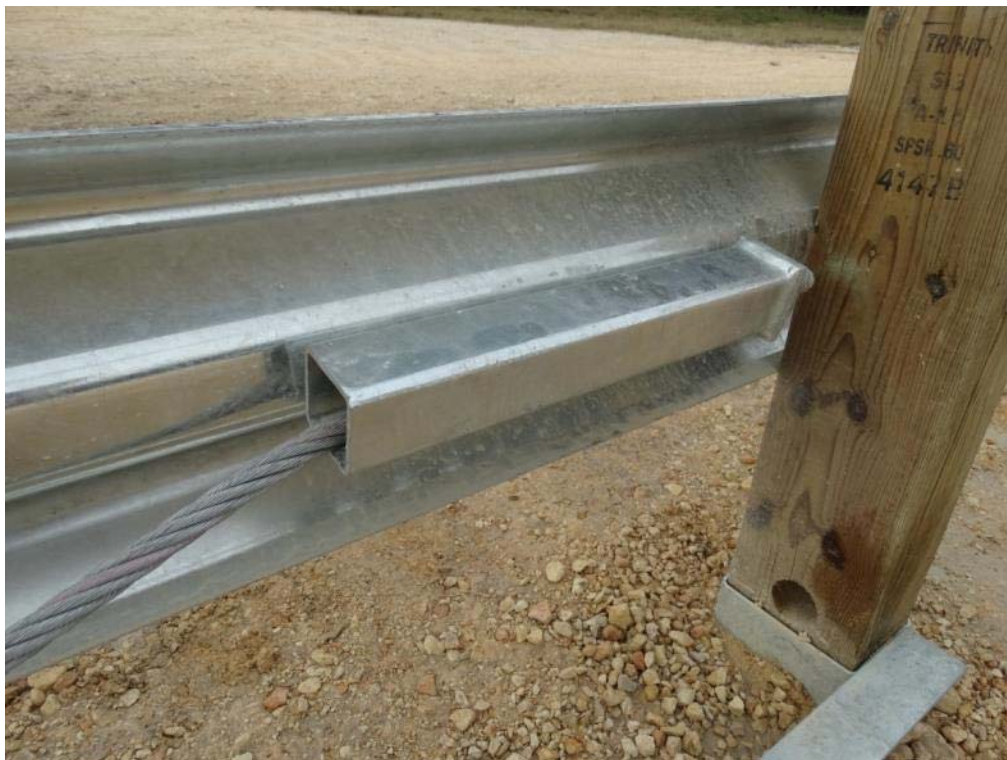
Figure 2.10: End Terminal Cable Anchor
