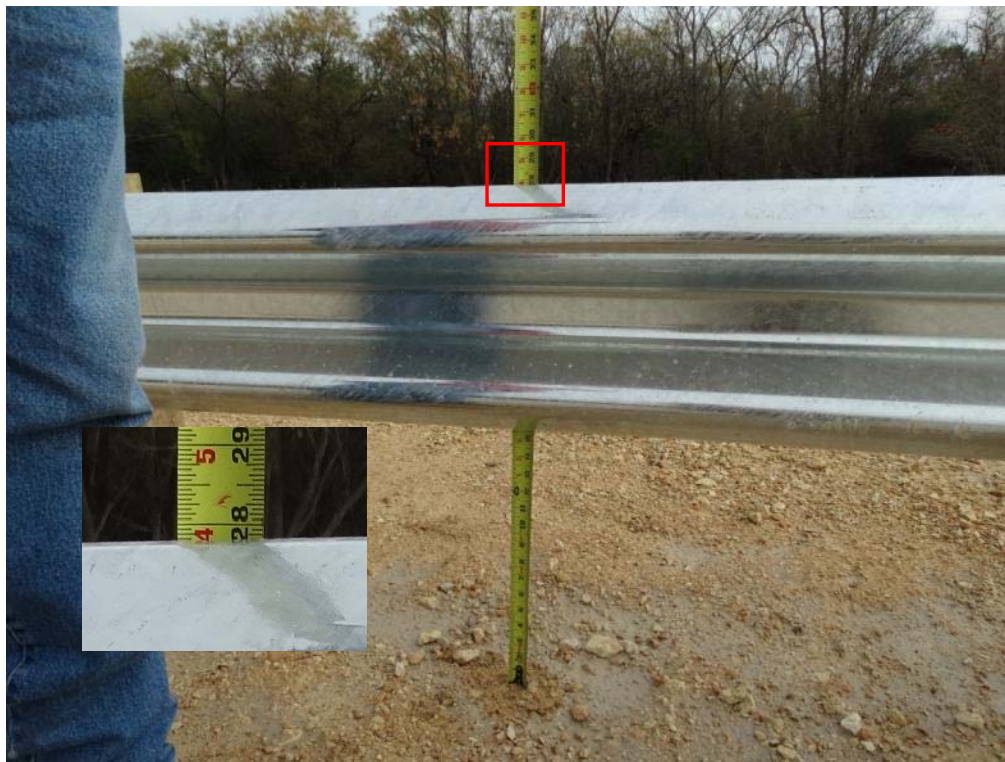
Figure 2.7: Measurement of Guardrail Installation Height
