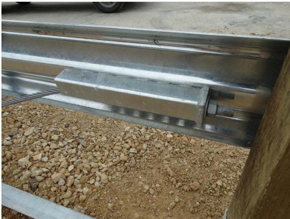
Figure 2.10: End Terminal Cable Anchor
