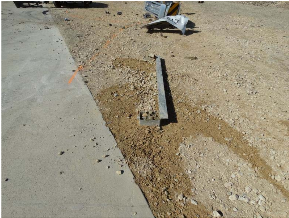
Figure 3.7: Post Test – Foundation Sleeves at Posts 1 and 2
