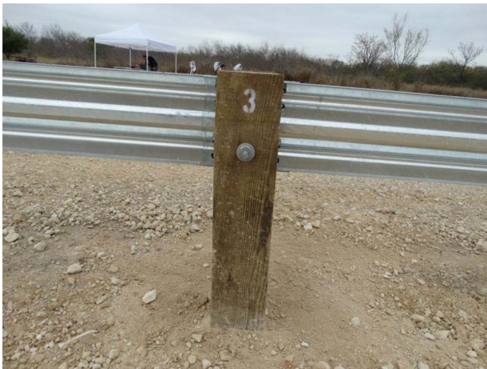
Figure 2.12: First Guardrail Panel Splice Joint – Back Side (Nuts Painted for Visibility in Video)
