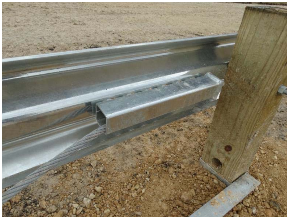
Figure 2.10: End Terminal Cable Anchor
