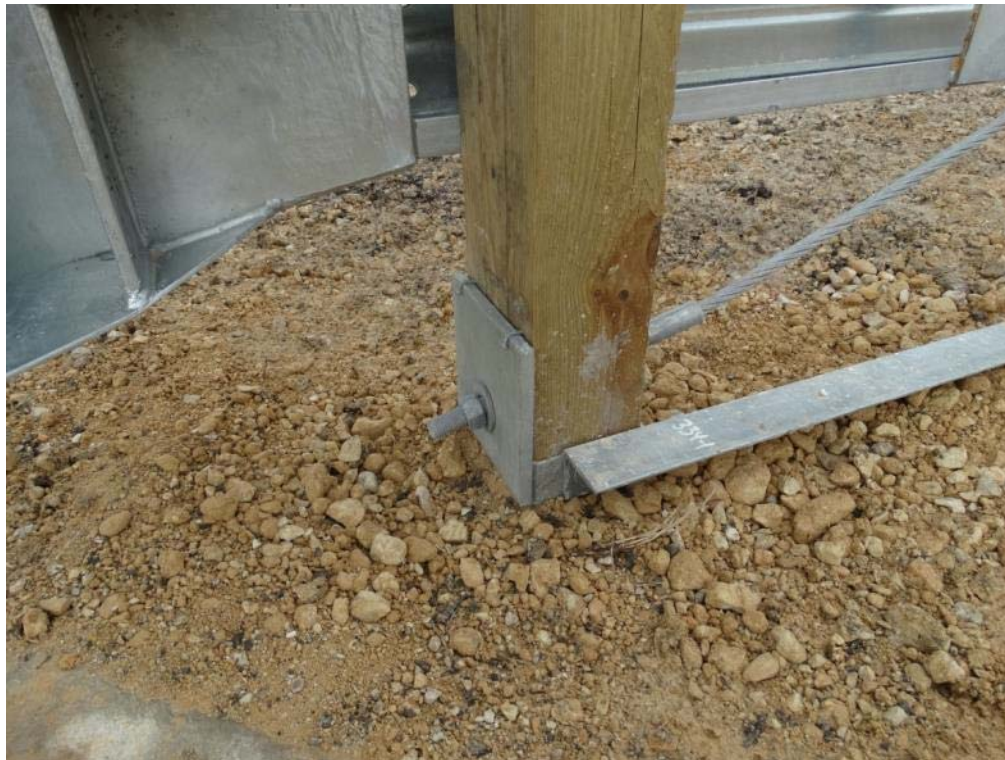
Figure 2.9: End Terminal Anchor Cable Mount – Post 1
