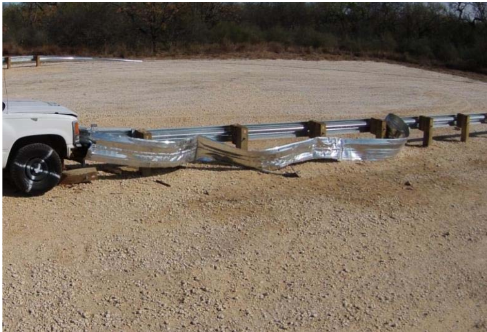
Figure 3.24: Post Test – Extruded Guardrail
