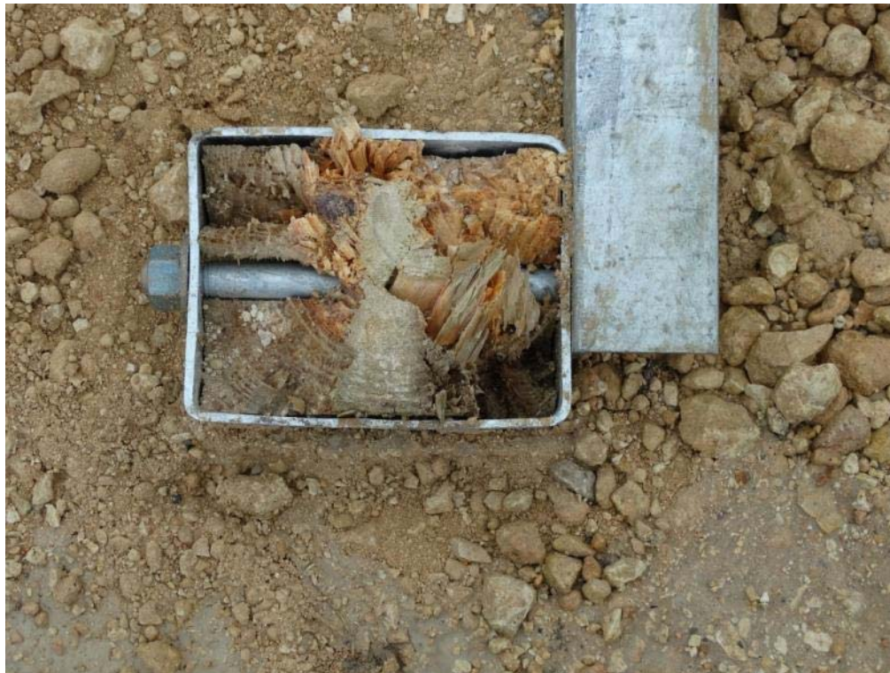
Figure 3.8: Post Test – Foundation Sleeve at Post 1
