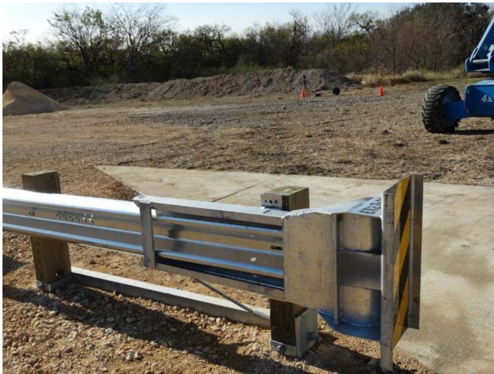
Figure 2.4: ET Plus End Terminal
