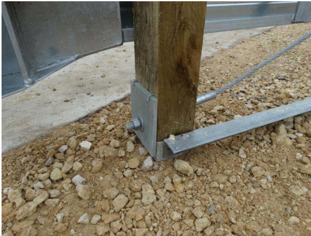
Figure 2.9: End Terminal Anchor Cable Mount – Post 1
