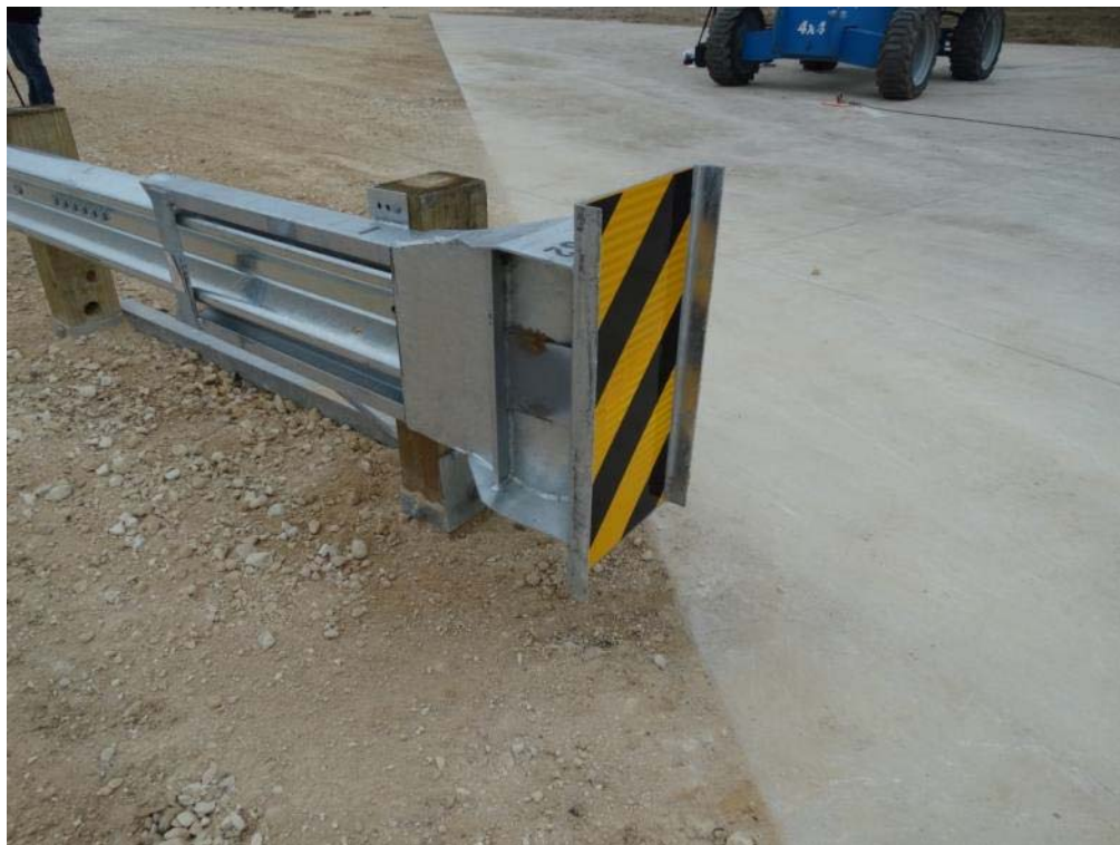
Figure 2.4: ET Plus End Terminal
