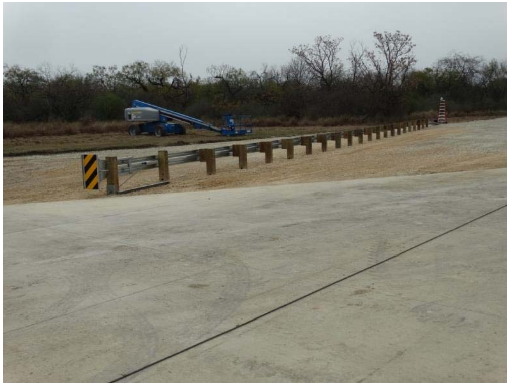
Figure 2.3: Test Installation for ET Plus Test ET27-32
