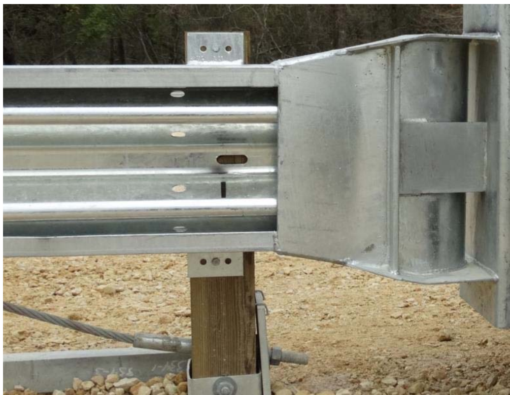
Figure 2.14: ET Plus Head and Post 1 – Close-up
