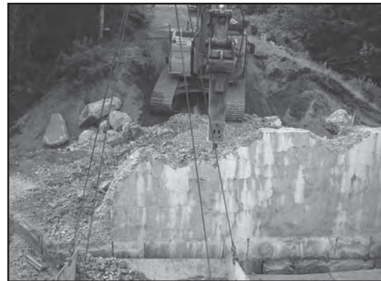
Saving the old abutments and using precast components to replace the Lamson Bridge in Maine cut construction time from nine months to ninety days.
