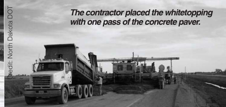
North Dakota's new concrete whitetopping uses the strength of the underlying asphalt base.
