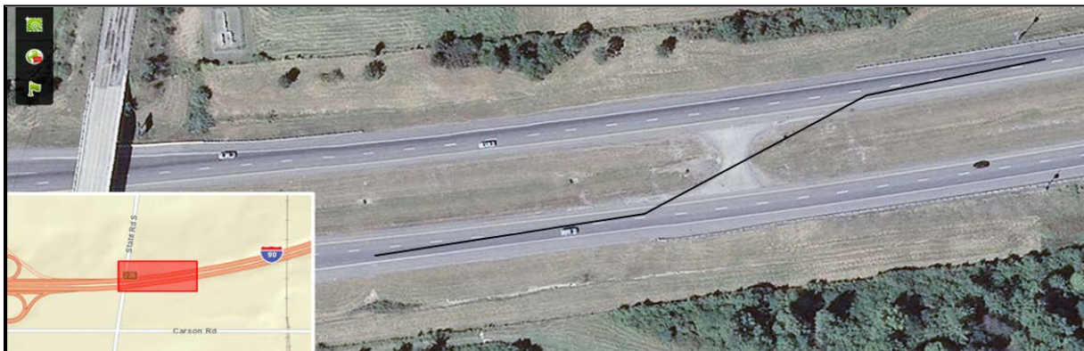
Figure 19. Photo. AWP treatment location on I-90.
