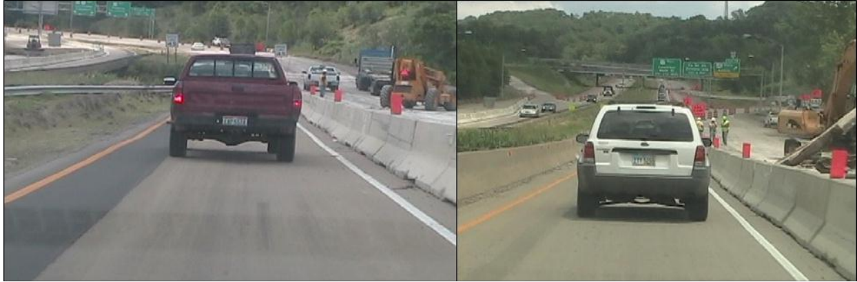
Figure 16. Photos. The AWP (left) and standard pavement marking (right) work zones on eastbound US-32/33/50 during the day.
