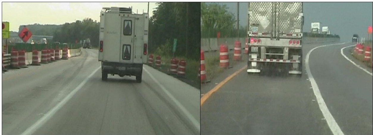
Figure 21. Photos. View of the AWP (left) and standard pavement marking (right) double-lane crossover.
