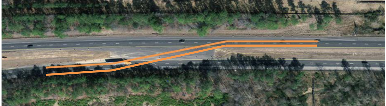
Figure 8. Photo. Aerial view of northern crossover. Southbound traffic shifts to northbound side divided by a jersey barrier.
