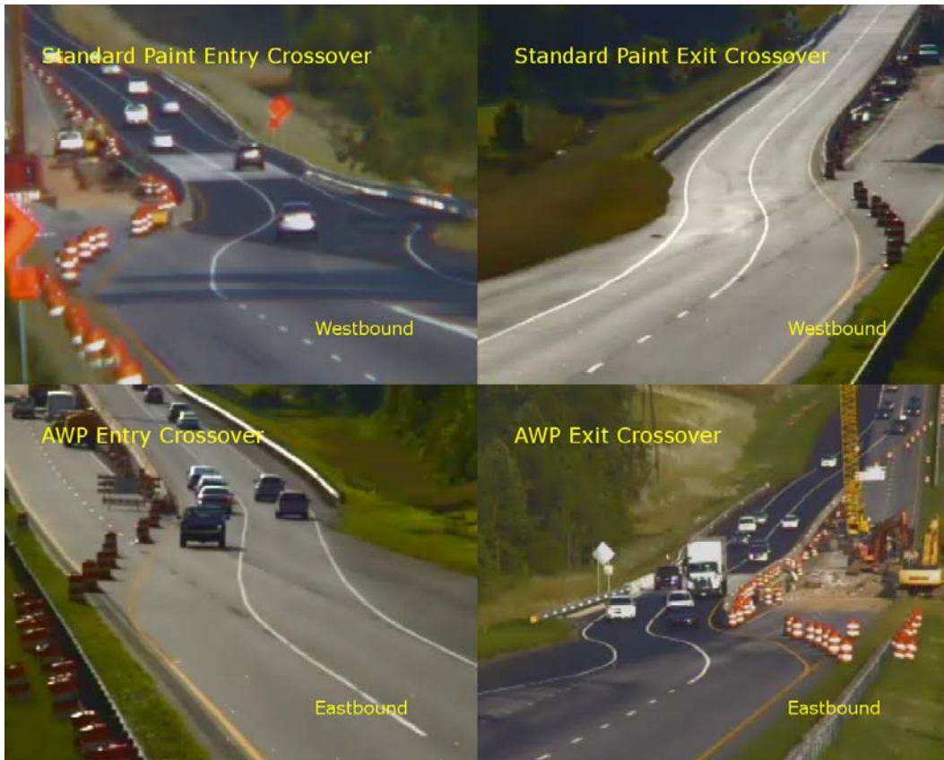
Figure 14. Photos. Four curves at the US-421 test site.
