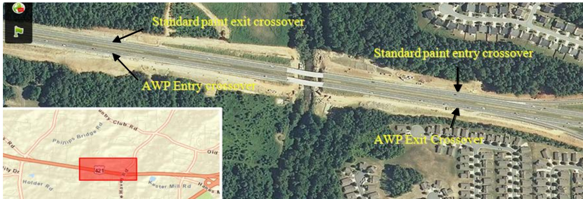
Figure 13. Photo. US-421 crossover locations.
