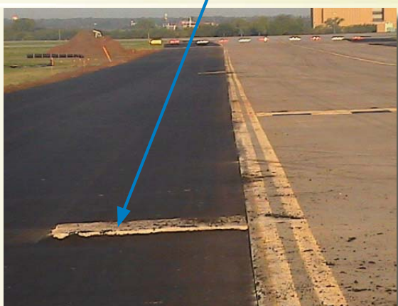
Concrete manhole covers
