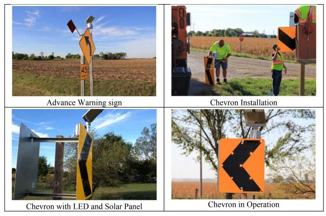
Figure 13. Photos. Installation of the SDCWS. (Source: ISU/TTI)
