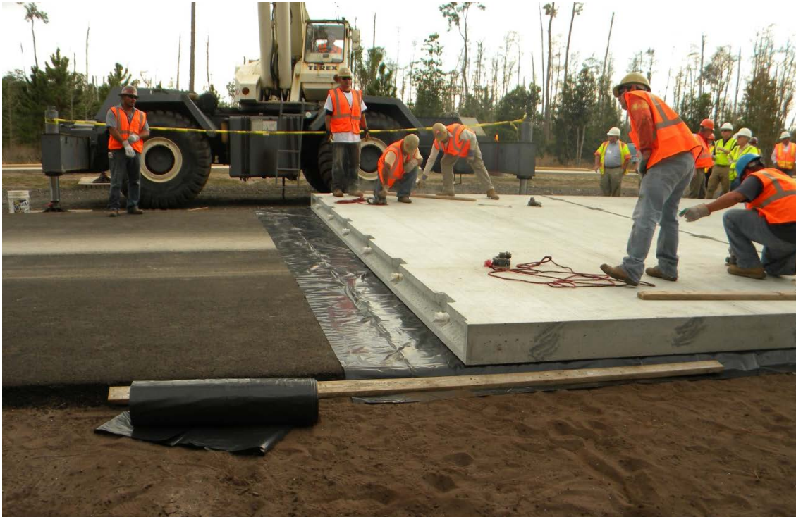
Figure 4. Photo. Panel placement.
