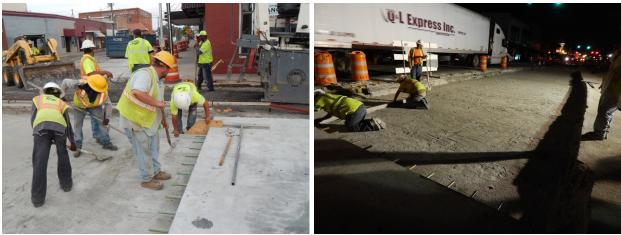
Figure 35. Photos. Hand manipulation of the bedding material at a joint location.
