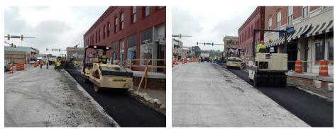
Figure 39. Photos. Parking lane construction using asphalt concrete.
