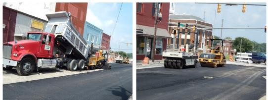
Figure 40. Photos. Resurfacing of an intersecting street.
