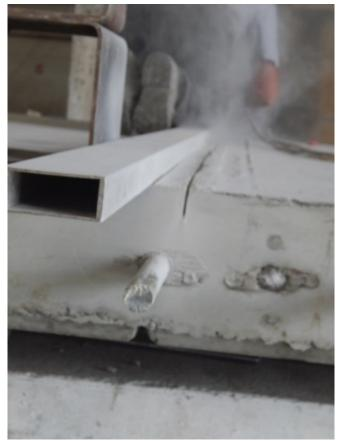
Figure 27. Photo. Longitudinal sawcut in a two-lane wide panel (also showing dowel bar located at the sawed centerline).
