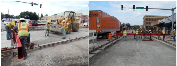
Figure 34. Photos. Bedding material placement and compaction.
