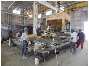
Figure 25. Photo. Concrete placement and consolidation.
