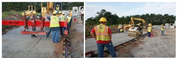
Figure 15. Photos. Base grading and compaction.
