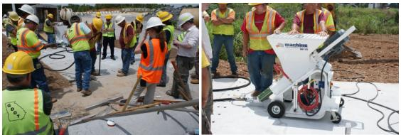
Figure 18. Photos. Slot grouting and grout pump.
