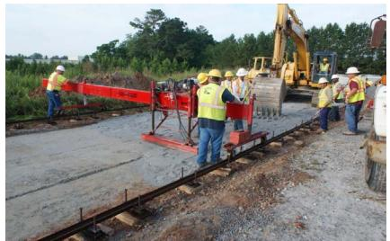
Figure 16. Photo. Bedding layer grading.
