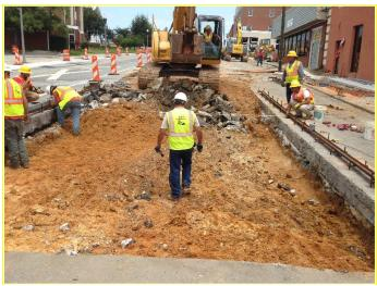
Figure 30. Photo. Existing composite pavement removal.
