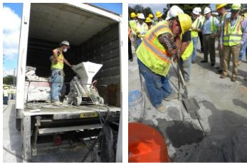
Figure 38. Photo. Dowel slot grouting operation.
