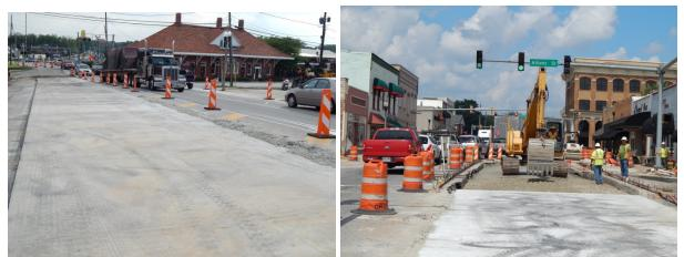
Figure 14. Photos. Lane closure and two-way traffic operation.
