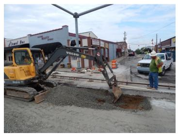
Figure 31. Photo. Removing the softer subgrade material.
