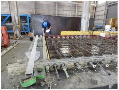
Figure 22. Photo. Formwork being checked for tolerances.
