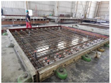
Figure 19. Photo. Panel formwork ready for concrete placement.
