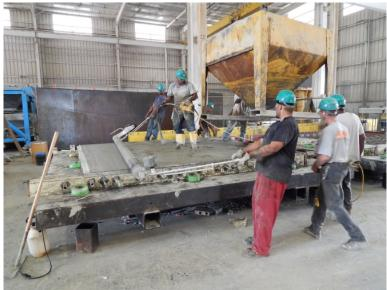
Figure 26. Photo. Concrete surface finishing using a roller screed.
