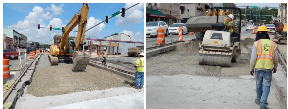
Figure 32. Photos. Base material placement and compaction.
