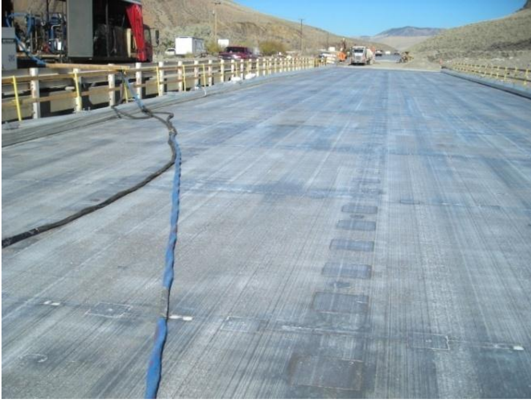
Figure 16. Photo. Finished milled deck.
