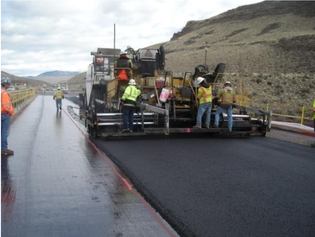
Figure 17. Photo. Paving on deck.
