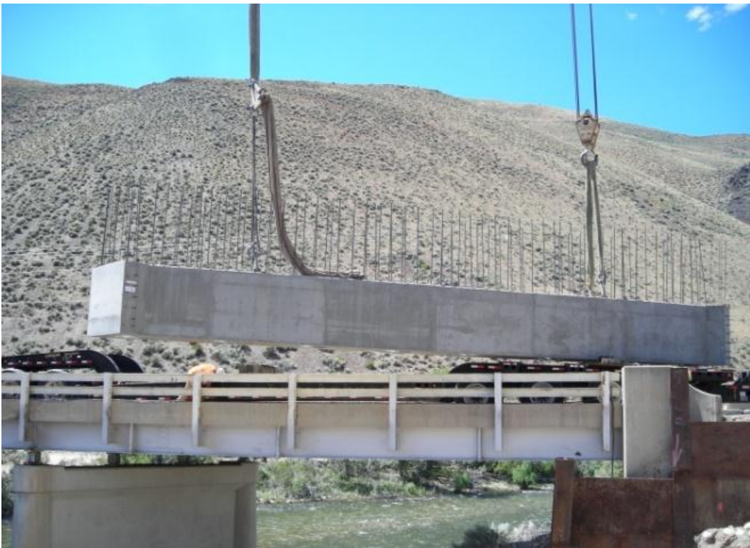
Figure 5. Photo. Precast abutment.
