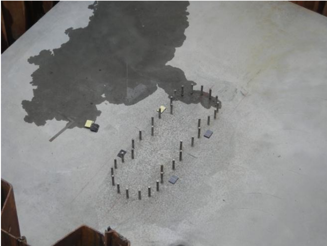
Figure 7. Photo. Pier footing rebar.
