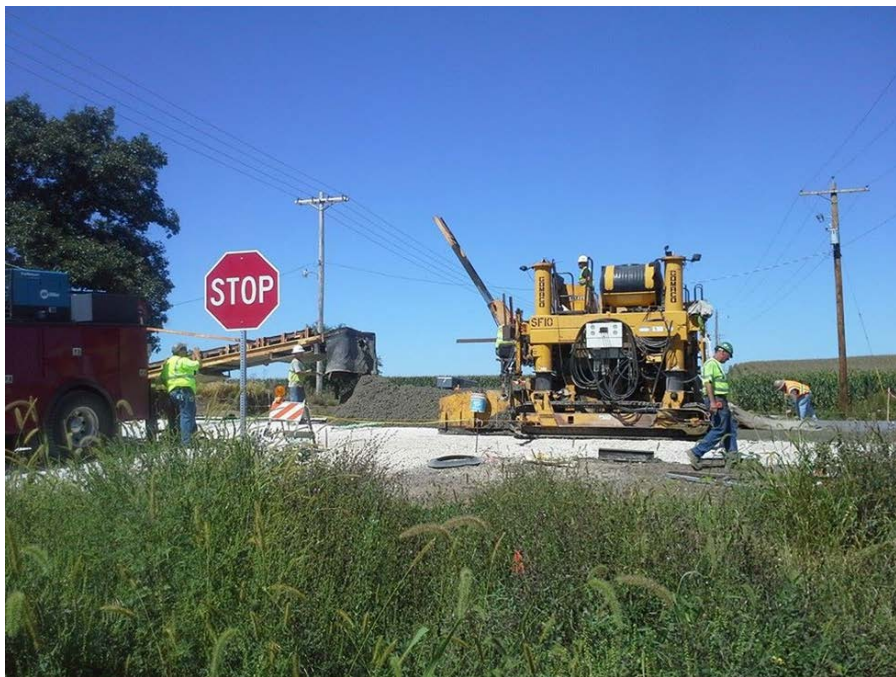
Figure 11. Photo. Placement of concrete at 1600E intersection. (courtesy: Knox County Highway Department)
