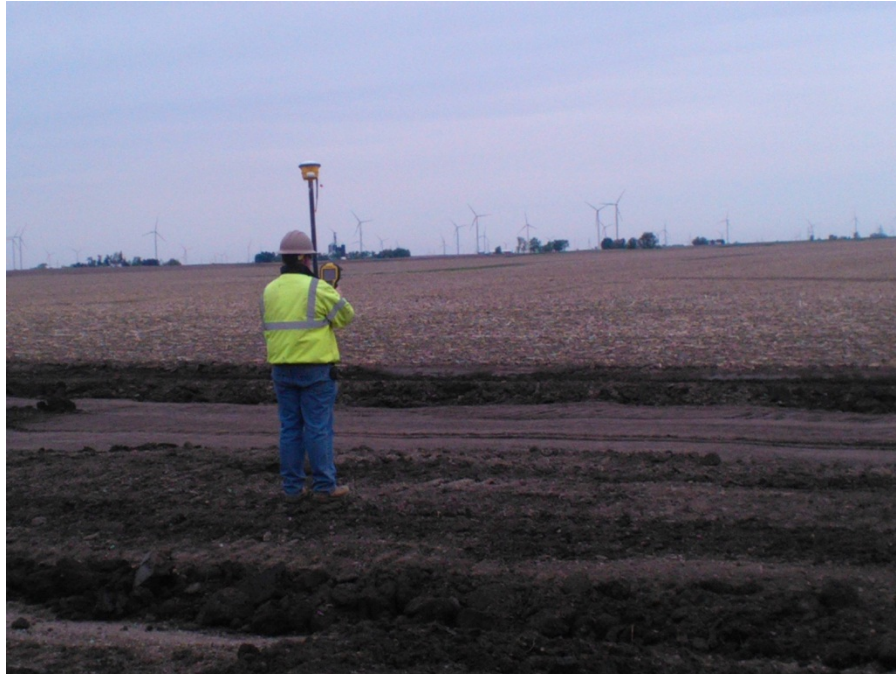
Figure 3. Photo. An operator using the GPS survey rover.
