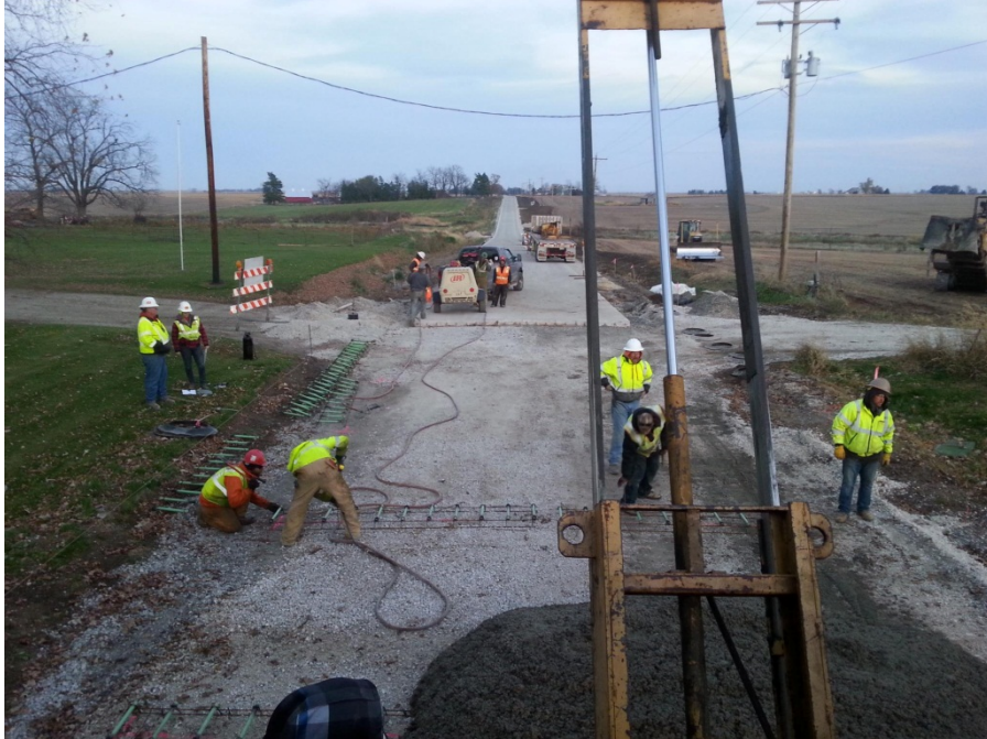
Figure 10. Photo. Aggregate base and dirt fill being carried out. (courtesy: Knox County Highway Department)
