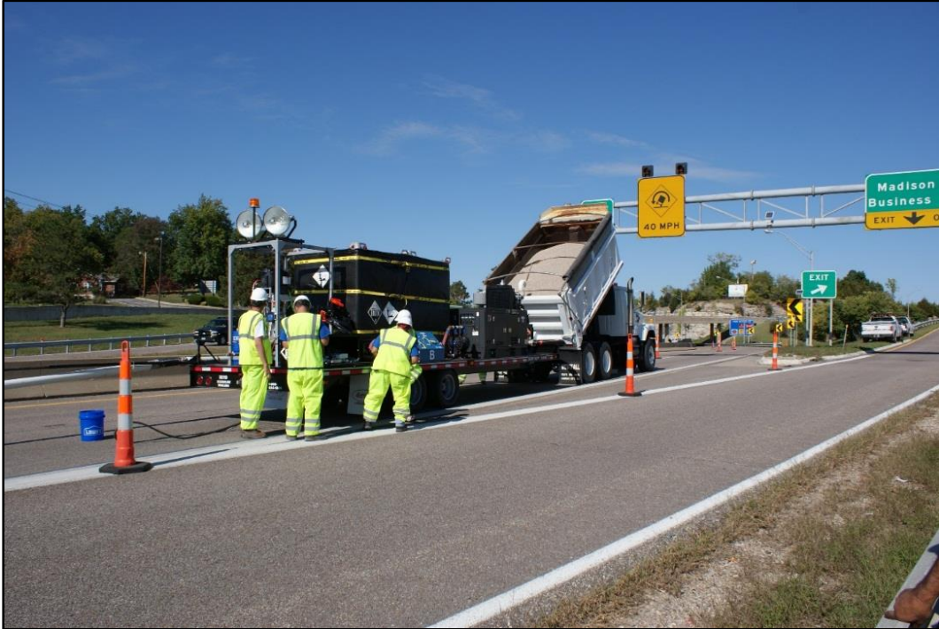
Figure 8. Photo. Dump truck supplying surface to distribution trailer.
