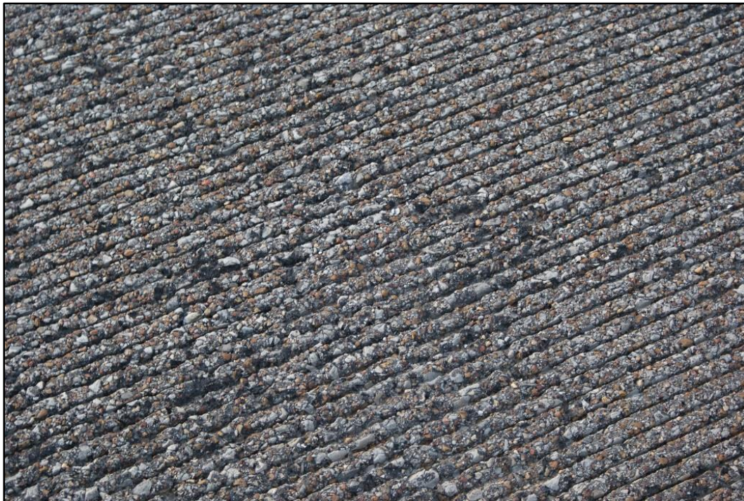
Figure 16. Photo. Grooved pavement surface prior to application (near MO J).
