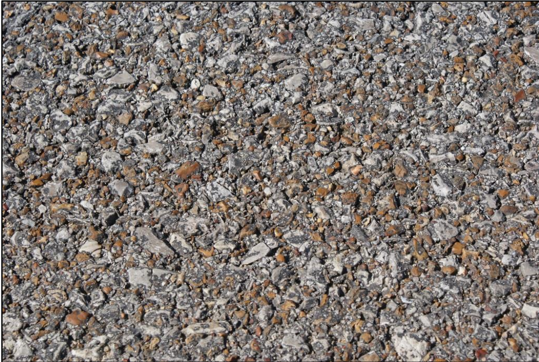
Figure 4. Photo. Surface prior to application.
