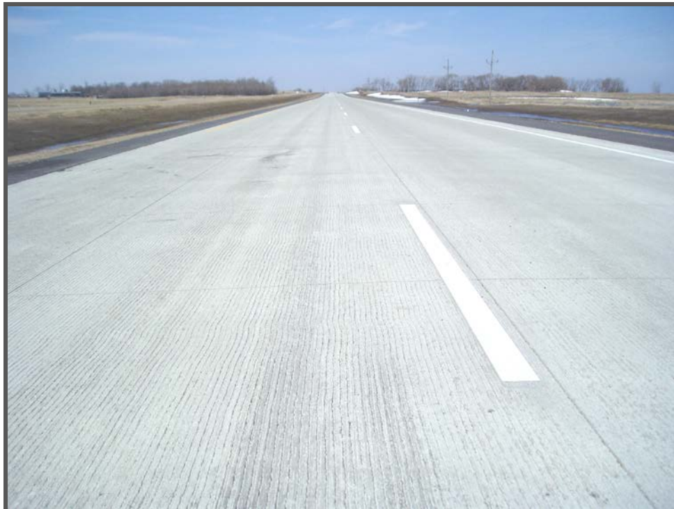
Figure 8. Closeup of the completed whitetopping showing the longitudinally tined surface texture and sawcut joints.
