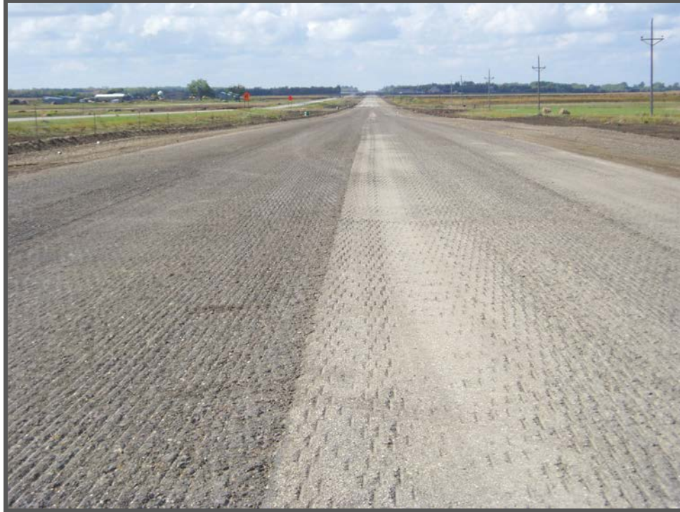
Figure 4. Rough-milled surface of the original HMA pavement.
