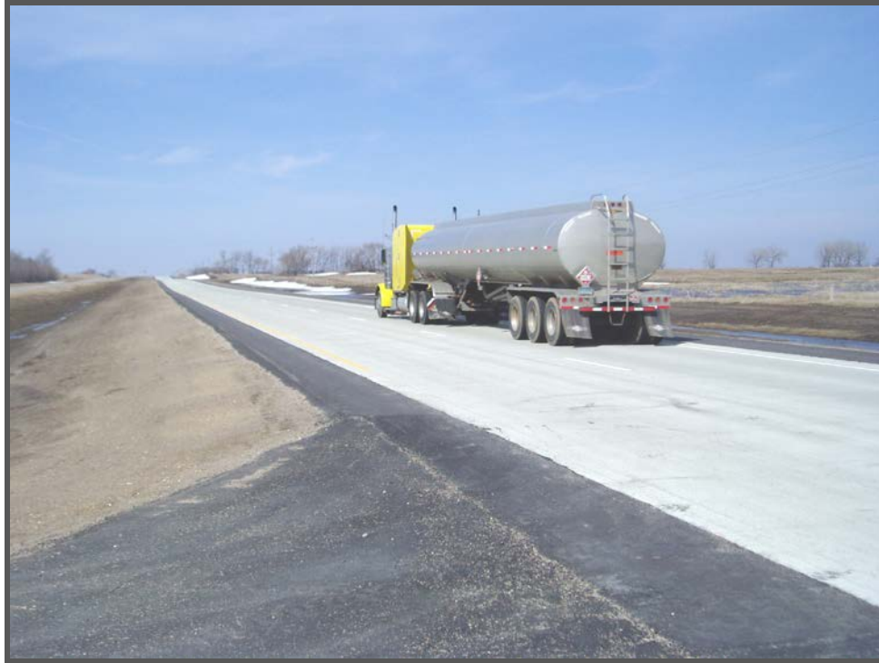
Figure 7. Completed whitetopped pavement.
