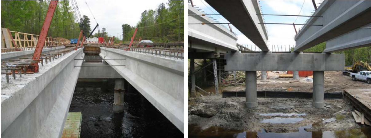
Figure 12. Construction of Black River Bridge (Phase I).
