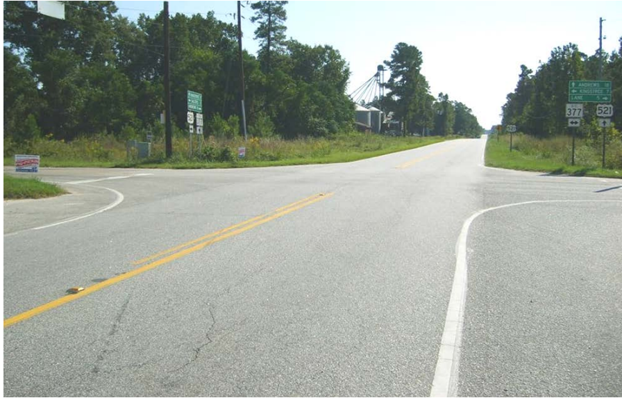
Figure 6. Intersection of U.S. 521 and SC 377 before reconstruction.
