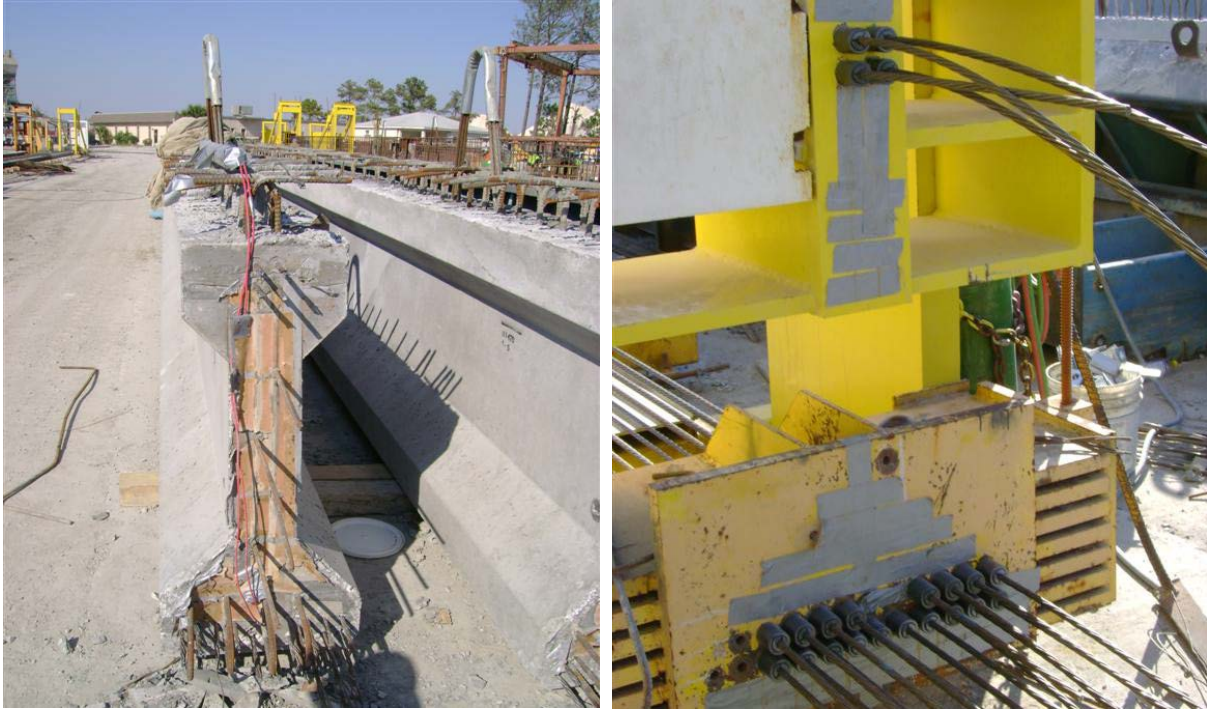
Figure 10. SCC beam pretension tendon detail.
