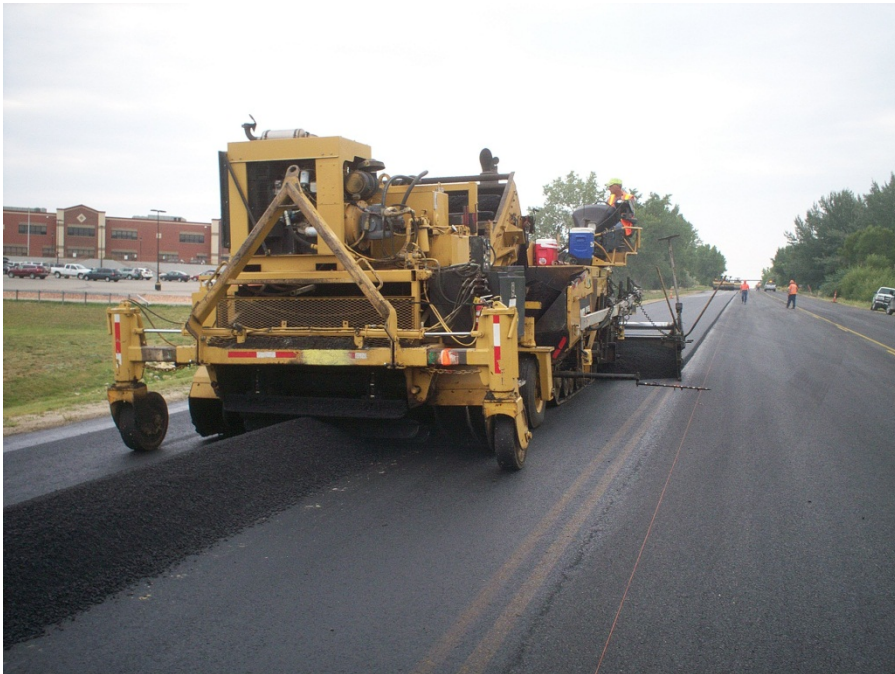
Figure 25. Photo. WMA paving. (courtesy: Wyoming DOT)
