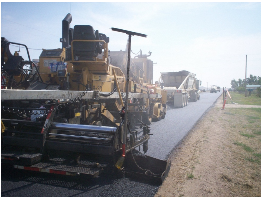
Figure 13. Photo. 6:1 taper for an unpaved shoulder. (courtesy: Wyoming DOT)
