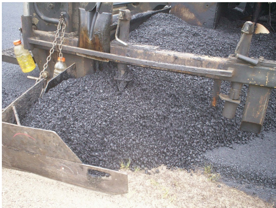
Figure 11. Photo. Fabricated shoe attached to the paver. (courtesy: Wyoming DOT)
