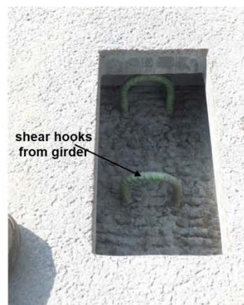
d) Shear pocket ( panel-to-girder connection)
