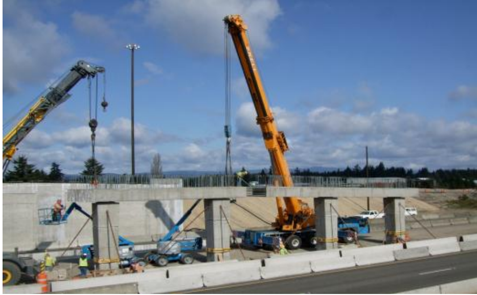
Figure 47. Photo. Precast cap beam placement.
