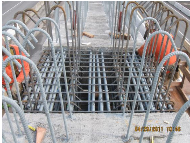
Figure 54. Photo. Lower-stage cap beam closure prior to concrete placement.
