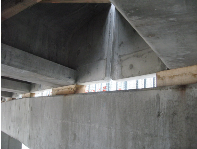
Figure 55. Photo. Girder end wall diaphragms and girders on oak blocks.
