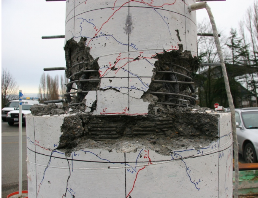
Figure 38. Photo. Specimen DS-1 after testing.
