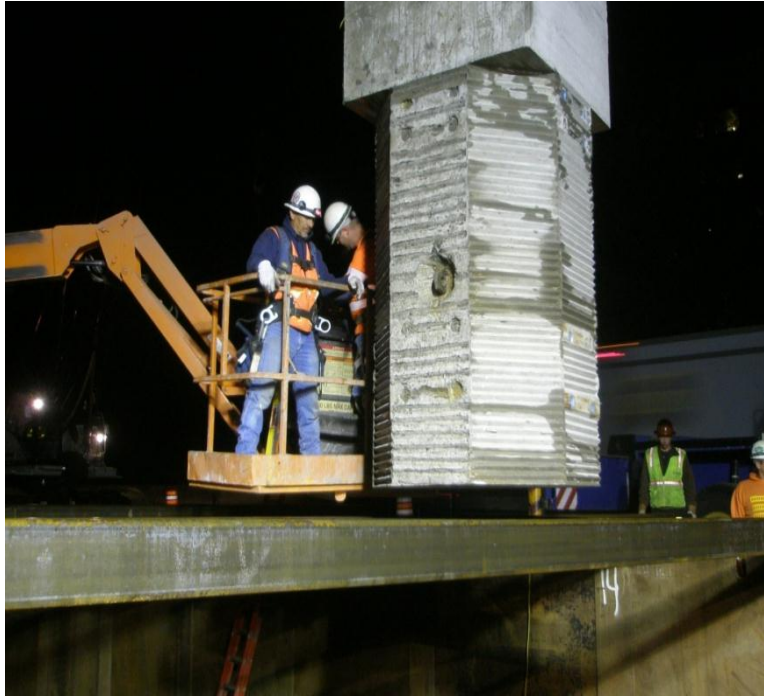
Figure 5. Photo. Socket connection concept, as originally used.
