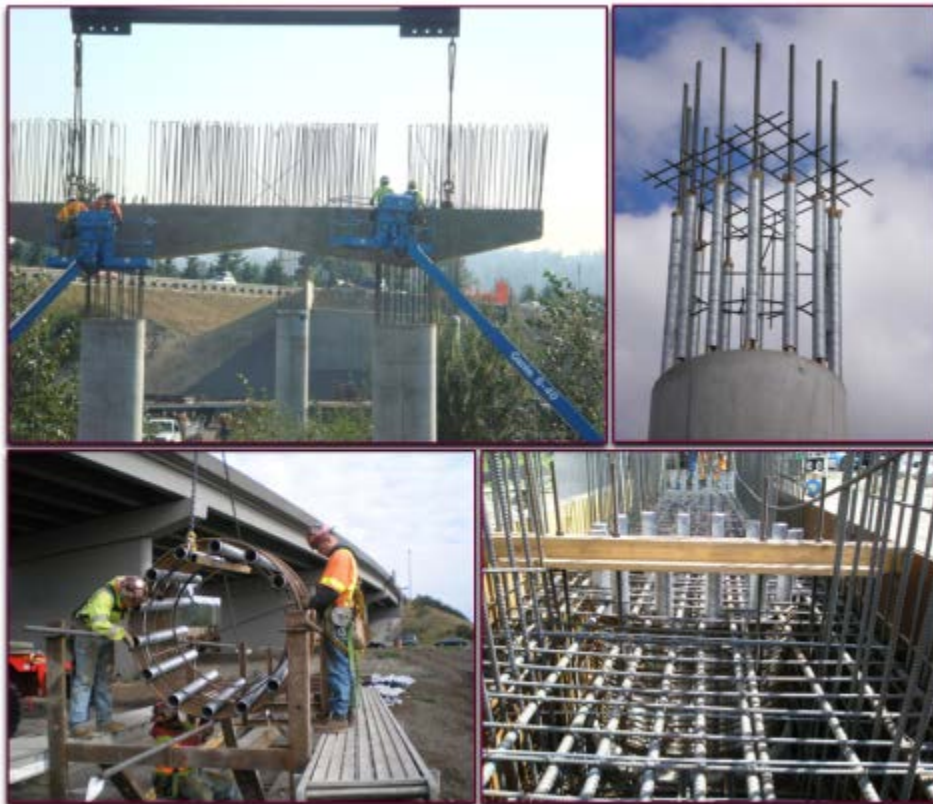
Figure 6. Photos. Precast bent cap under construction in Washington State.
