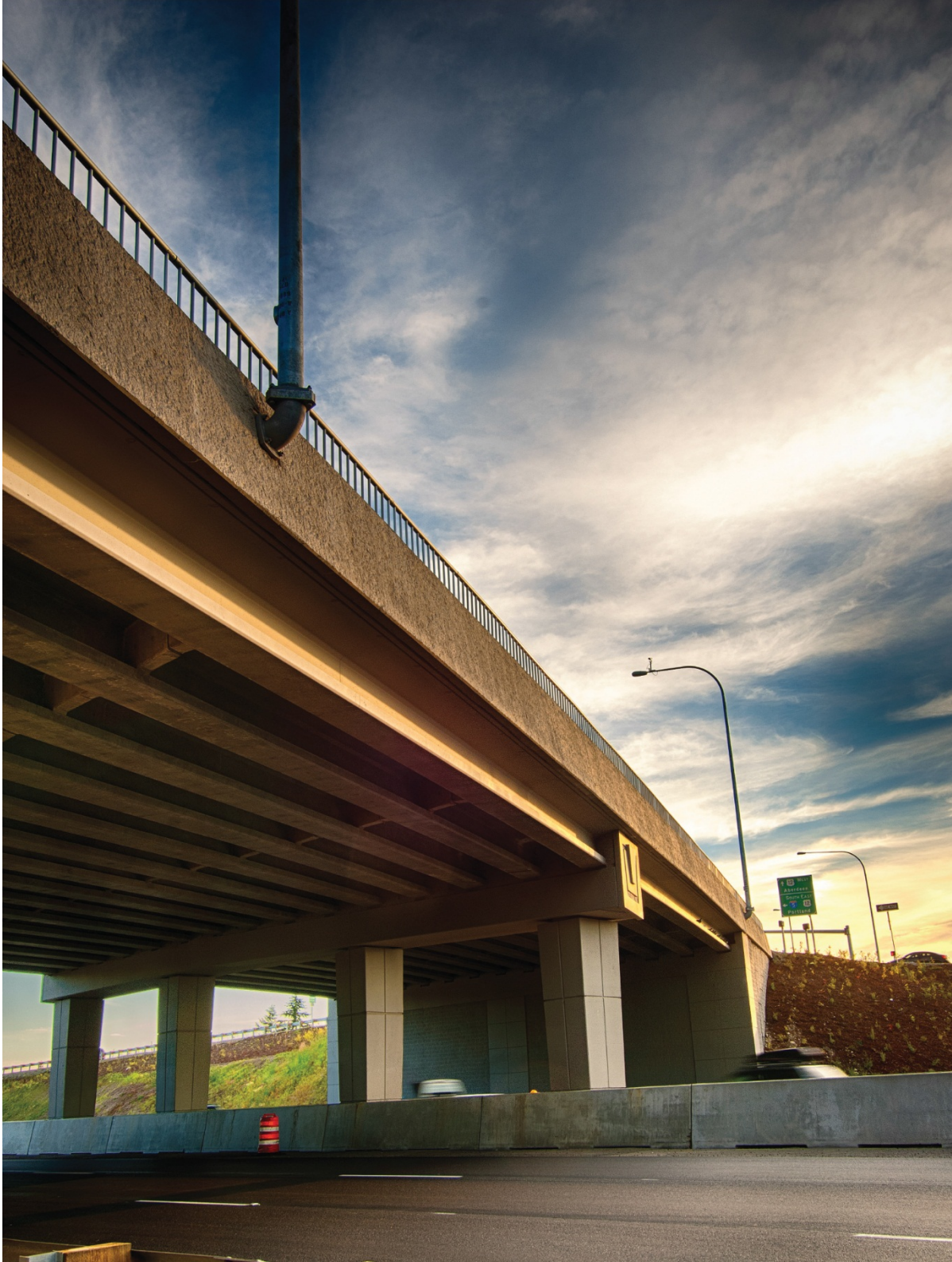
Figure 50. Photo. Completed demonstration bridge (photo courtesy of the Precast/Prestressed Concrete Institute).
