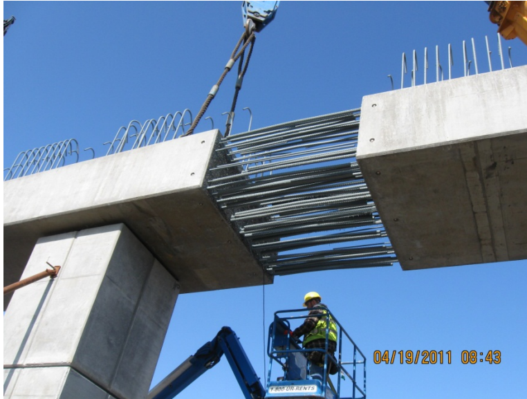
Figure 53. Photo. Lowering the second lower-stage cap beam into place.
