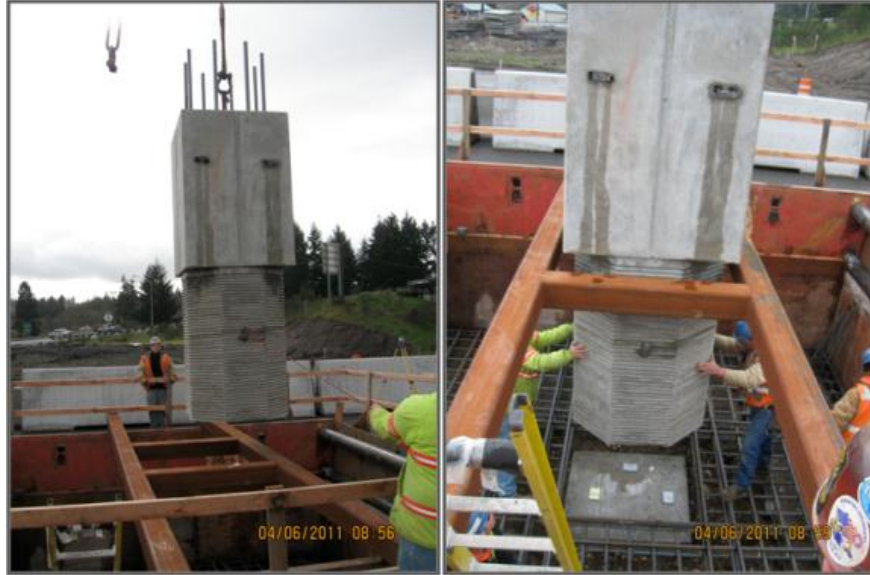
Figure 45. Photos. Construction sequence for placement of first precast column segment.
