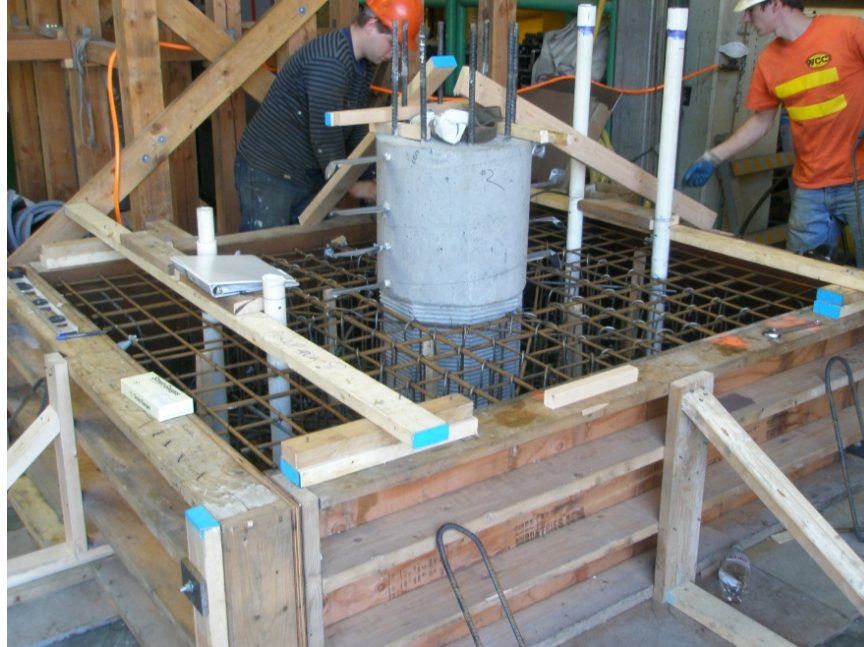
Figure 15. Photo. Construction of spread footing test specimen.
