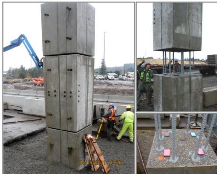
Figure 46. Photos. Construction sequence for placement of the column segments.
