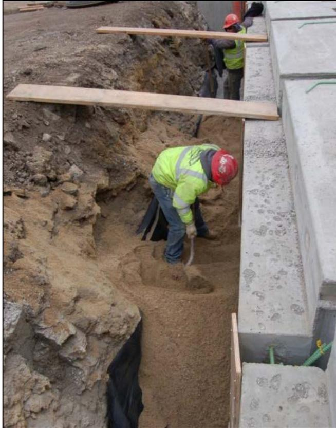
Figure 15. Workers spread granular backfill behind an abutment.
