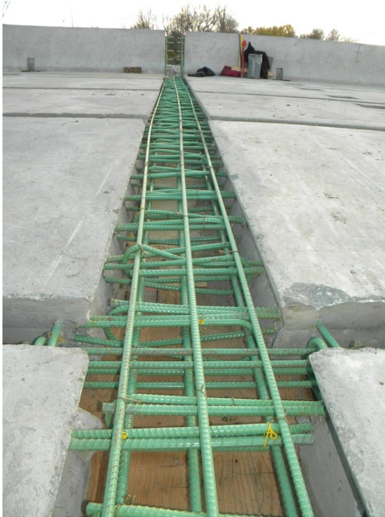
Figure 18. Pier joint reinforcement.
