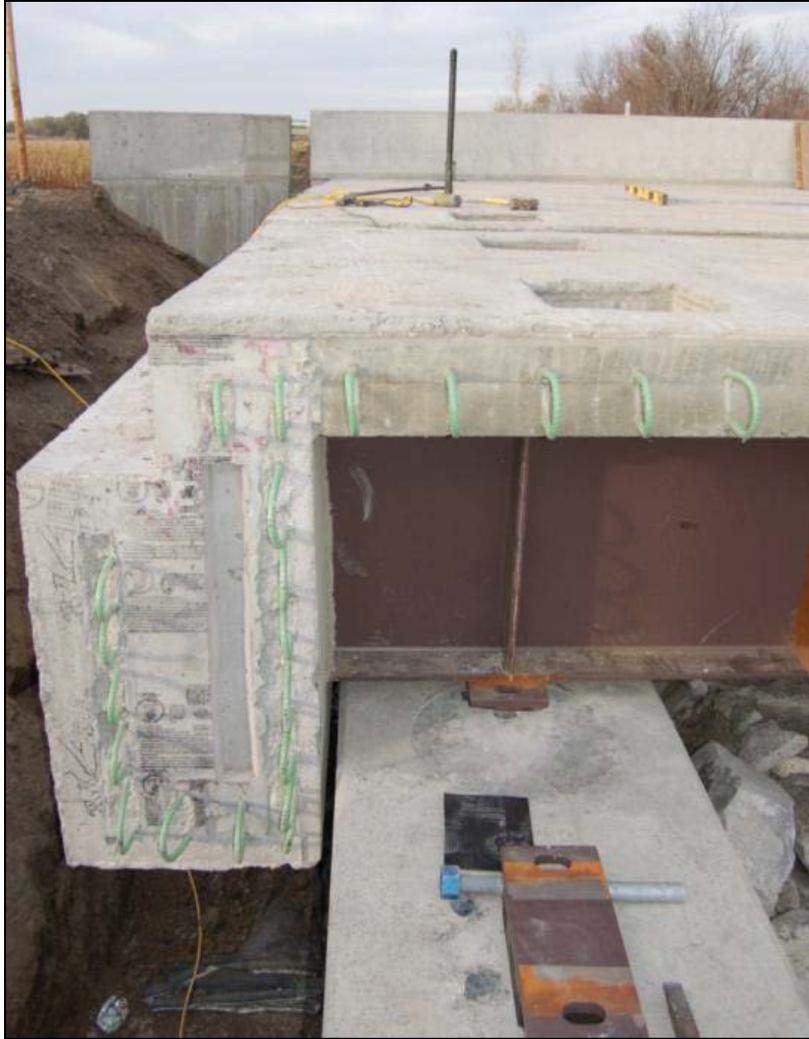
Figure 14. Suspended backwall of an interior module (source: HNTB Corp.).
