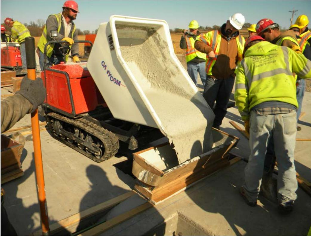
Figure 19. Workers place UHPC in a longitudinal joint.
