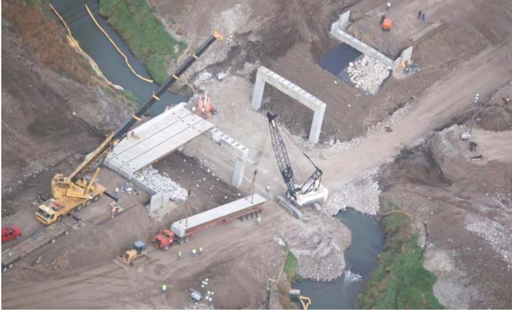
Figure 9. Aerial view showing placement of bridge modules.
