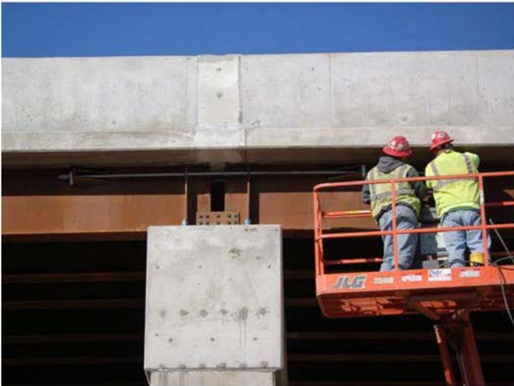
Figure 21. Post-tension retrofit installation.
