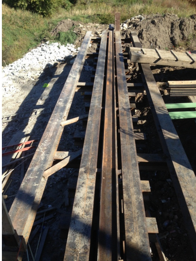
Figure 14. Photo. Slide channel on falsework (courtesy: Iowa DOT).
