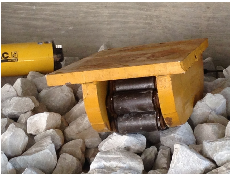
Figure 30. Photo. Removed rollers (courtesy: Iowa DOT).
