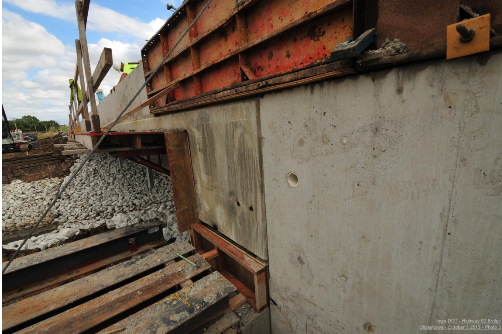
Figure 33. Photo. Bridge diaphragm and wing.
