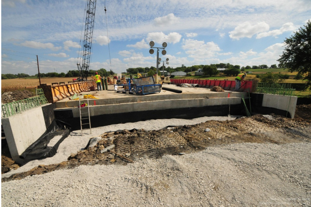
Figure 35. Photo. Abutment backfill (courtesy: Iowa DOT).
