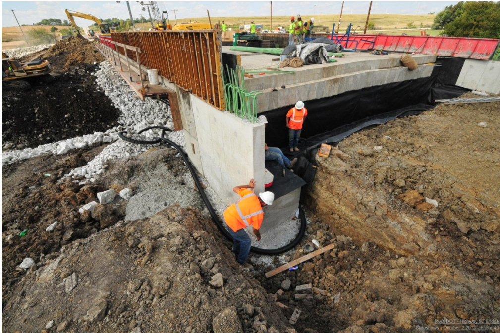
Figure 34. Photo. Subdrain (courtesy: Iowa DOT).
