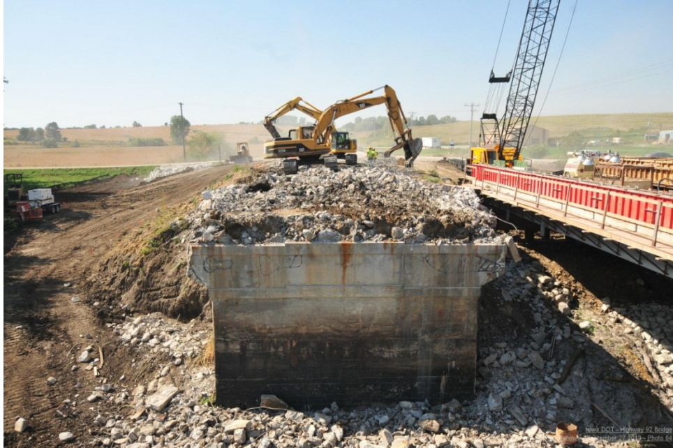
Figure 15. Photo. Bridge being demolished (courtesy: Iowa DOT).
