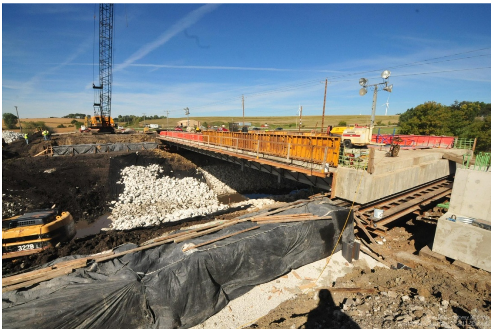
Figure 18. Photo. Abutment footing (courtesy: Iowa DOT).
