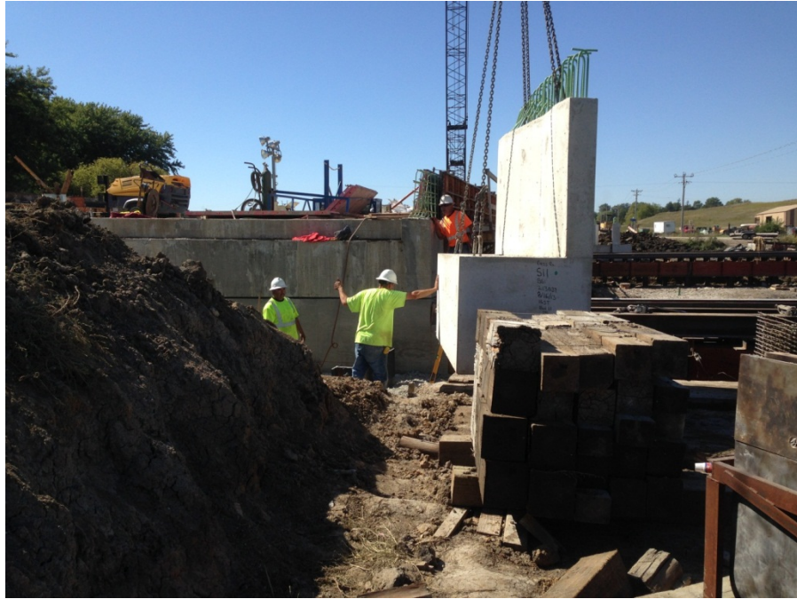
Figure 31. Photo. Precast wingwalls (courtesy: Iowa DOT).
