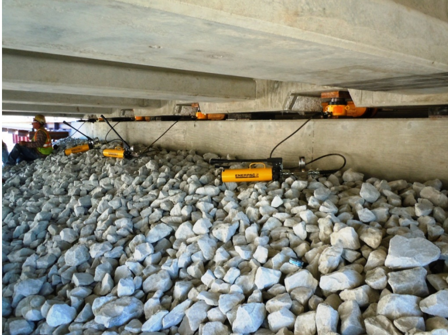
Figure 29. Photo. Bridge jacking (courtesy: Iowa DOT).
