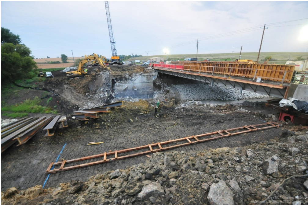
Figure 16. Photo. H-pile template (courtesy: Iowa DOT).
