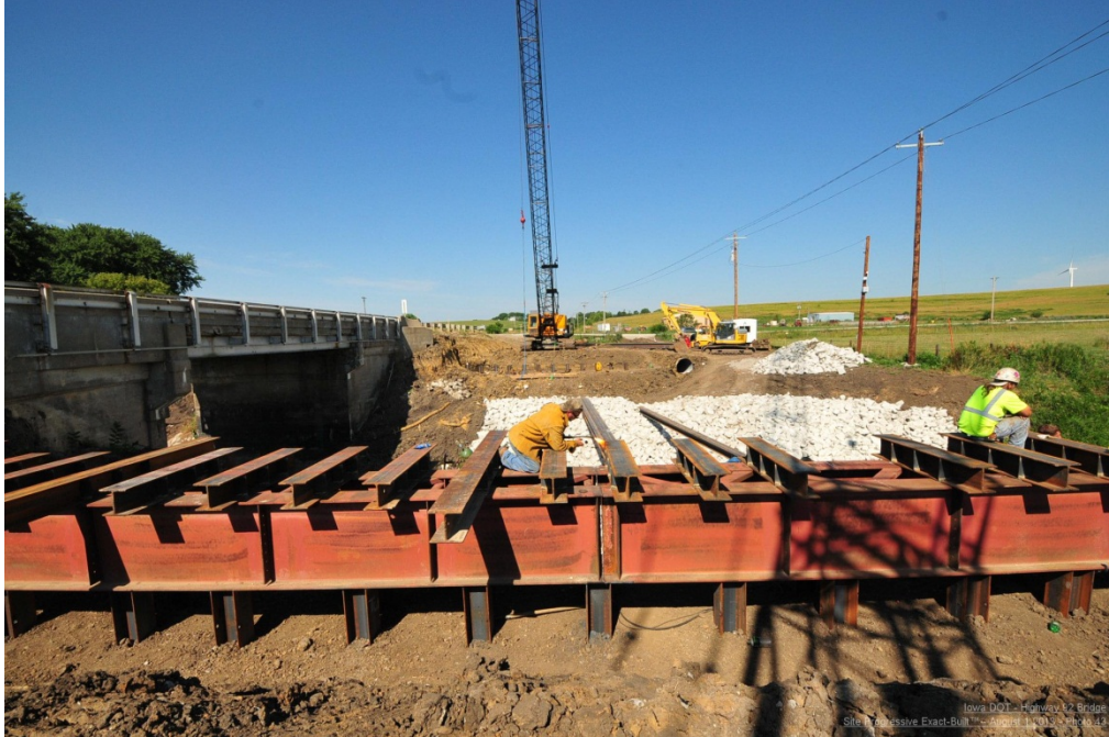
Figure 11. Photo. Falsework (courtesy: Iowa DOT).
