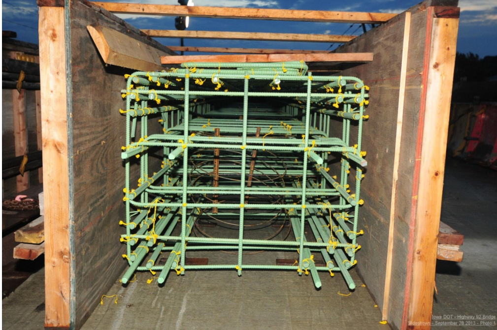
Figure 19. Photo. Pre-tied cage (courtesy: Iowa DOT).
