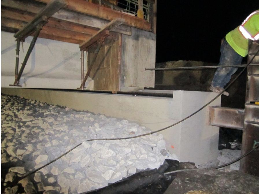
Figure 27. Photo. Slide near completion (courtesy: Iowa DOT).
