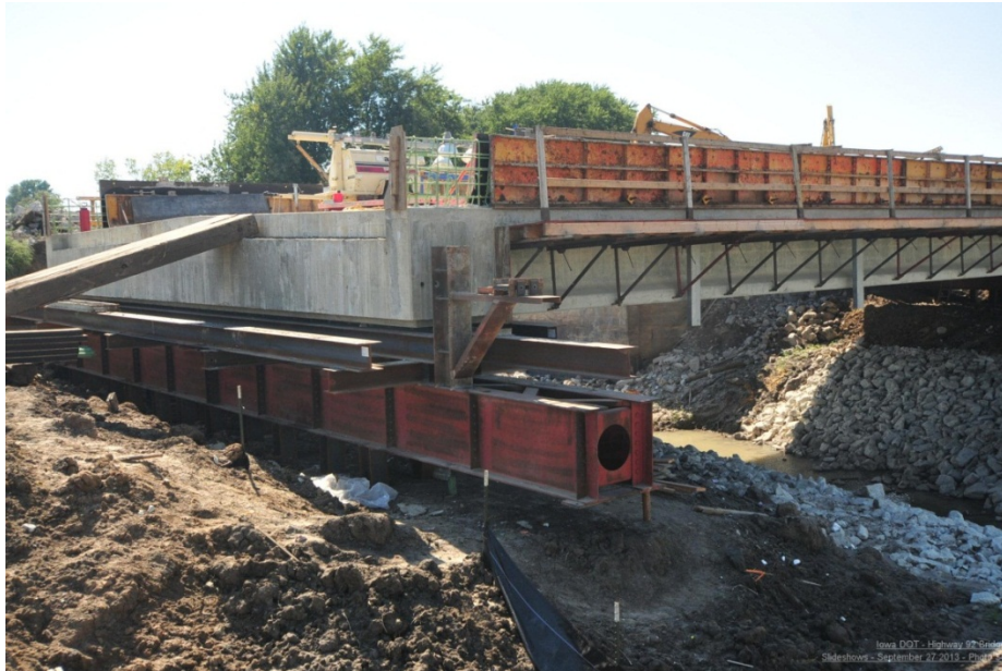
Figure 13. Photo. Completed superstructure (courtesy: Iowa DOT).
