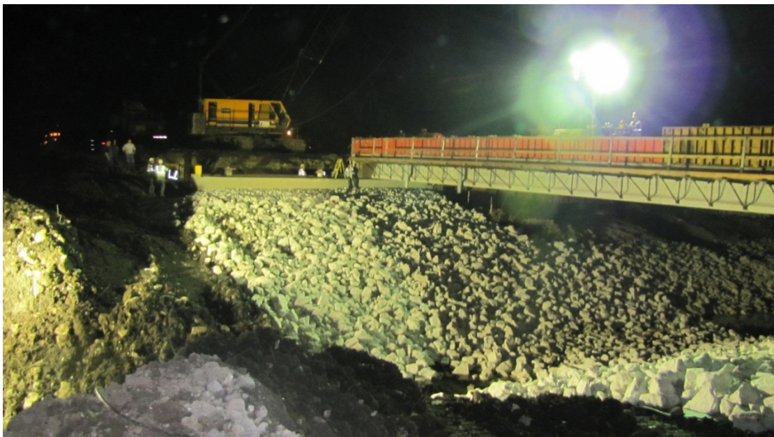
Figure 26. Photo. Bridge slide (courtesy: Iowa DOT).
