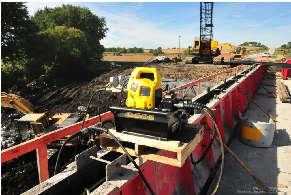
Figure 22. Photo. Slide jack control (courtesy: Iowa DOT).
