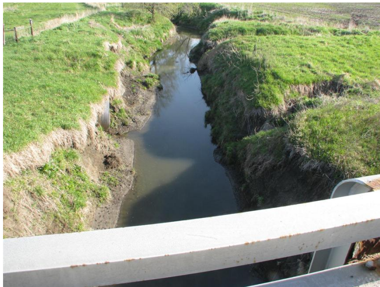
Figure 10. Photo. Project staging area (courtesy: Iowa DOT).
