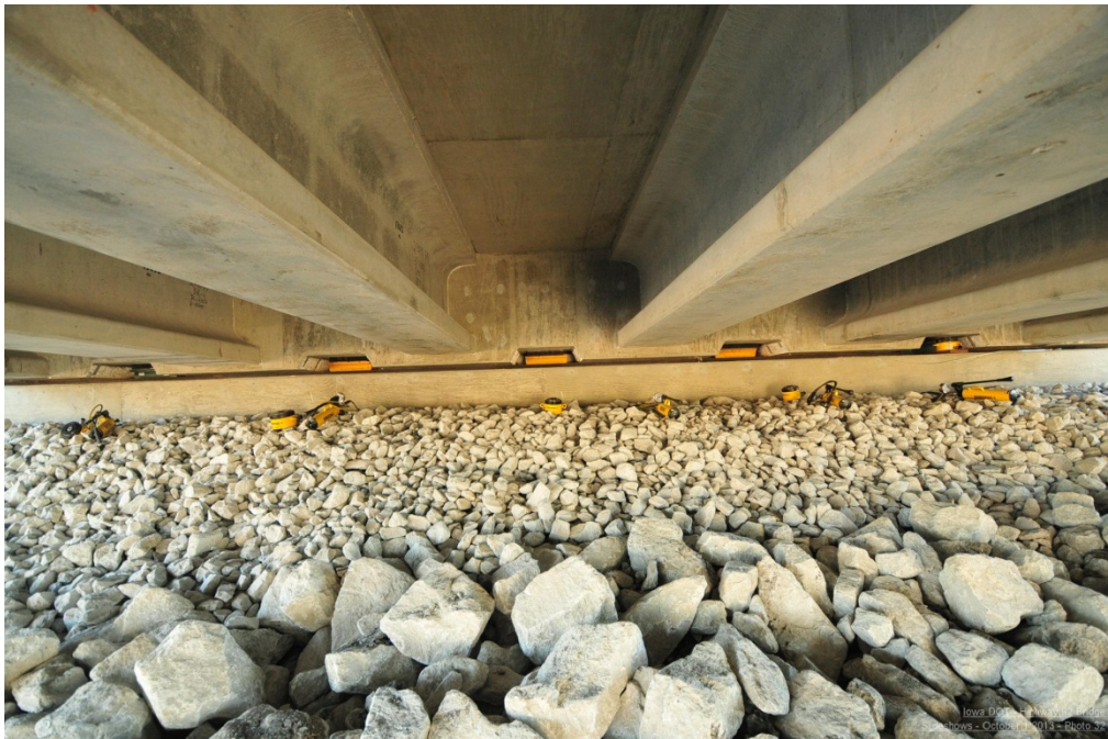
Figure 28. Photo. Roller removal (courtesy: Iowa DOT).
