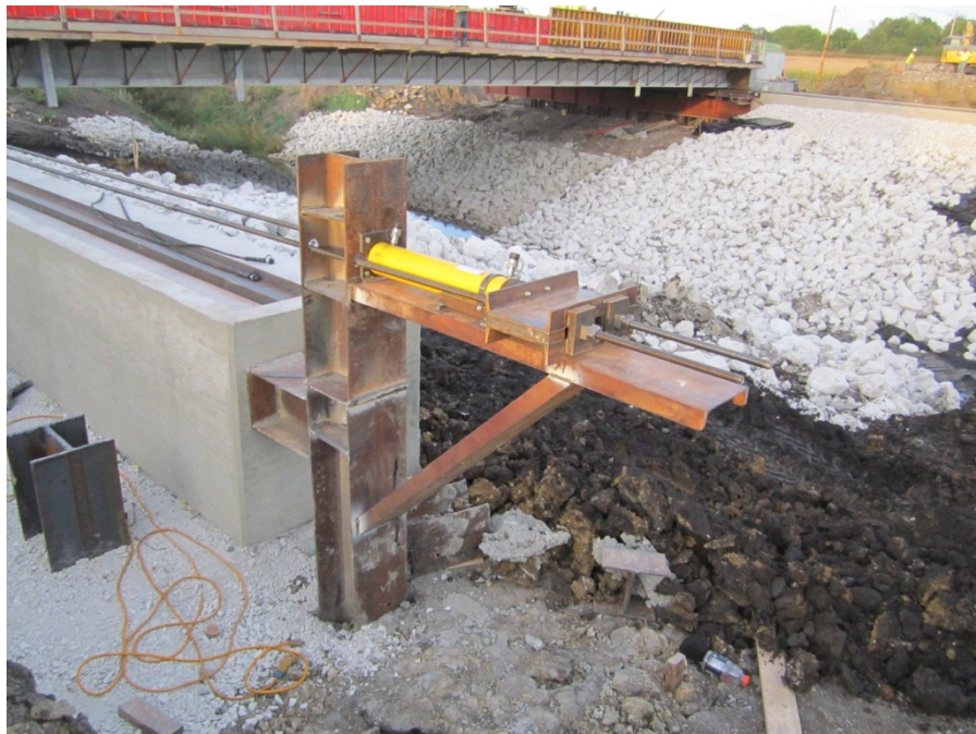
Figure 23. Photo. Jacking frame (courtesy: Iowa DOT).
