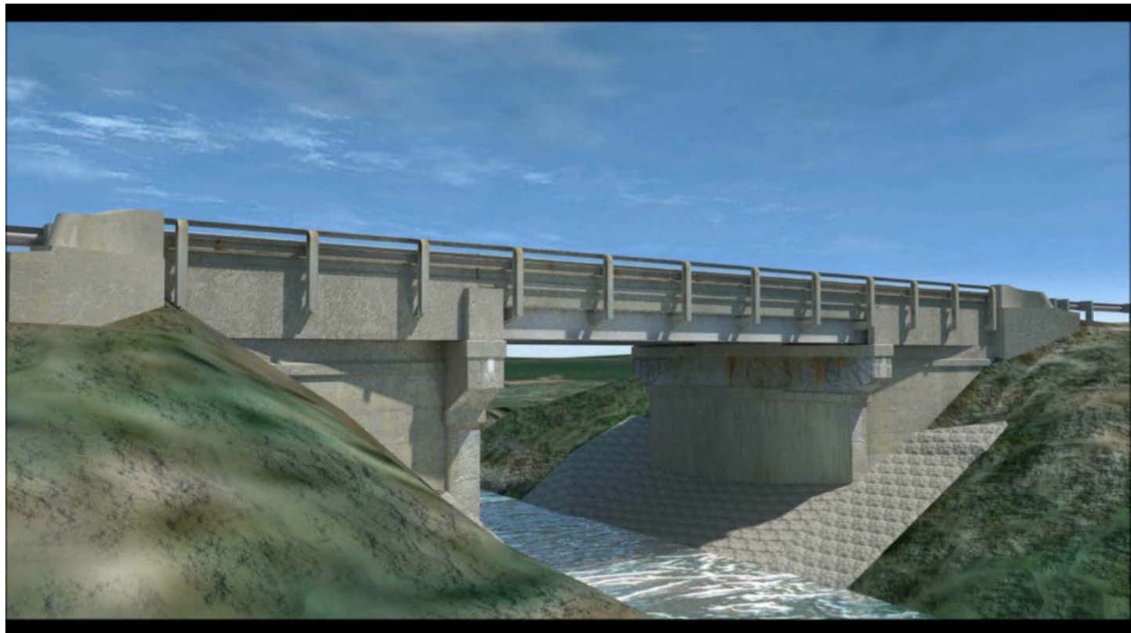
Figure 5. Illustration. Bridge construction visualization (source: Iowa DOT website).
