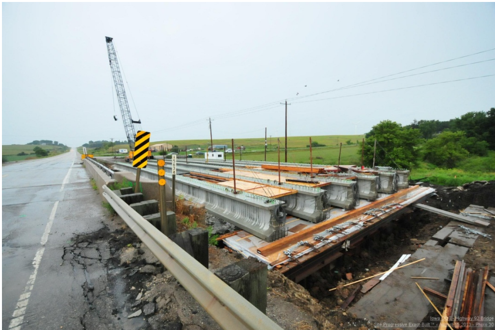
Figure 12. Photo. Concrete beams and decking (courtesy: Iowa DOT).
