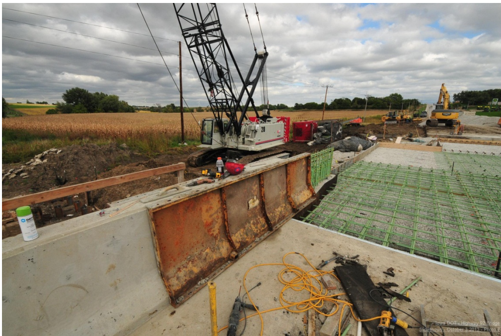
Figure 36. Photo. Approach and barrier (courtesy: Iowa DOT).
