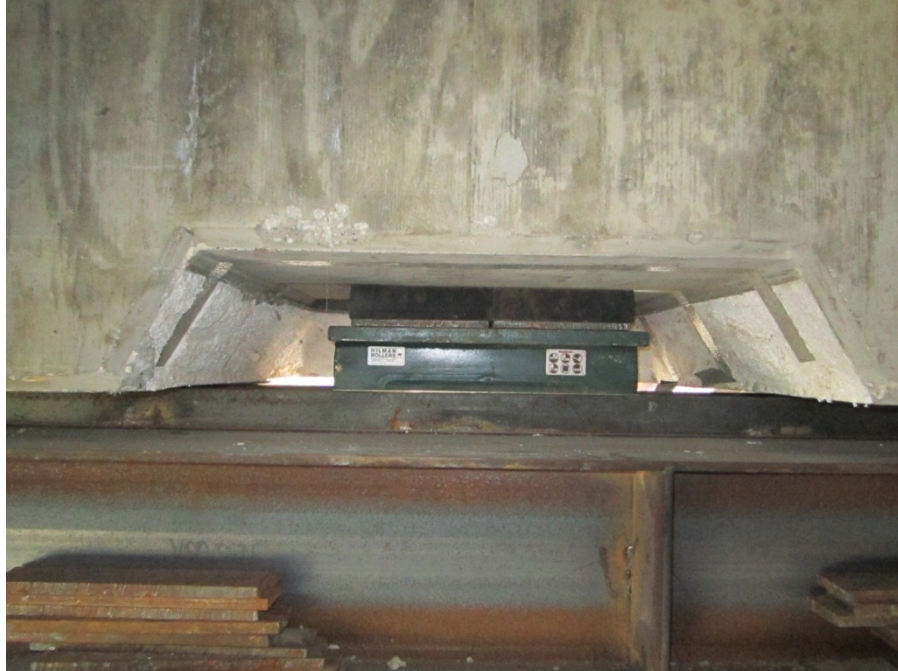
Figure 21. Photo. Sliding pad and roller system (courtesy: Iowa DOT).
