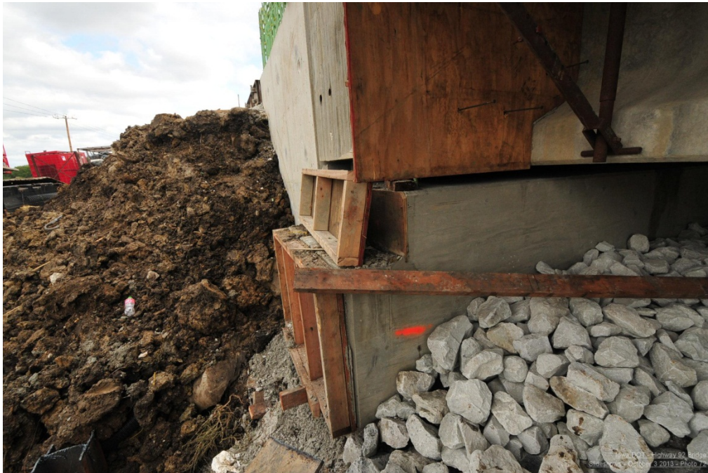
Figure 32. Photo. Falsework seat (courtesy: Iowa DOT).
