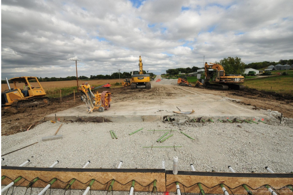
Figure 37. Photo. Approach connection (courtesy: Iowa DOT).
