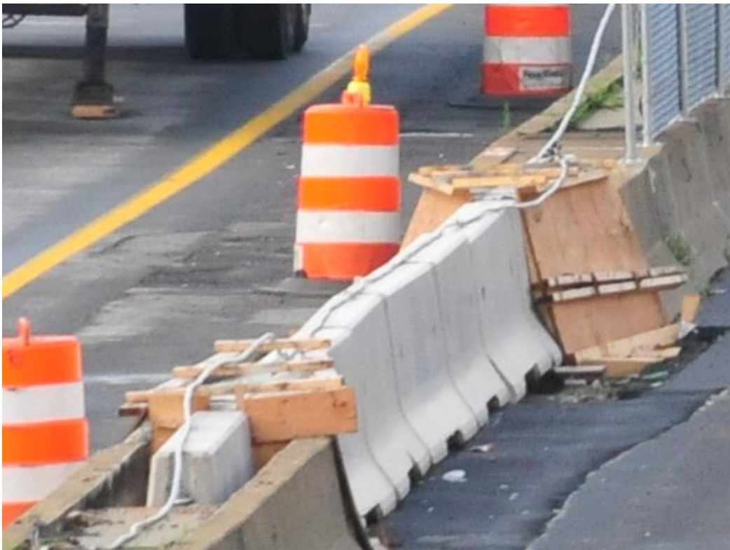
Figure 28. Photo. Movable barriers at emergency access points.
