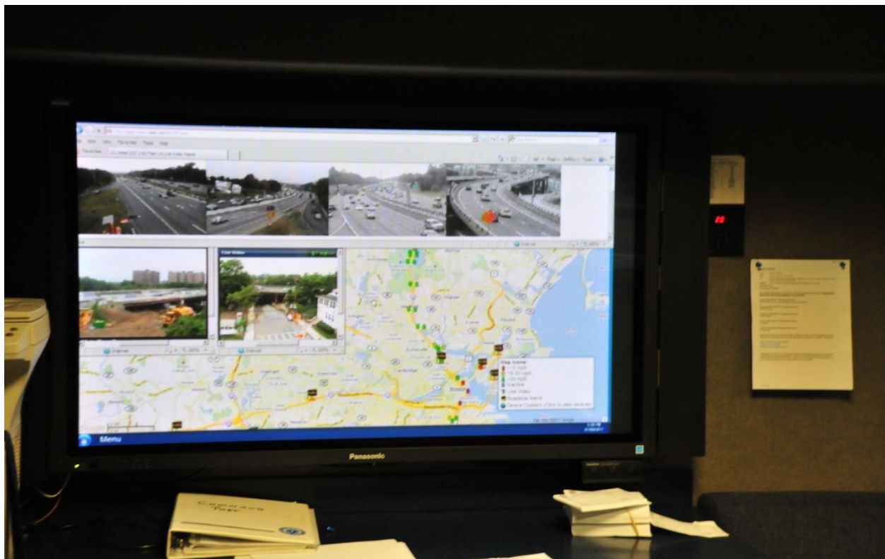
Figure 34. Photo. Video wall at command post.
