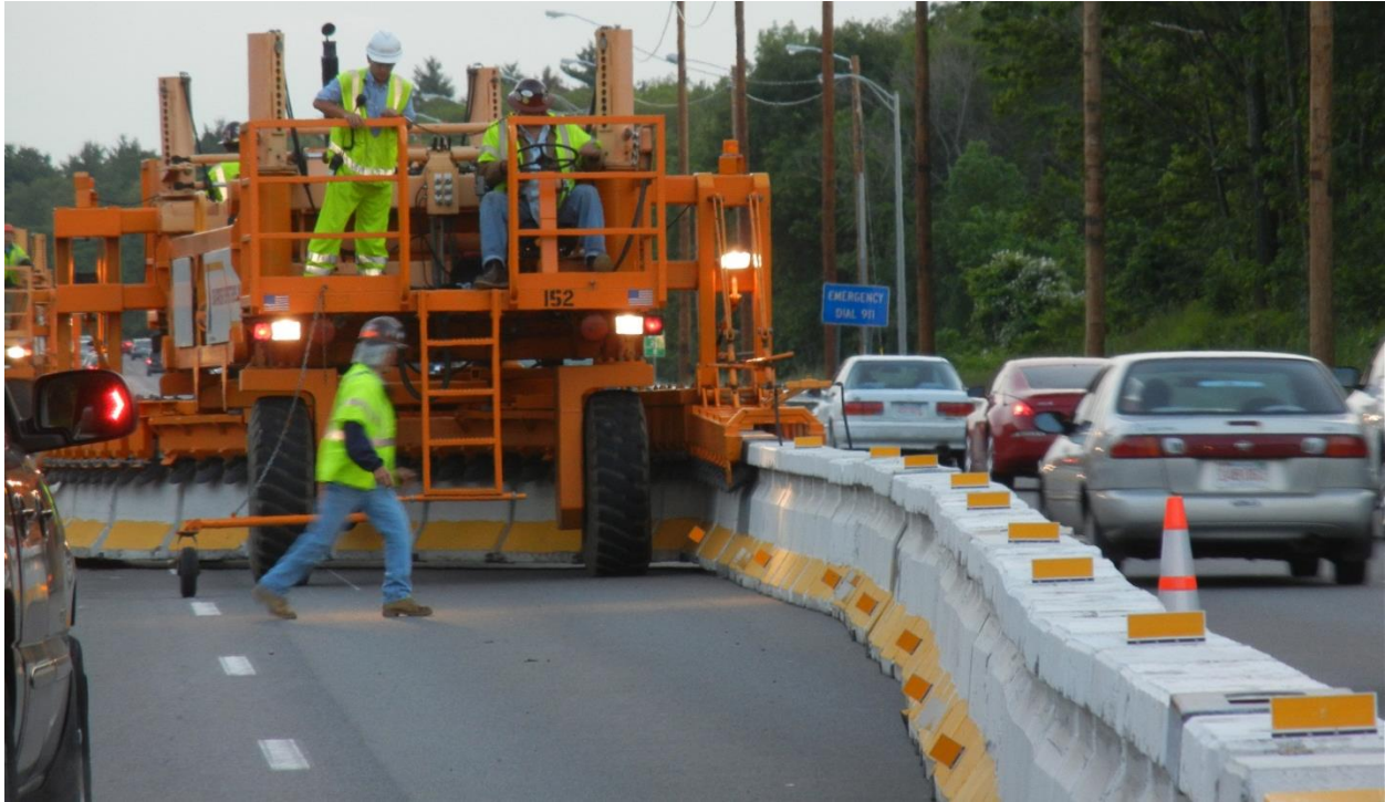
Figure 25. Photo. Installation of movable barriers.
