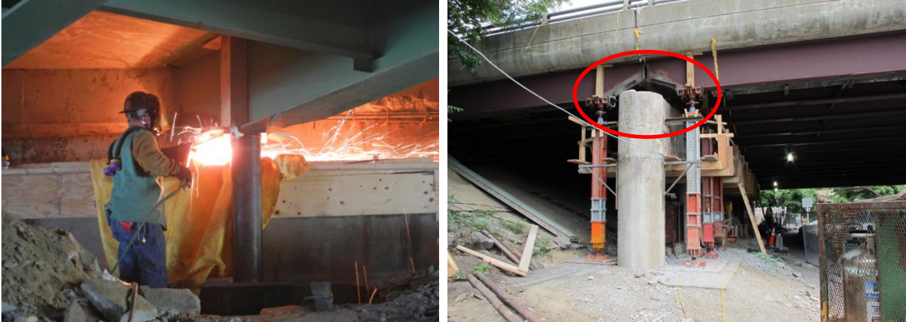
Figure 16. Photo. Shoring and coping of beam ends.
