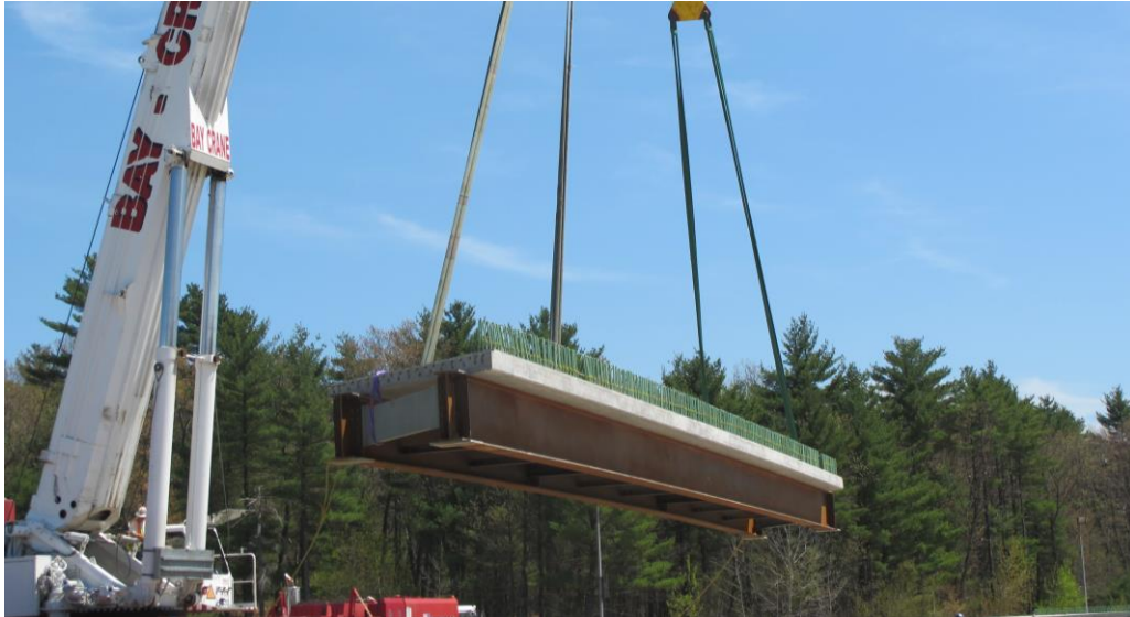
Figure 4. Photo. Modular beam/deck system.
