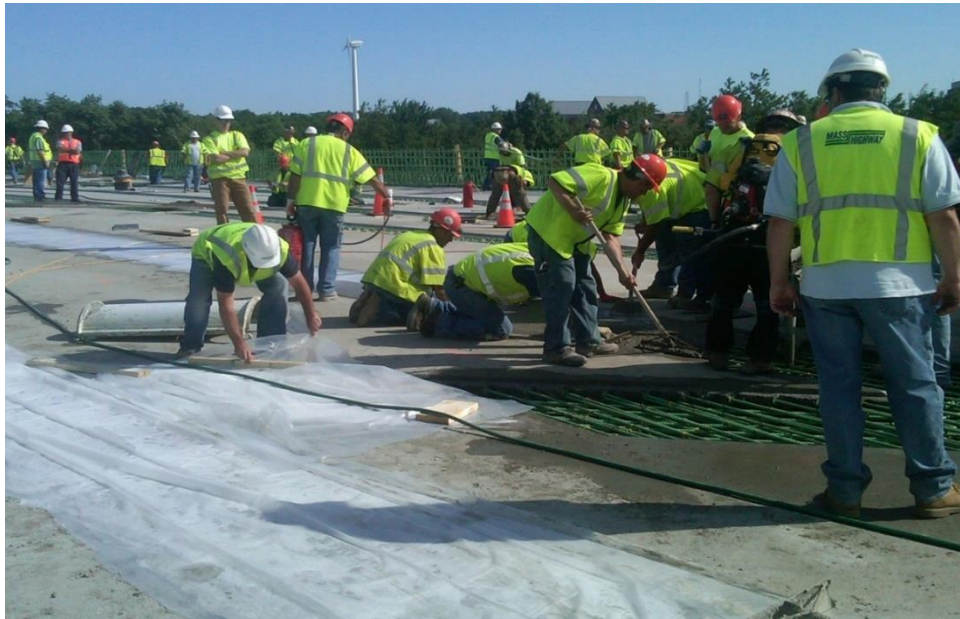
Figure 41. Photo. MassDOT personnel conducting inspection during bridge deck closure pour.
