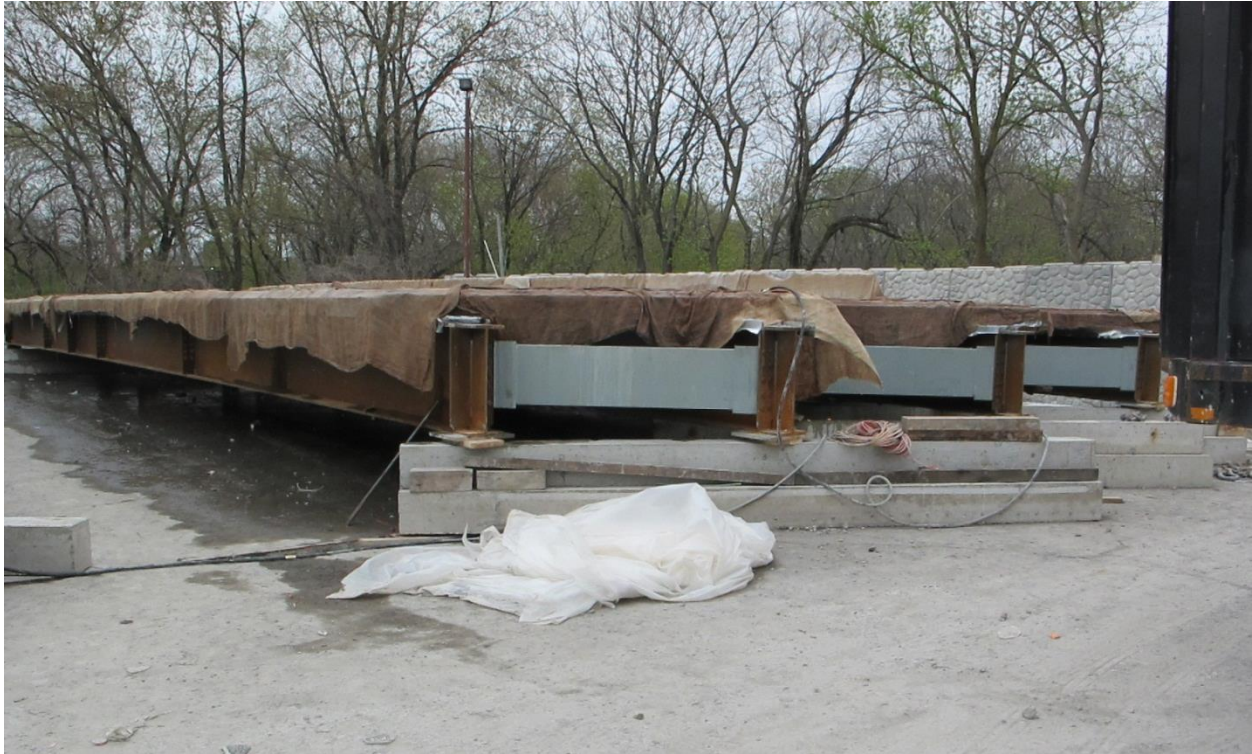
Figure 13. Photo. Water curing of PMSE units at the precast facility.
