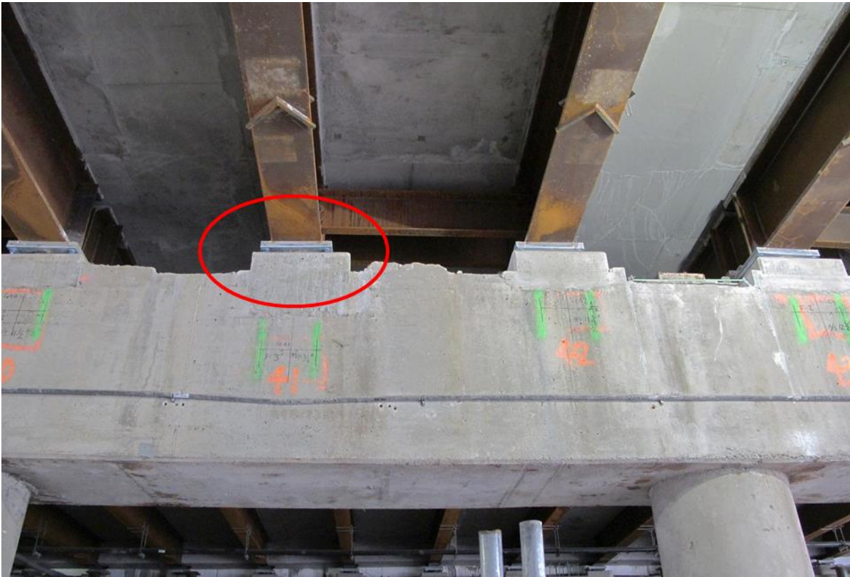
Figure 17. Photo. Pedestal placement for beam seats.
