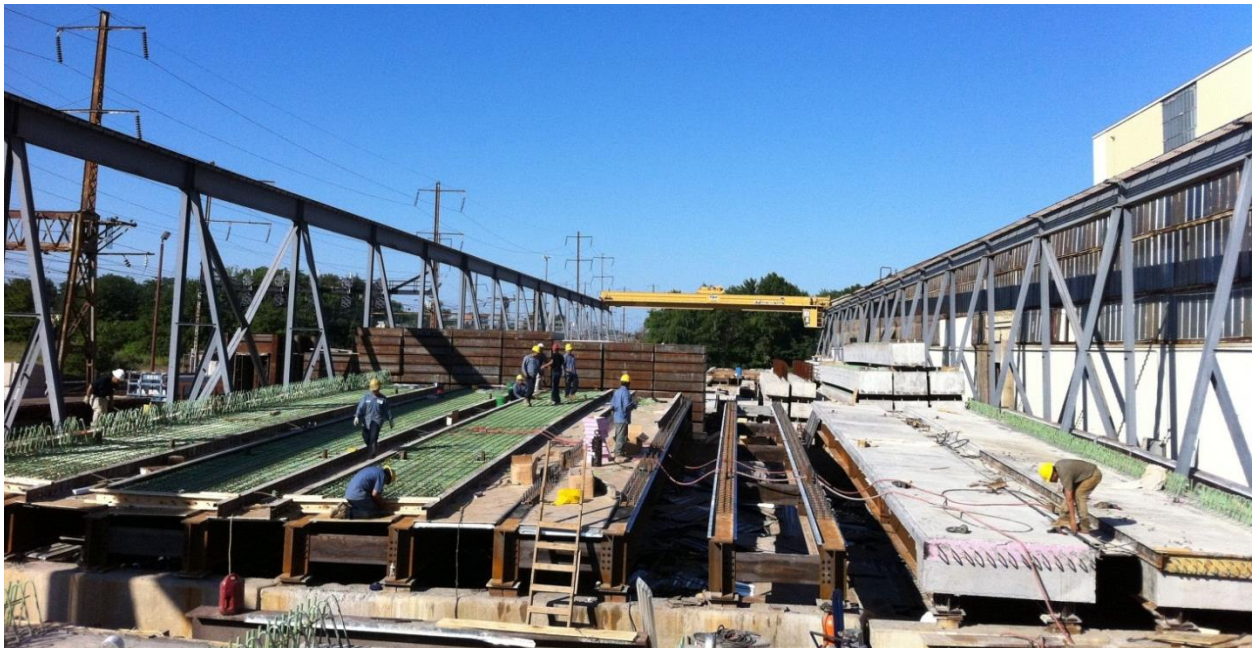
Figure 12. Photo. Typical form table assembly.
