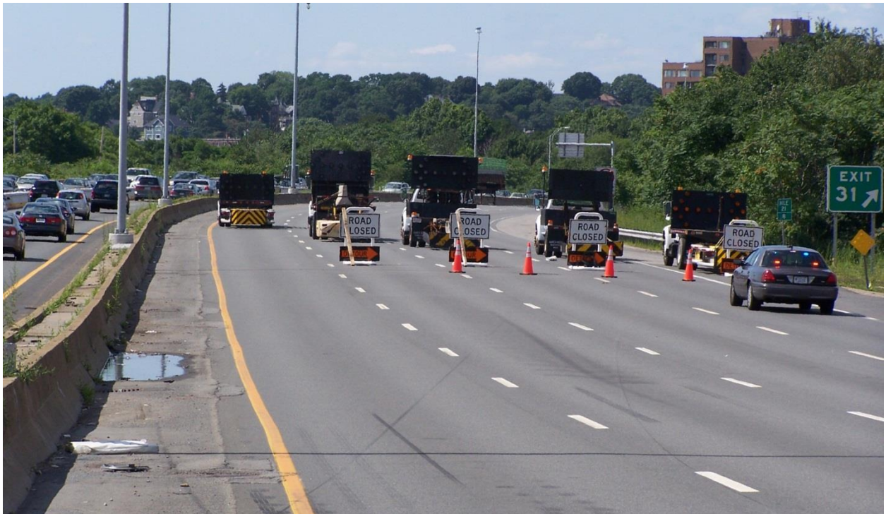
Figure 32. Photo. Work area protection.
