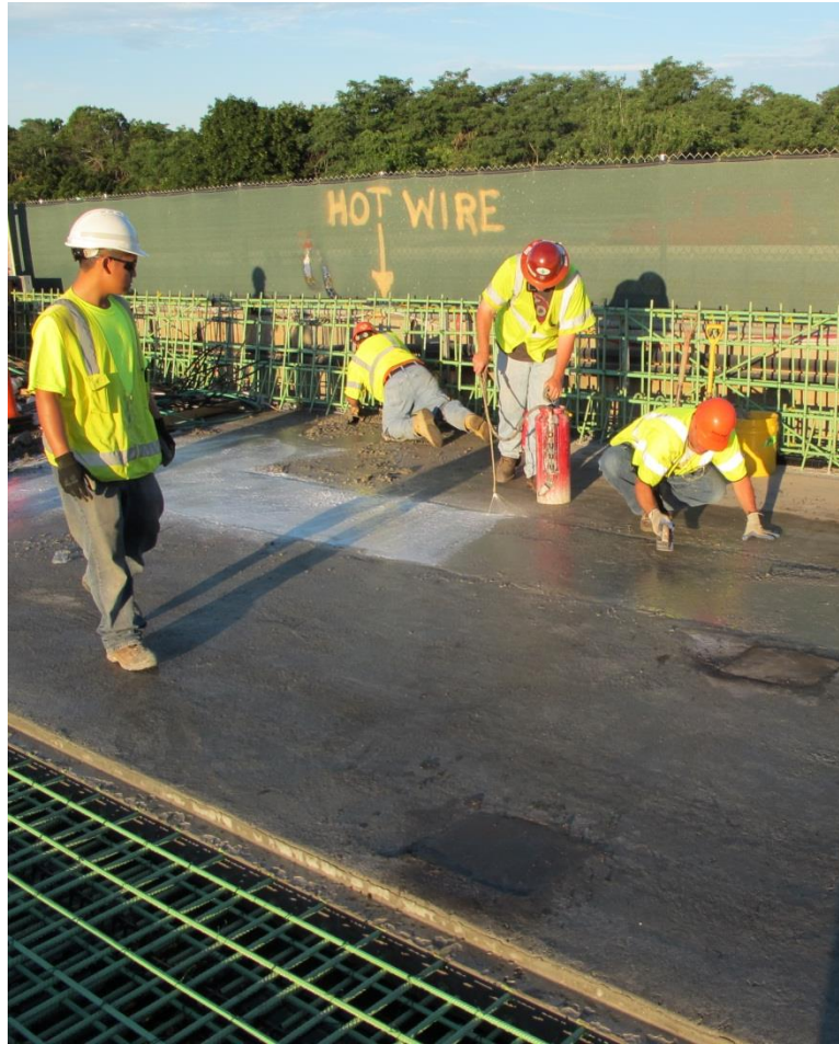
Figure 21. Photo. Curing and protection of concrete at bridge deck closure pours.
