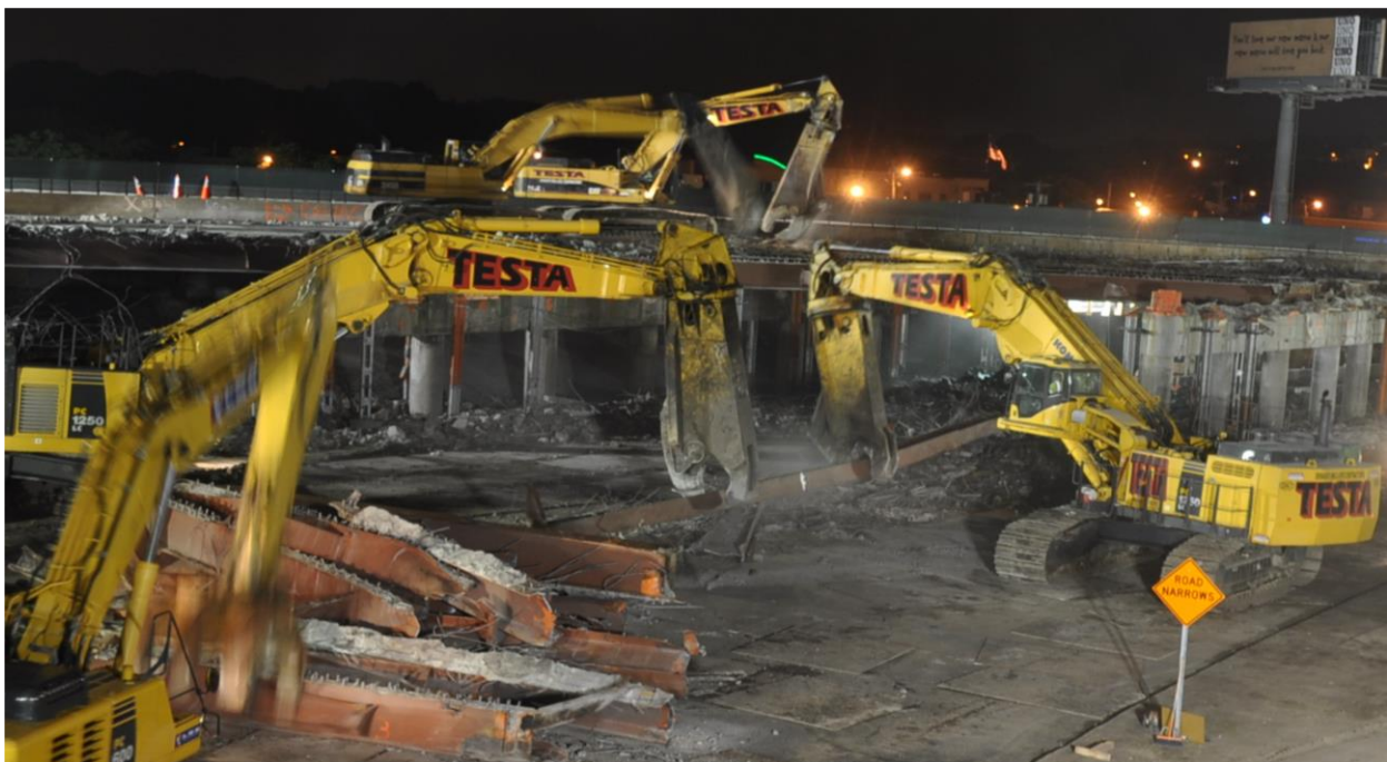
Figure 18. Photo. Demolition of existing bridge superstructure.
