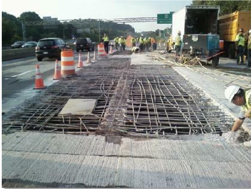
Figure 3. Photo. Deck condition on I-93 over Valley Street prior to construction.
