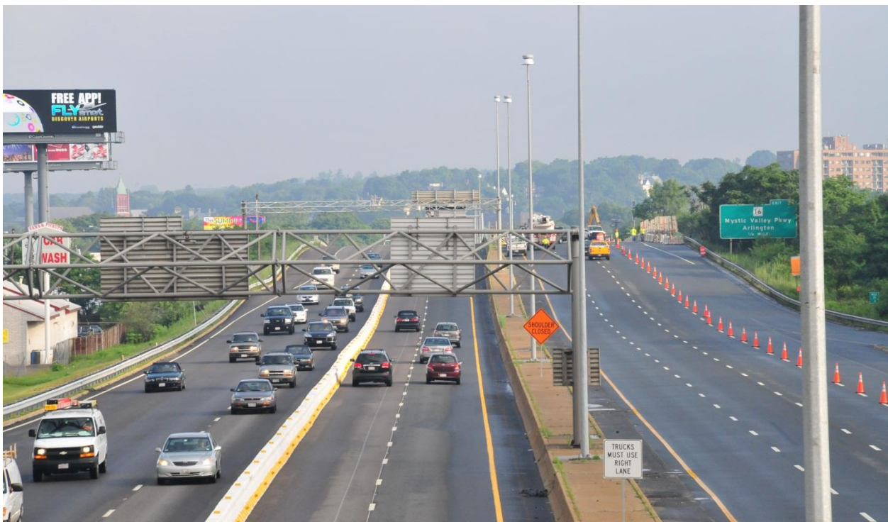
Figure 26. Photo. Movable barriers facilitating counter-flow traffic at crossovers.
