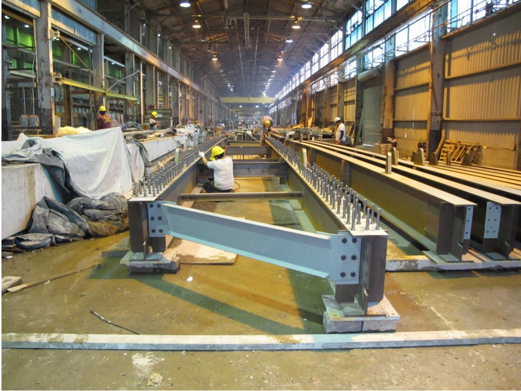
Figure 11. Photo. Form support angles.
