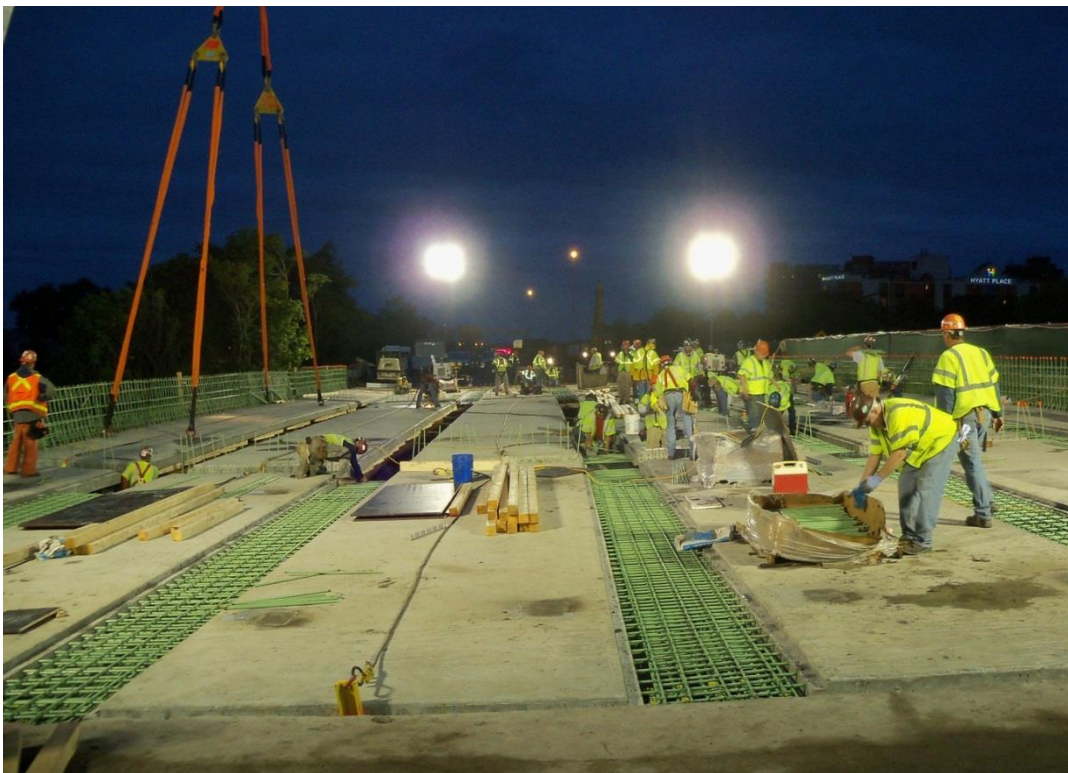
Figure 5. Photo. Wider closure pour for bridge decks.
