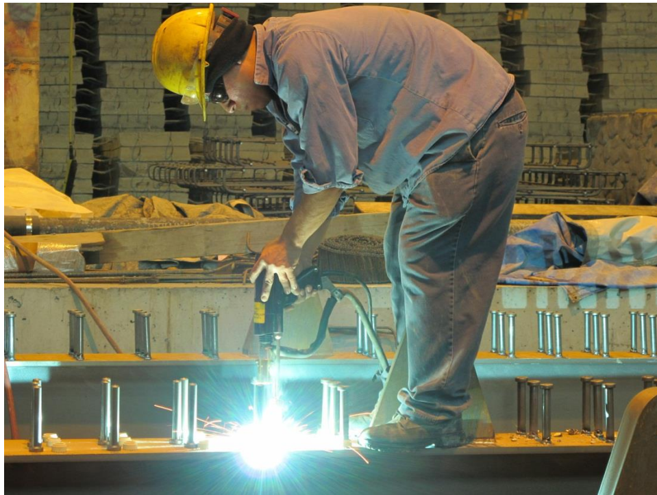
Figure 10. Photo. Shear stud welding.
