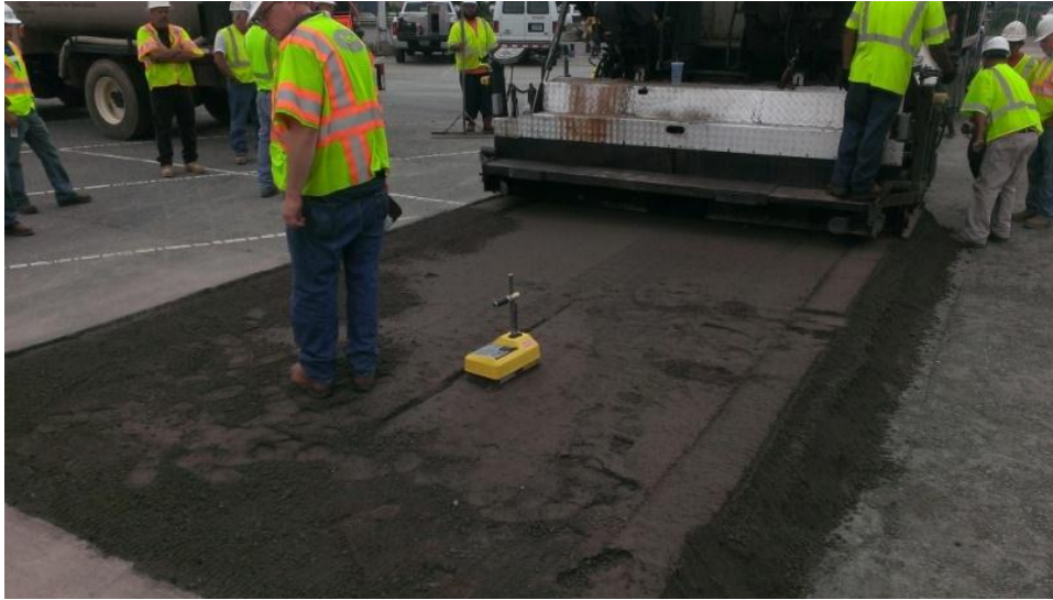
a) RCC placement at the test section
