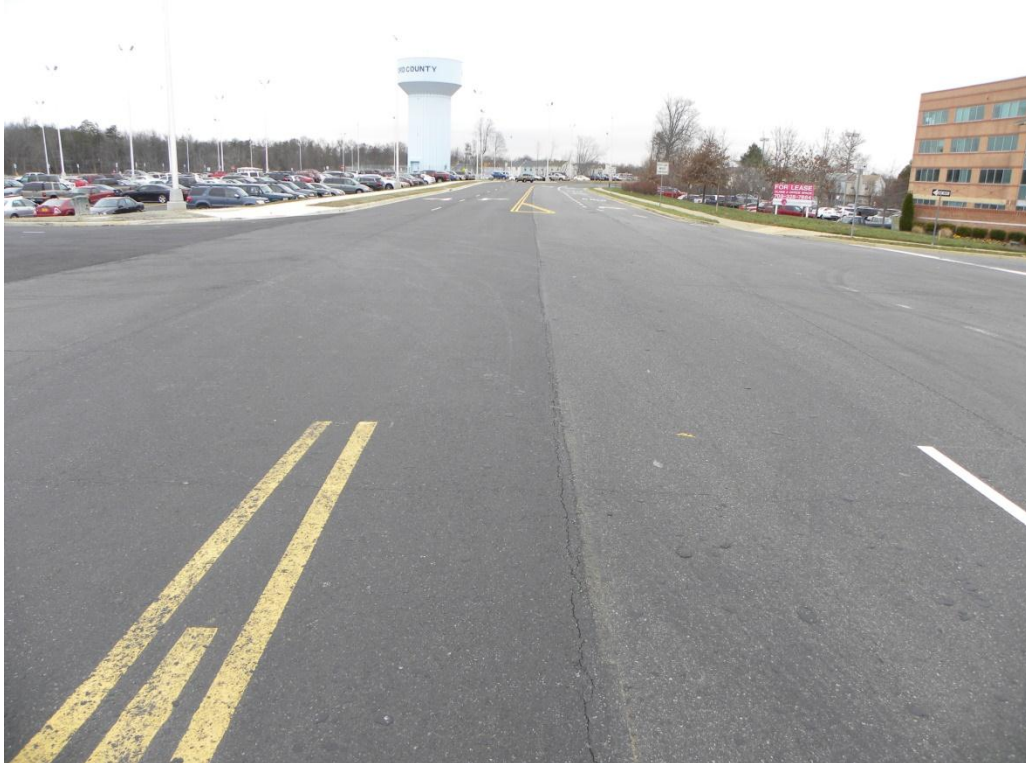
Figure 15. Photos. Completed portions of Staffordboro Boulevard with AC surfacing, as of December 2014.
