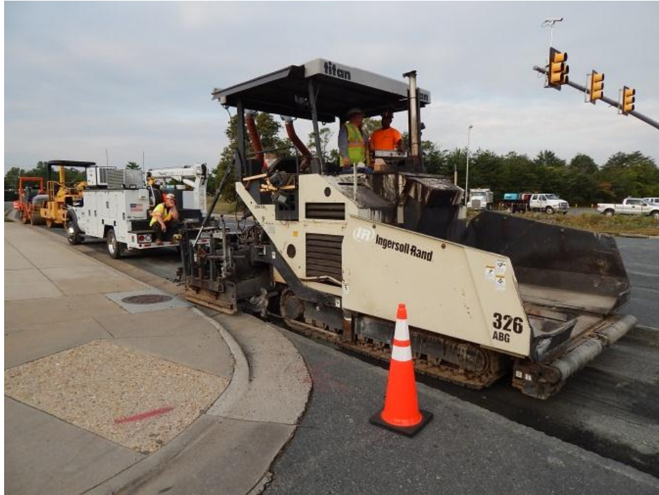
Figure 8. Photo. Asphalt paver used.
