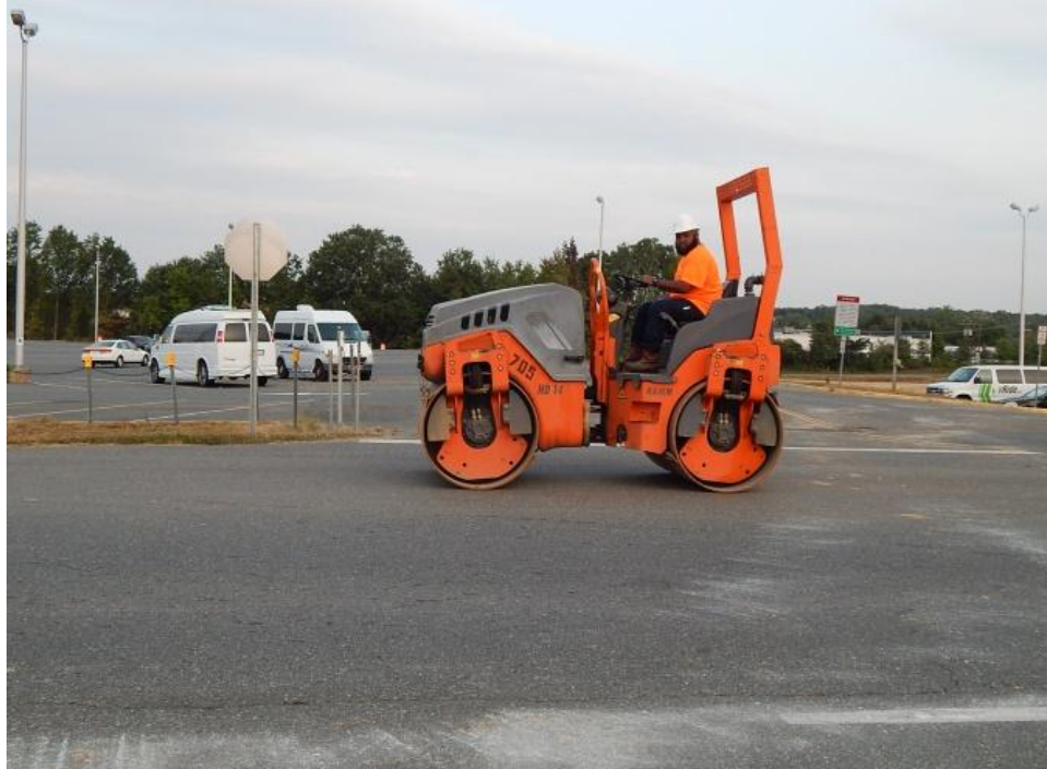
Figure 10. Photos. Asphalt roller used. Top - Primary Roller, Bottom - Finishing Roller.
