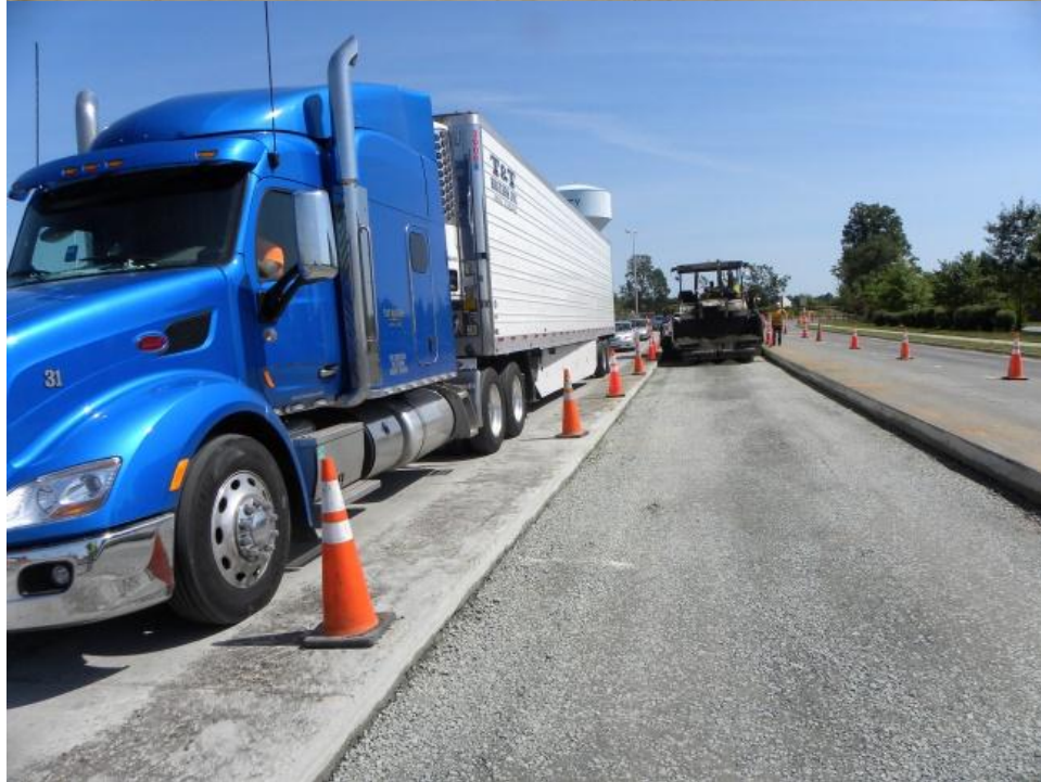
Figure 16. Photos. Traffic flow during RCC placement.
