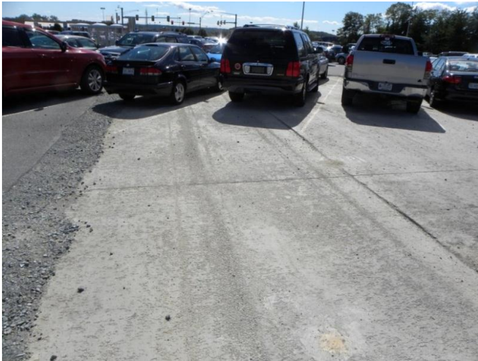
b) Completed RCC test sections
