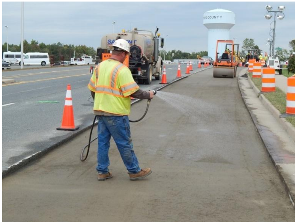
Figure 13. Photo. Water curing soon after compaction is completed.
