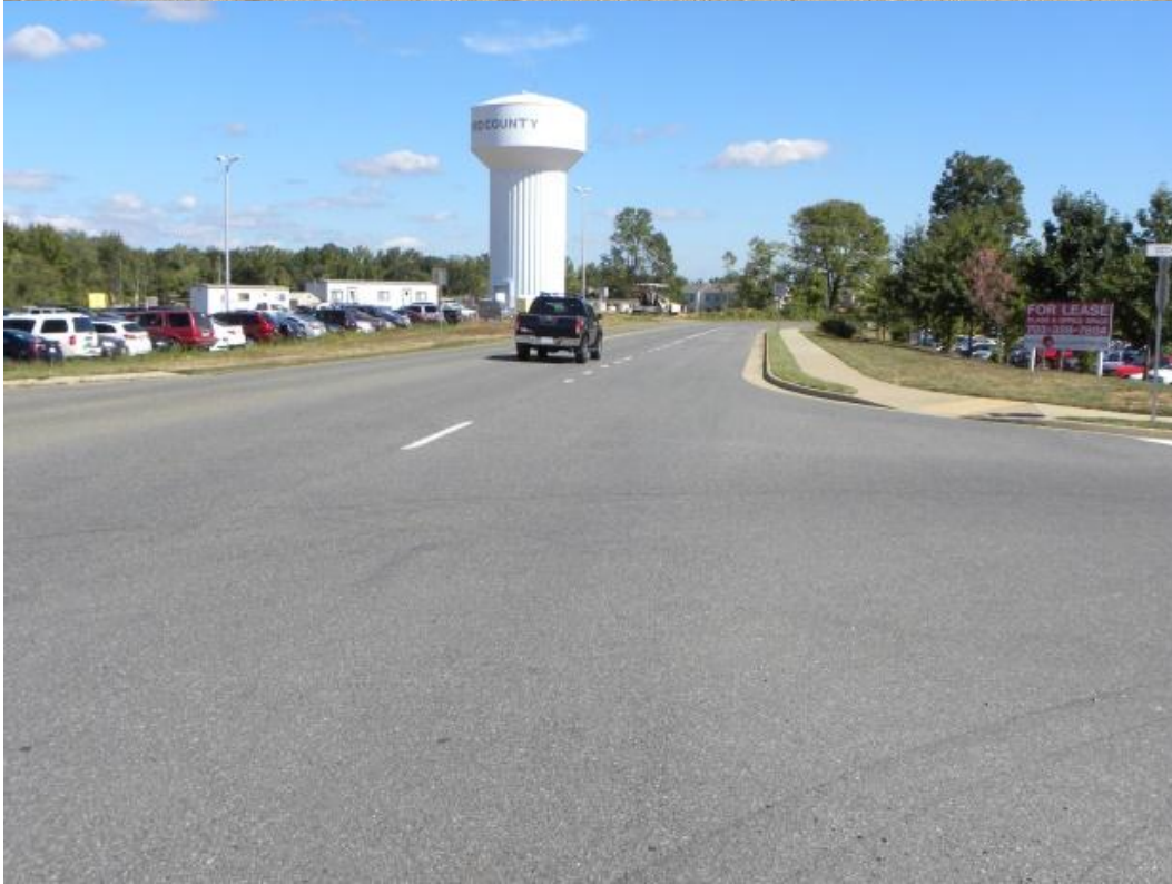
Figure 3. Photos. Views of Staffordboro Boulevard just prior to construction.
