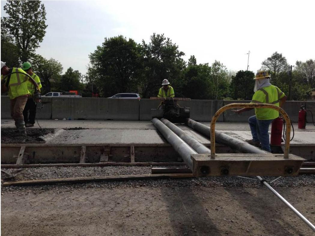
Figure 9. Photo. Tube rolling of concrete material.
