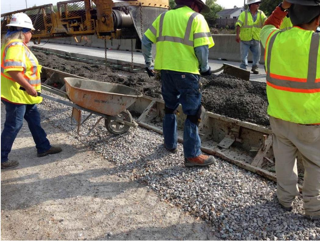
Figure 8. Photo. Placement of fresh concrete.
