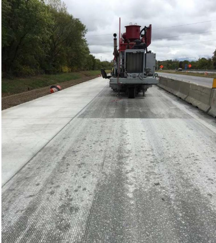
Figure 12. Photo. Application of NGCS – second pass.
