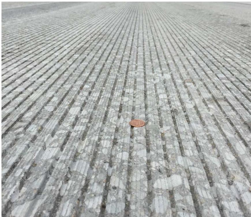
Figure 13. Photo. Concrete surface with double pass NGCS.
