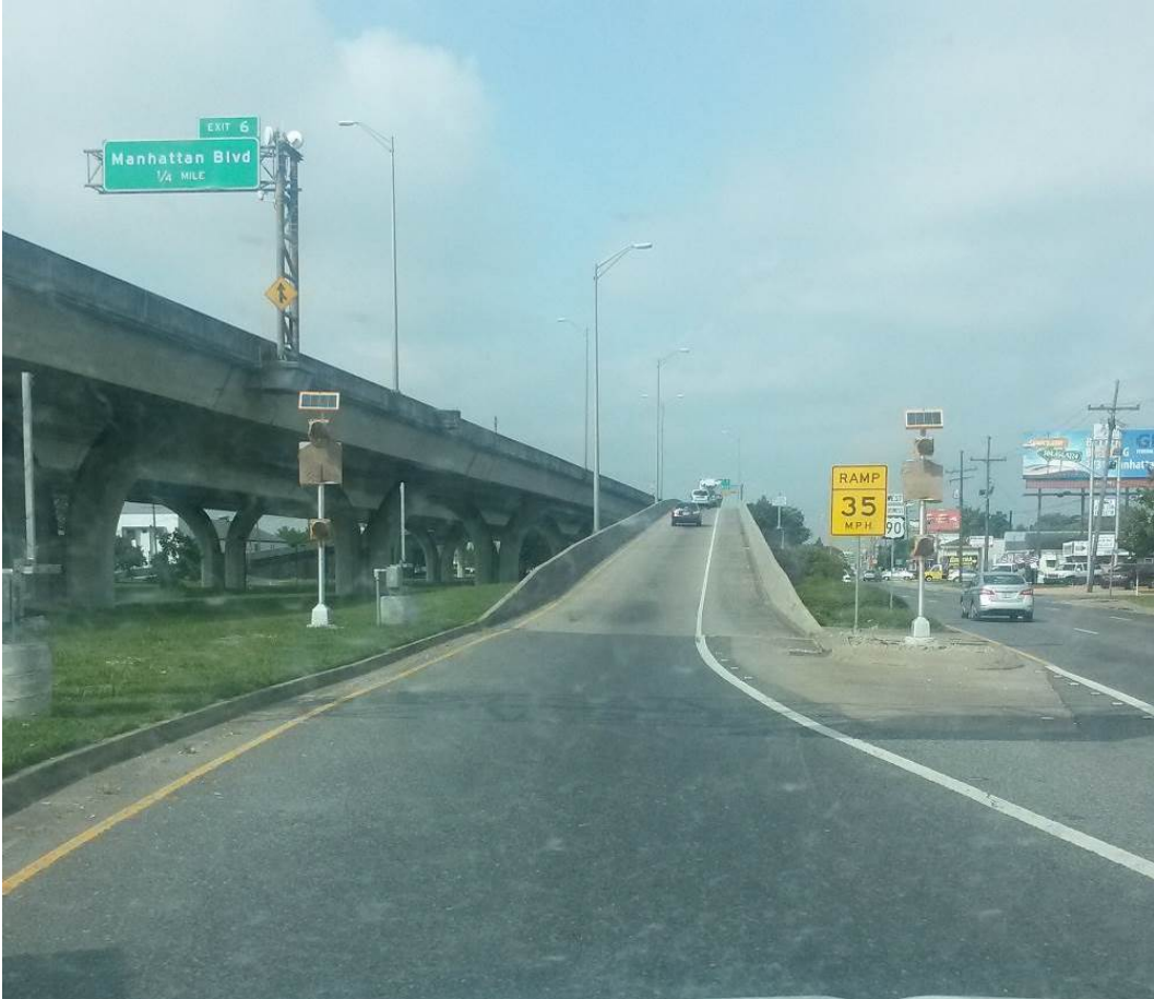
Figure 6. Photo. Foundations and poles for the automated gates.
