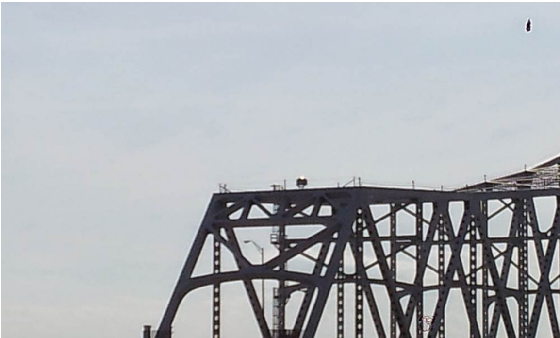
Figure 3. Photo. LADOTD's radar unit mounted on top of the Crescent City Connection Bridge No. 1.
