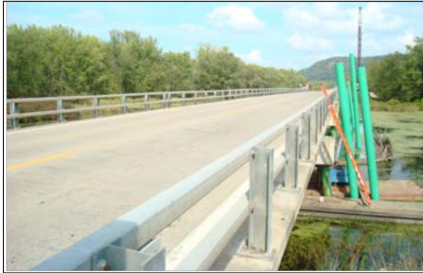
Figure 3. Bridge #2 showing the piles added to support the deck widening.
