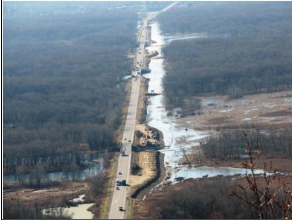
Figure 5. Aerial view of WIS 25 looking west toward Minnesota.
