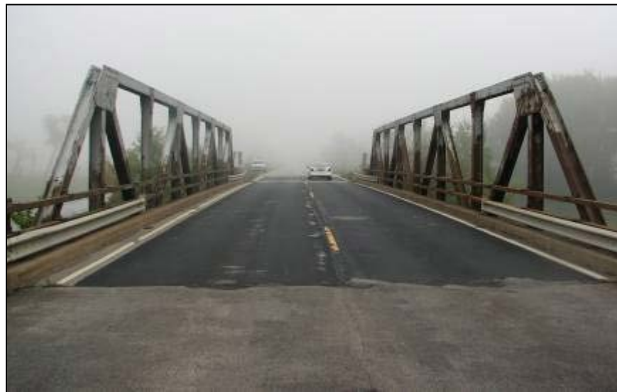
Figure 2. The pony truss bridge #1 prior to reconstruction.
