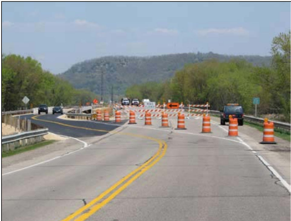
Figure 6. Temporary bypass bridge in use at bridge #3.
