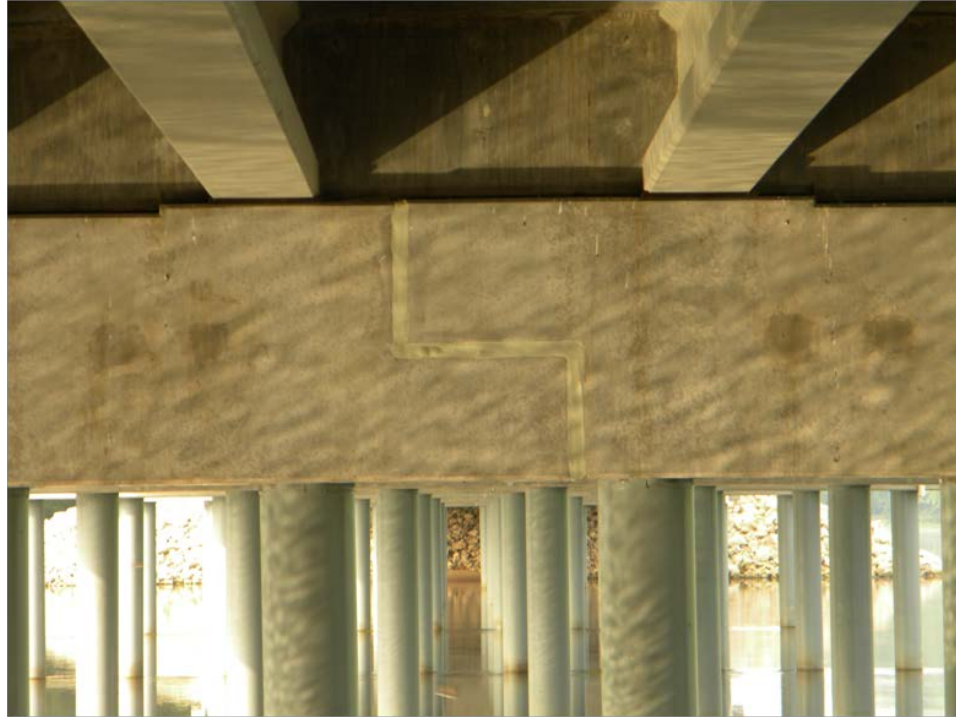
Figure 12. Sealed joint between the two halves of a completed pier cap.
