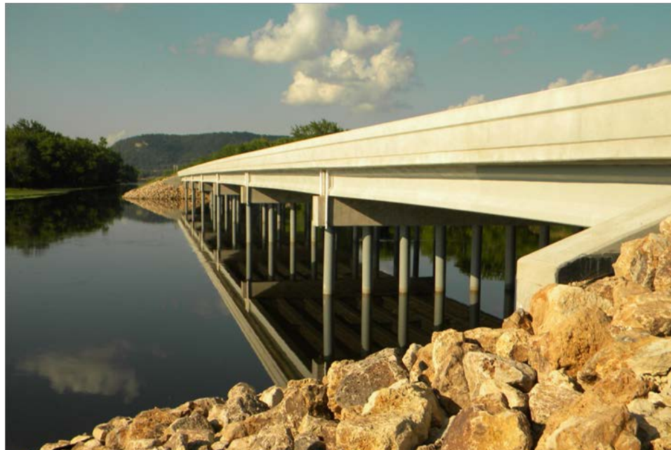
Figure 9. Finished open pile bents at bridge #3.
