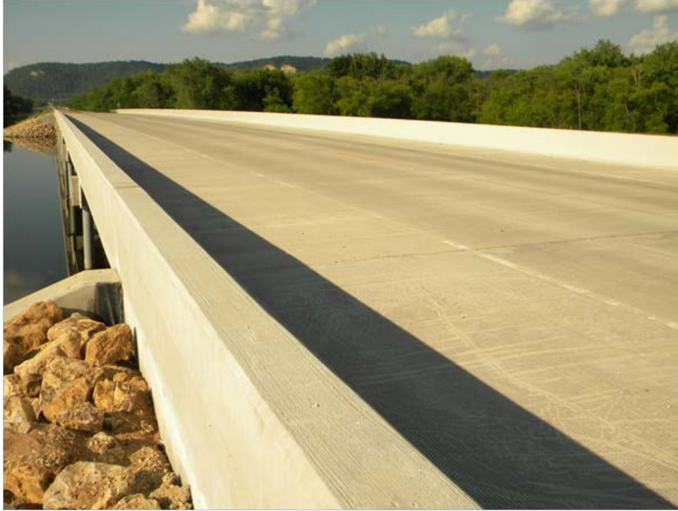
Figure 14. Finished deck of bridge #3.
