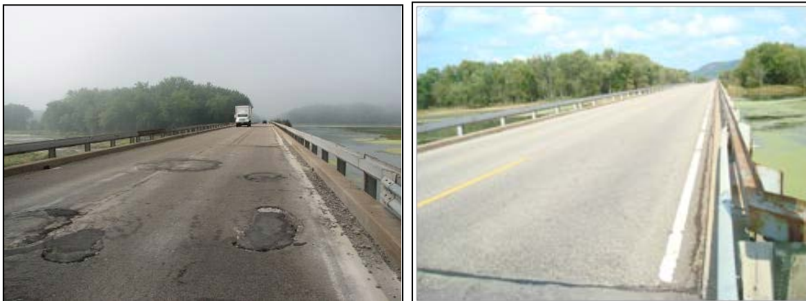
Figure 4. Existing bridge #3 (left) and existing bridge #4 (right).
