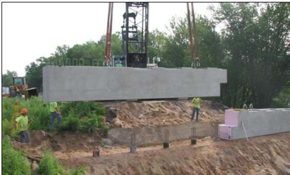
Figure 11. Precast abutment section being lowered into place (source: WisDOT).
