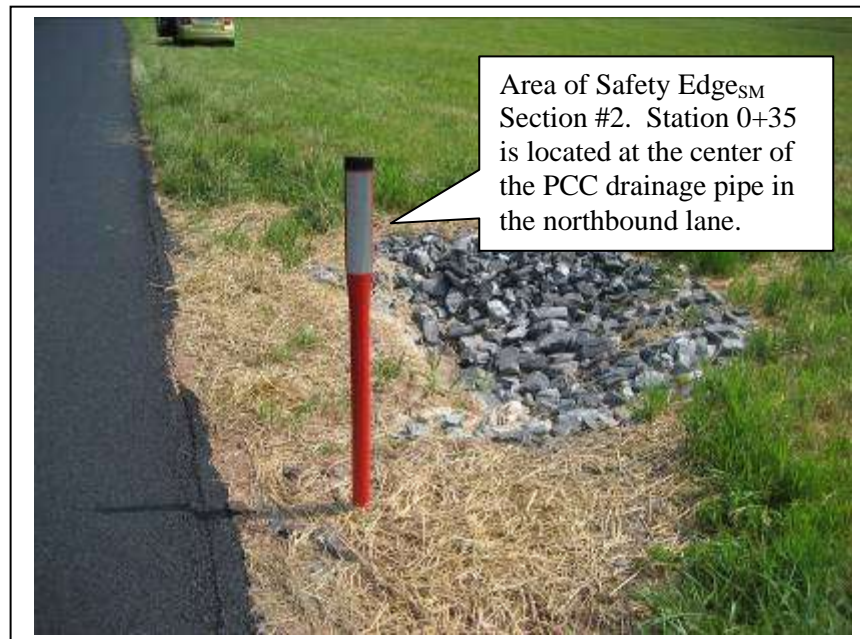
Figure 7. Reference marker for Safety Edge SM Section #2.
