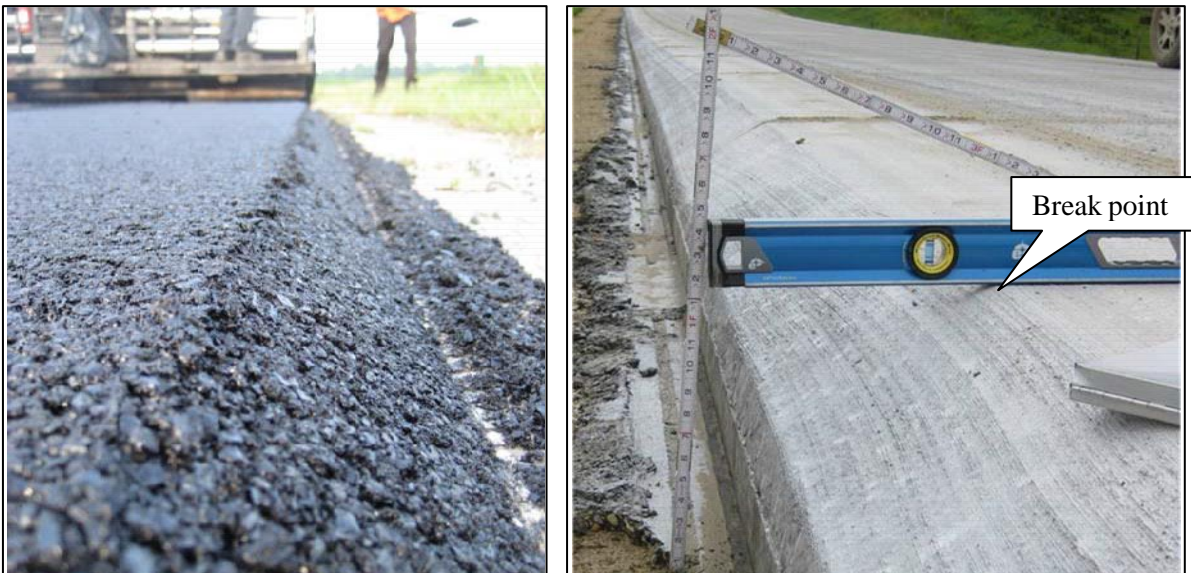
(a) AC Project.
