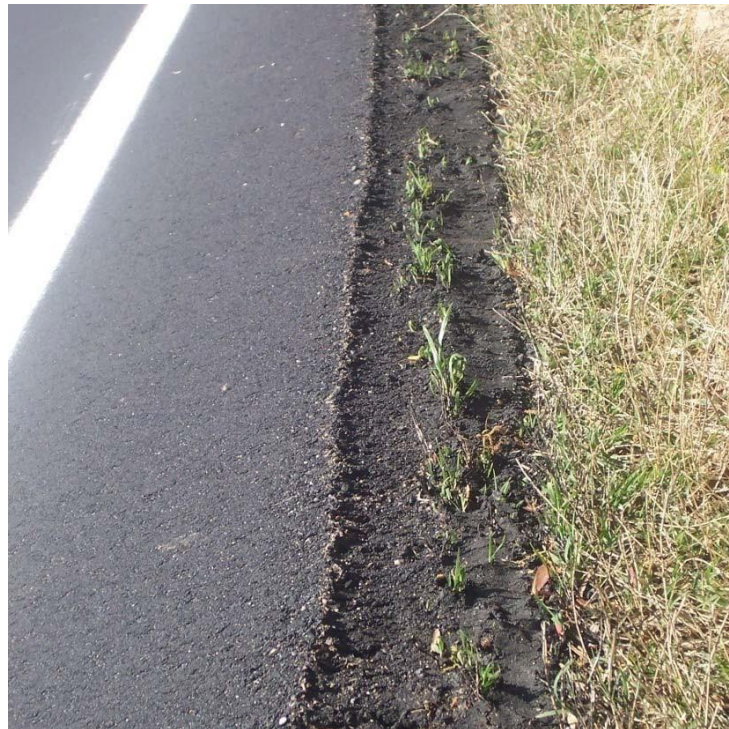
Figure 6. Example of Safety Edges SM placed on heavy vegetation – due to lack of adequate compaction the Safety Edges SM will deteriorate.
