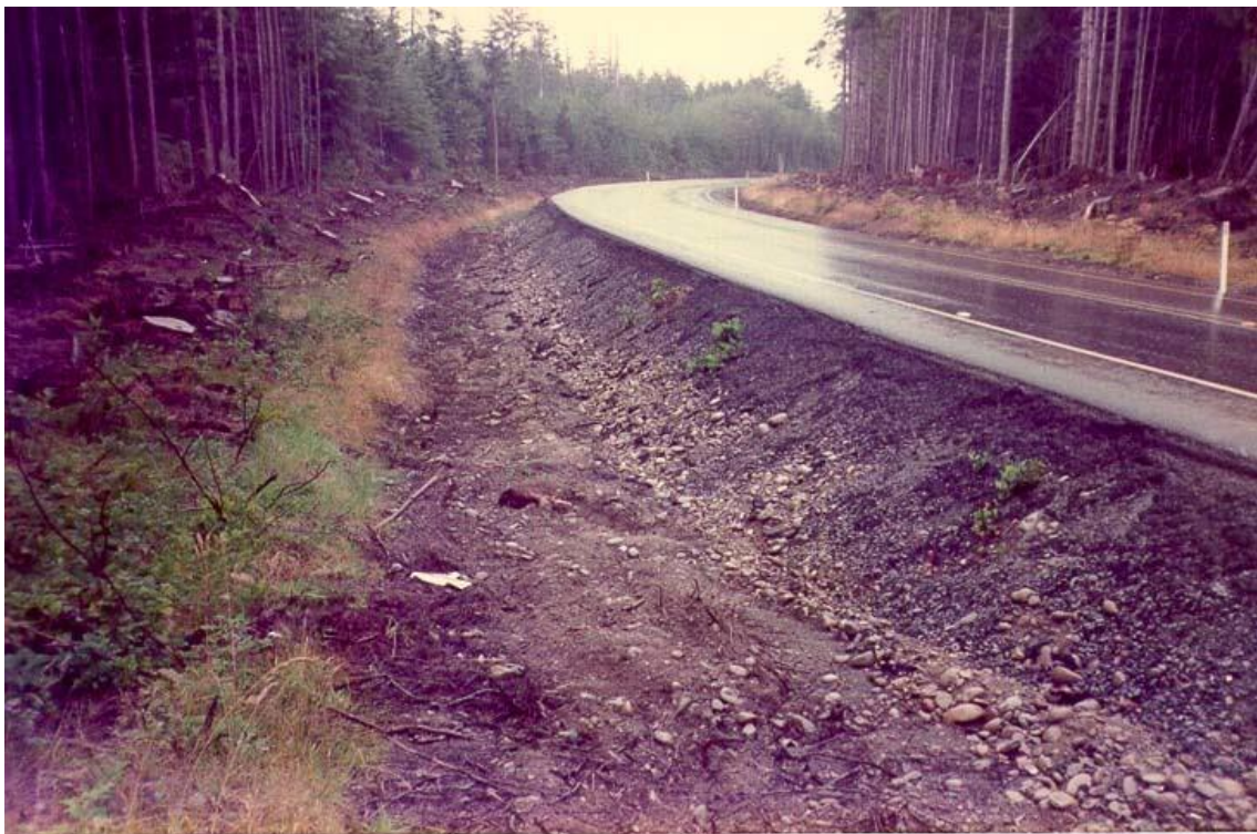
Figure 2. Example of where a foreslope/embankment is too steep for the Safety Edges SM .
