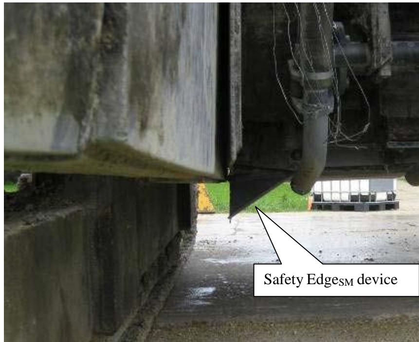
Figure 15. View of the Safety Edges SM device from front of paver.
