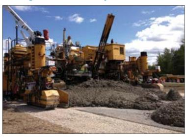
rehabilitation project on U.S. 10 in Midland County. This 6.9-mile project included the rehabilitation of eight bridges and the existing roadway. The project also included an alternate pavement bidding (APB) component, in which contractors could base their bid on rubblizing the existing pavement and placing an HMA overlay or constructing a concrete overlay.
