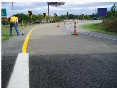
**FIGURE 2:** HFST at horizontal curve
