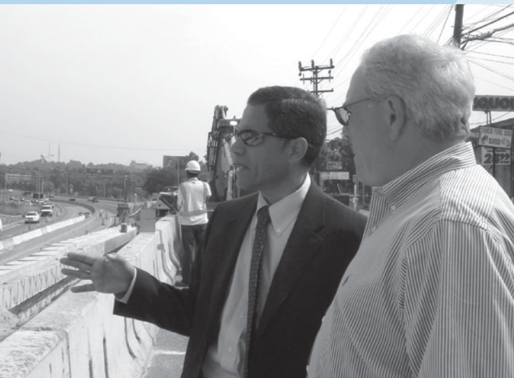
FHWA Administrator Victor Mendez (left) and Butch Marcelle of Fort Miller Co. check progress on a Washington, D.C., bridge project using prefabricated components to speed construction and reduce traffic impact.
