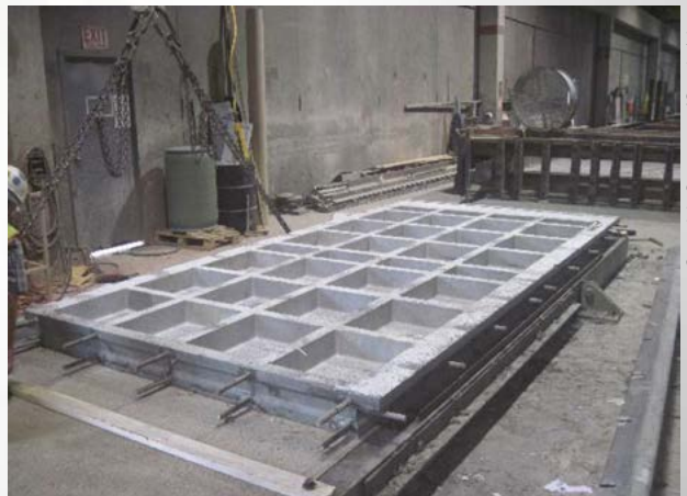
UHPC deck panels with a unique waffle shape were prefabricated for use on a bridge project in Iowa.
