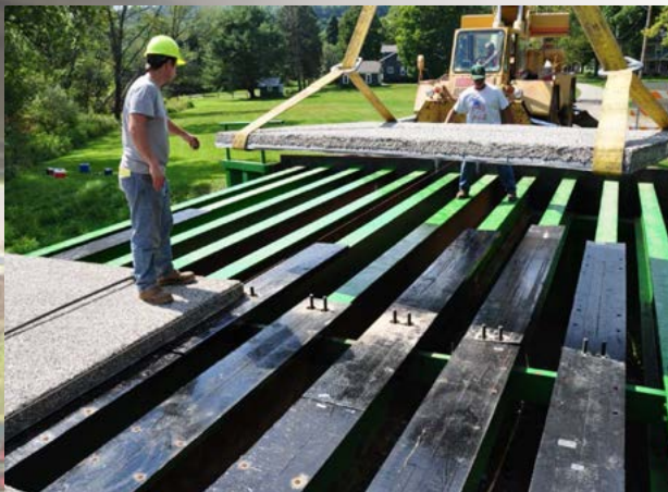
Lightweight, corrosion-resistant composite bridge decking was tested on a project in New York.
