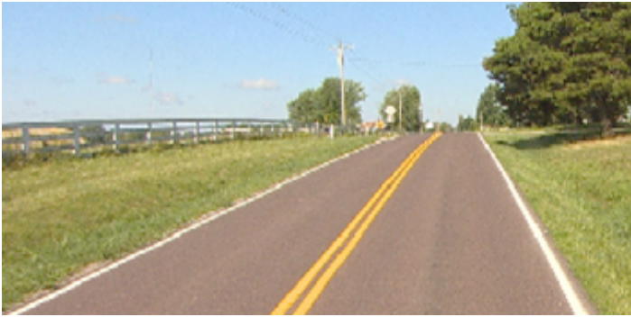
Using a systemic approach, the Missouri DOT added edgeline stripes to improve safety on rural roads such as Route M in Boone County.
