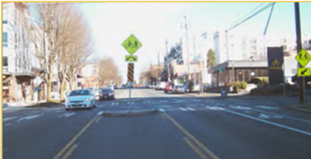
The Stone Way road diet in Seattle, Washington, improved pedestrian and bicycle safety by incorporating pedestrian refuge islands and a combination of shared lanes and bicycle lanes.
