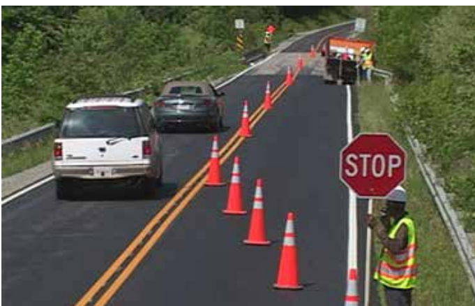
The North Carolina DOT collects data on the mobility impacts of manual flagging operations on rural roads.
