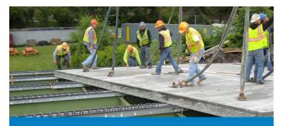
UHPC connection details make using prefabricated bridge elements simpler and more effective for accelerated bridge construction.
