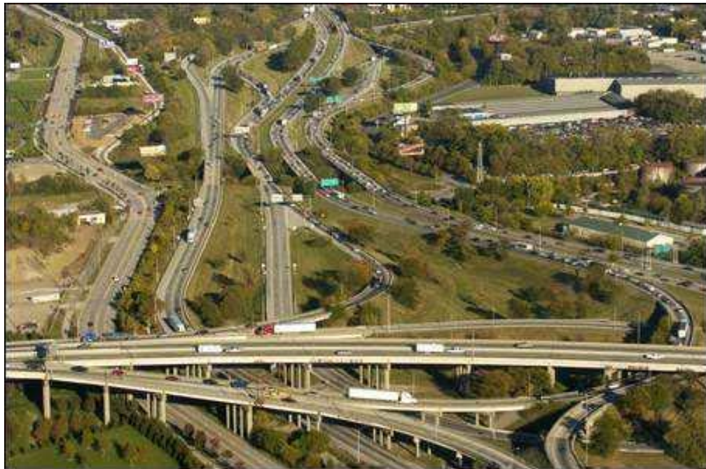
Existing Kennedy Interchange, Louisville, KY
