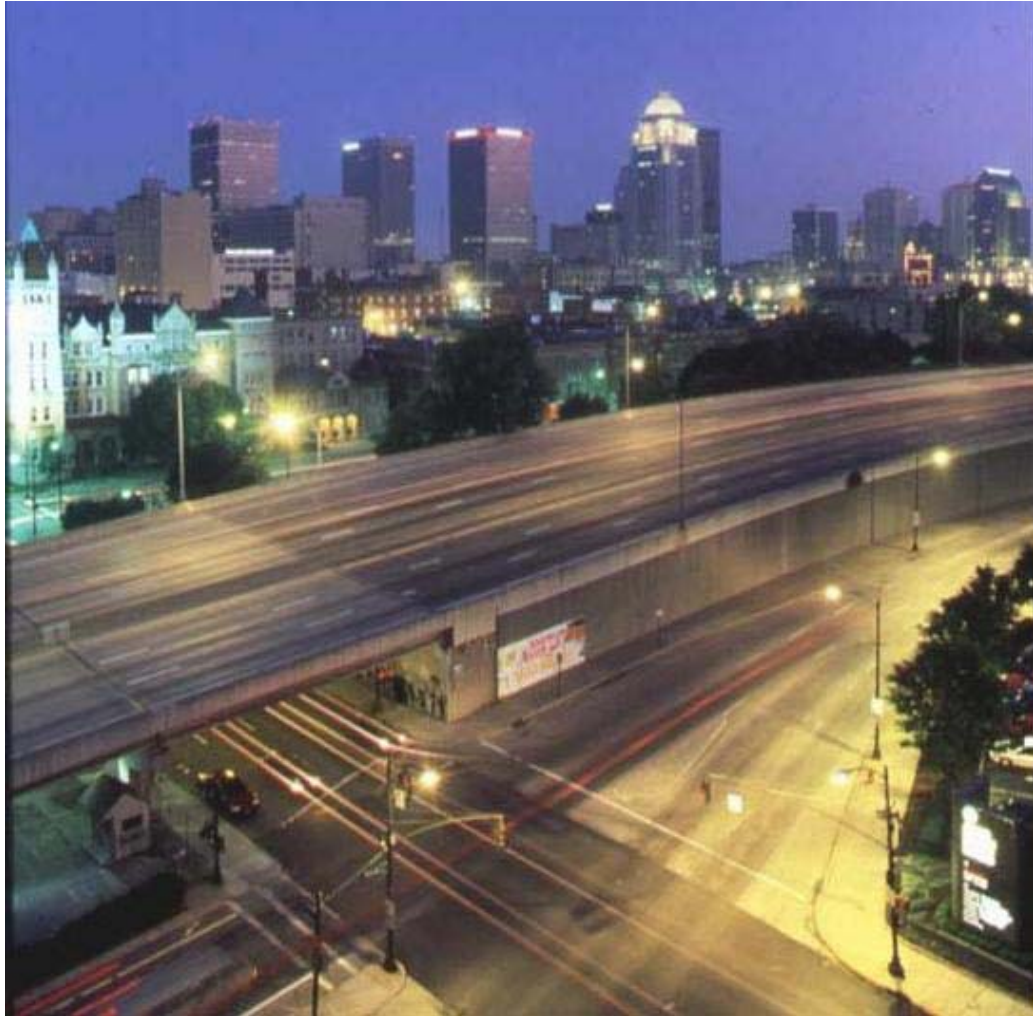
I-65 over East Broadway, Downtown Louisville
