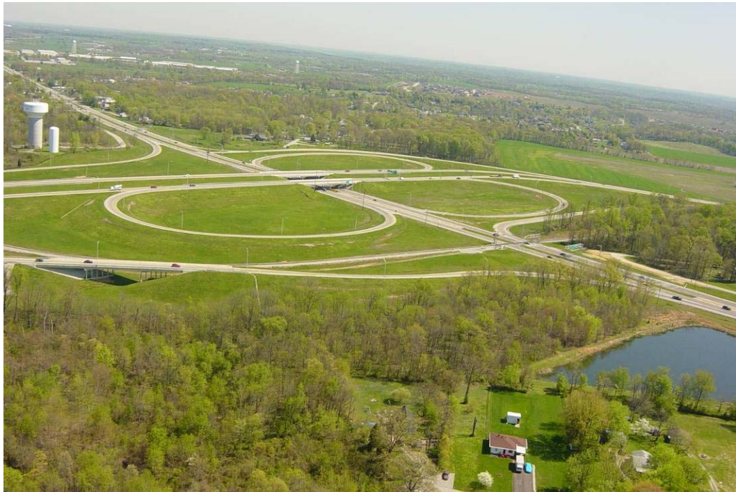
IN 265/SR62 /Port Road Interchange, Jeffersonville, IN
