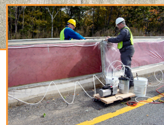
Pavement joint damage on an ASR-affected pavement near Mountain Home, ID (top); Vacuum impregnation treatment on ASR-affected highway barriers near Leominster, MA
