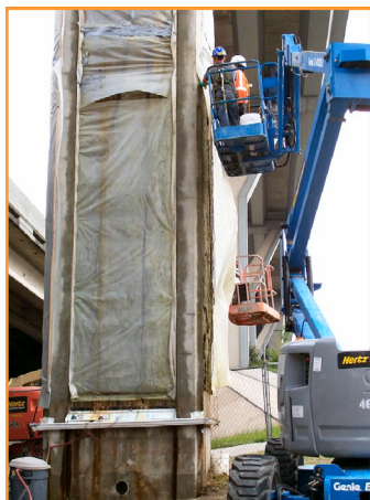
Electrochemical treatment on ASR-affected columns in Houston, TX
