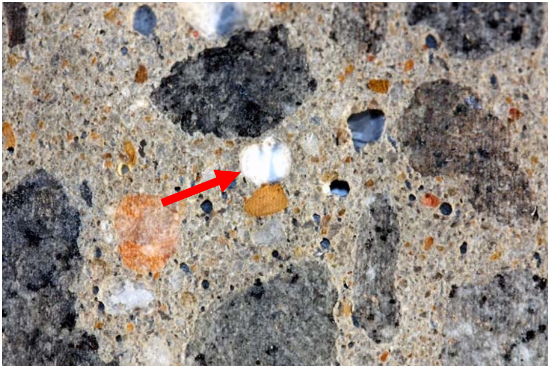
Figure A8: Details on core Ark-4. A: cracks in the cement paste running through a reactive sand particle; B: crack with alkali-silica reaction product in a reactive particle of the fine aggregate; C: air void filled with alkali-silica reaction product.
