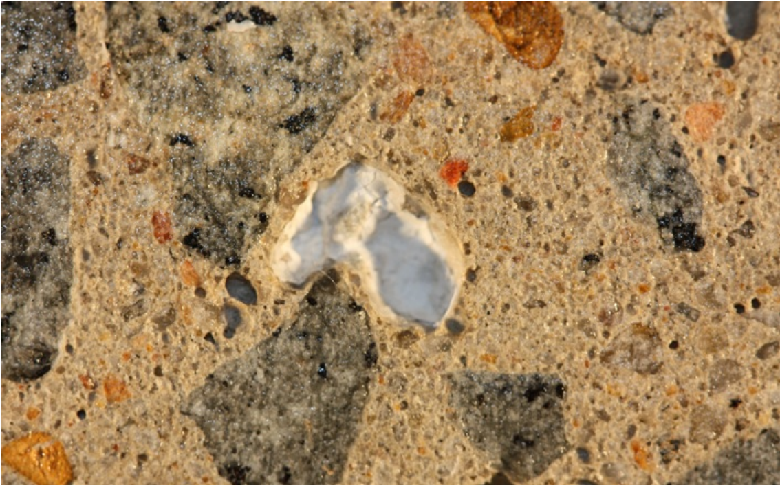
Figure A4: Details on core Ark-2. A: disaggregated/reacted aggregate particle; B: crack in the cement paste running through a reactive sand particle; C: air void filled with alkali-silica reaction product.
