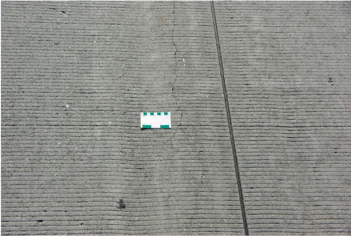
Figure A3 Cracking (0.03 – 0.06-in.) in panels where Cores #5 & #6 are located
