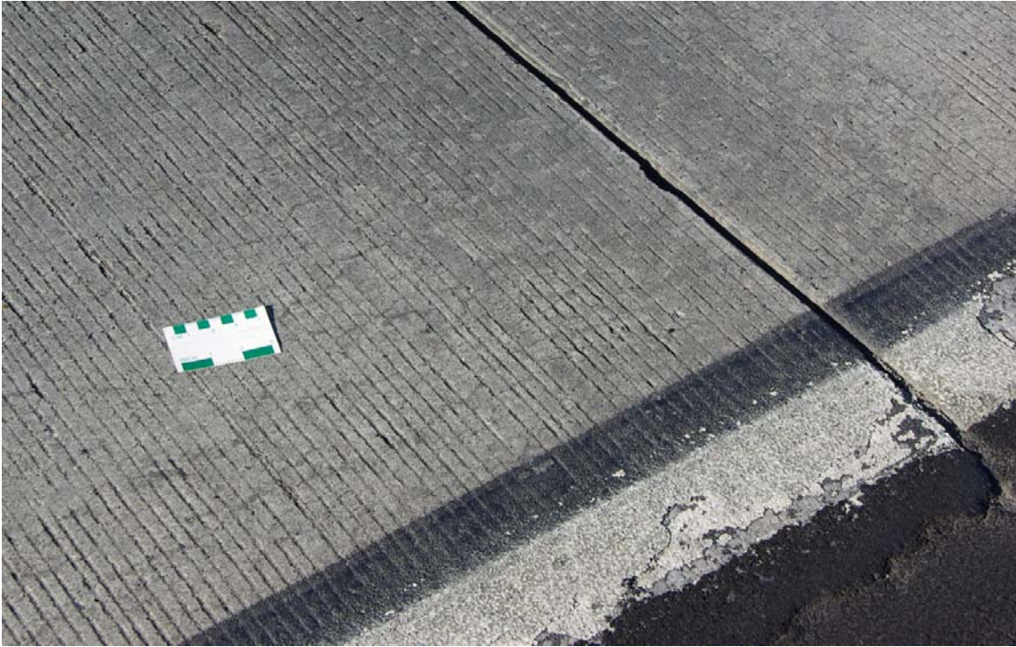
Figure A1 Staining around pavement joints
