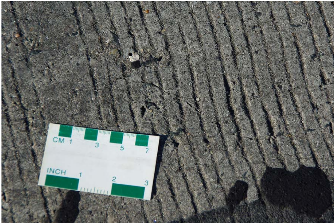
Figure A2 Hairline cracking (< 0.015-in) in panel where Core #3 is located
