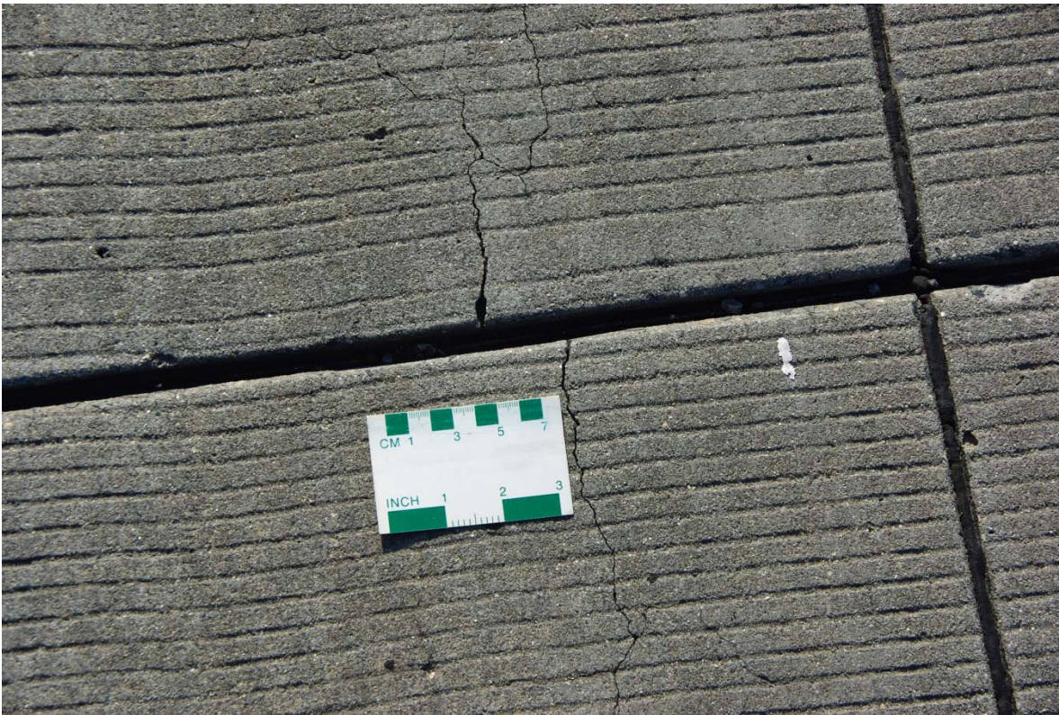
Figure A4 Close-up of Cracking (0.03 – 0.06-in.) in panels where Cores #5 & #6 are located
