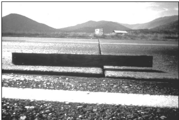
Figure 1. Diamond grinding can be used to correct surface irregularities such as faulting (difference in elevation across a joint or crack).
