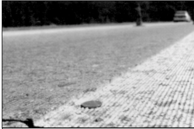
Figure 5. Final "corduroy" texture produced by diamond grinding.
