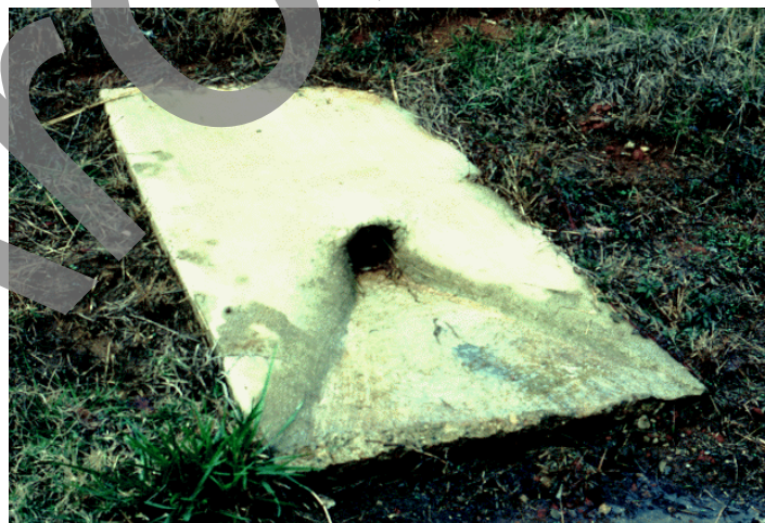
Photo No. 8 Large Outlet Pipe Headwall
