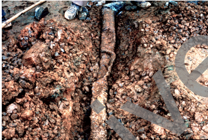
Photo No. 9 Crushed Edgedrain Pipe
