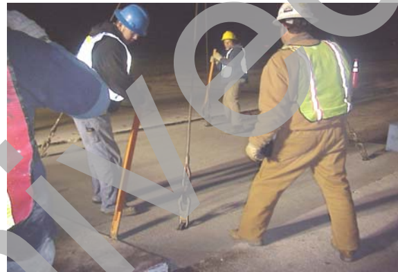
c) Alignment of panel.
