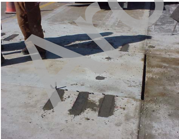
d) Back-filled dowel slots.
