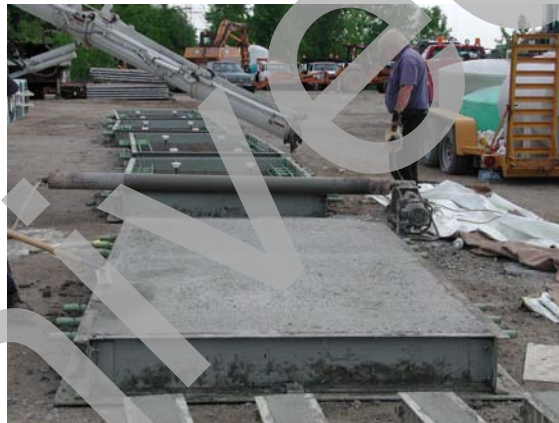
c) Texturing of fresh concrete.
