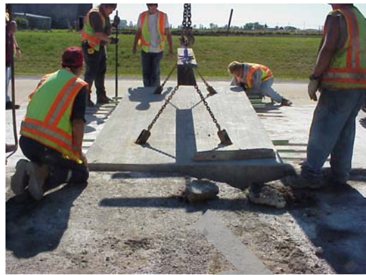
b) Panel installation and alignment.
