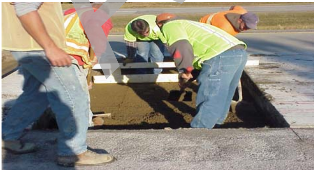
Figure 5. Initial cleaning and preparation of the base.
