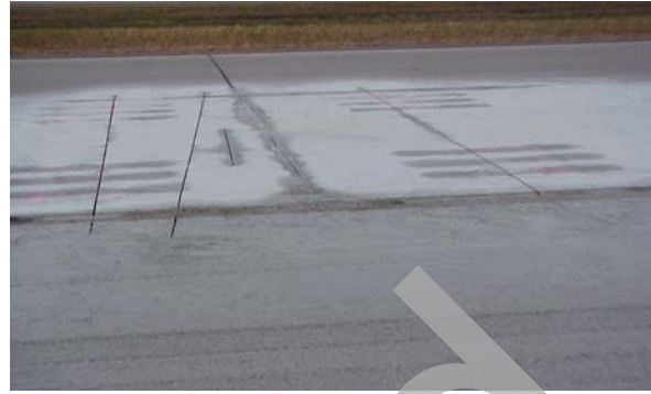
b) The existing slab after sawcutting.
