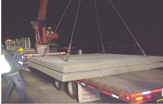
a) Panel moved from flatbed truck.
