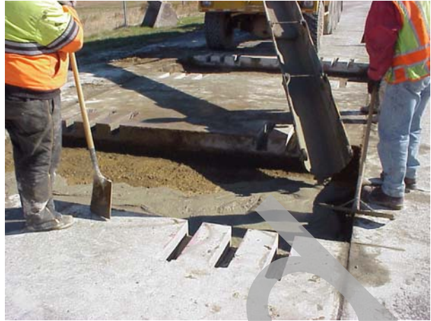
b) Leveling of flowable fill.
