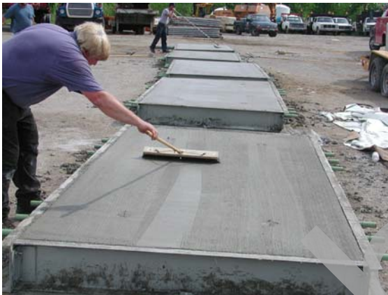
b) Concrete placement for precast panels.
