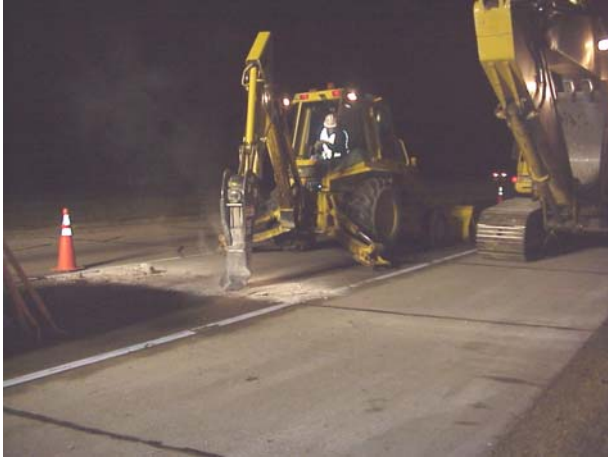
a) Slab demolition
