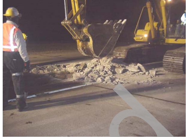
b) Removal of debris
