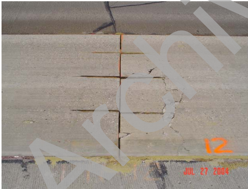
Figure 35. Typical crack patterns.
