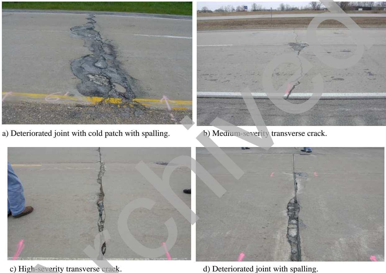
Figure 3. Typical distresses.
