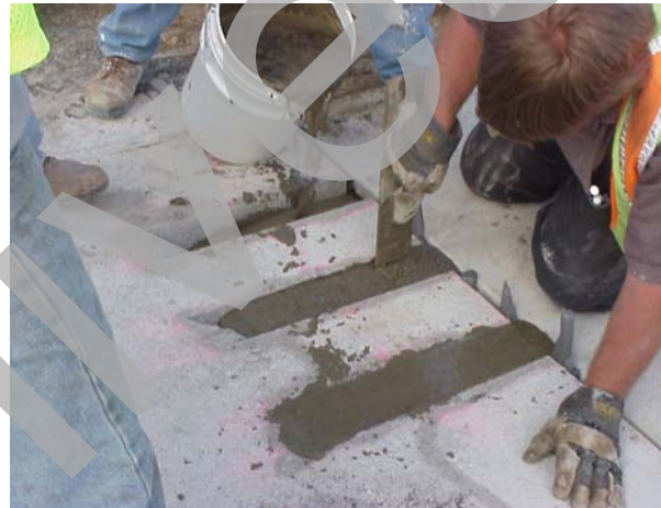
b) Leveling of flowable fill.
