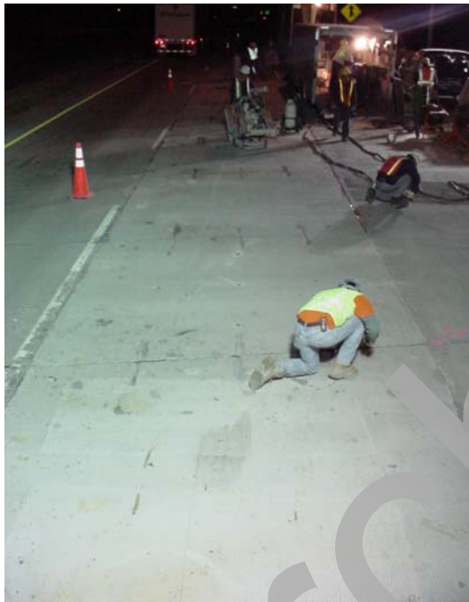
Figure 26. Completed cluster of panels.
