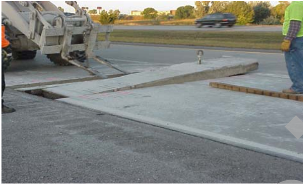
c) Removing the existing slab.
