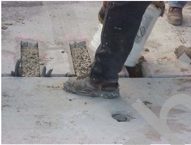
c) Back filling of dowel slots.
