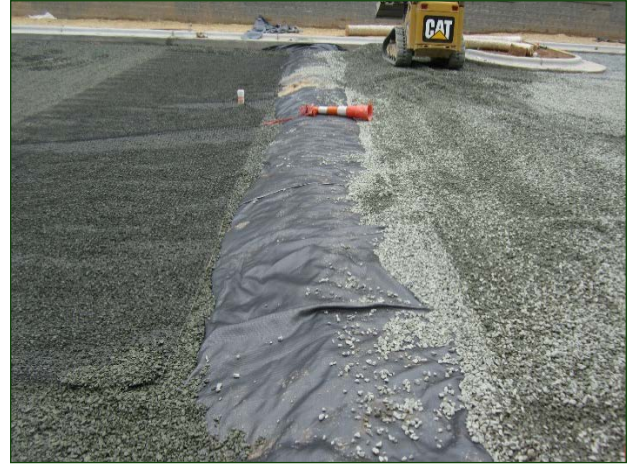
Figure 12. Aggregate and impermeable liner flow barrier
