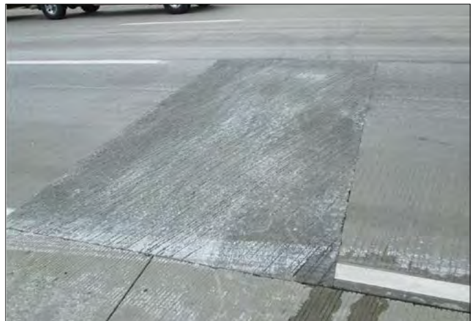
Figure 72. Completed FDR in CRCP.
