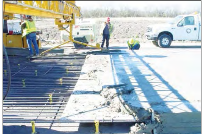
Figure 44. Wooden panels temporarily placed to facilitate removal of concrete carried over end-of-day header.
