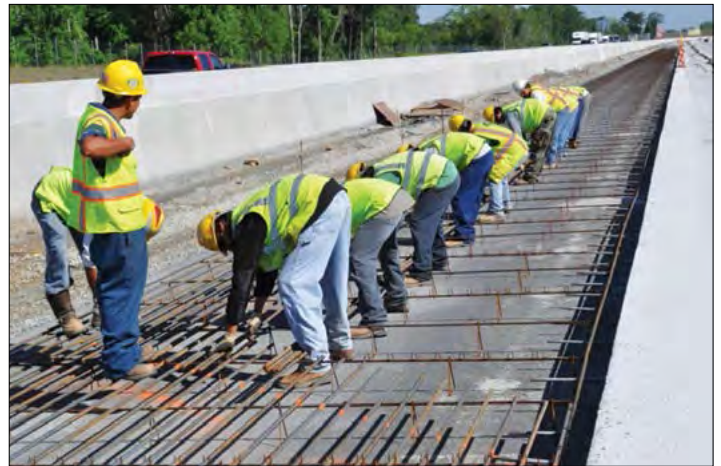
Figure 35. Placing longitudinal steel on TBAs.
