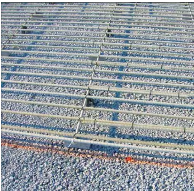
Figure 65. GFRP longitudinal reinforcement for CRCP (Canada).
