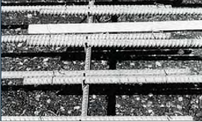
Figure 59. Longitudinal reinforcement lap splices and ties.
