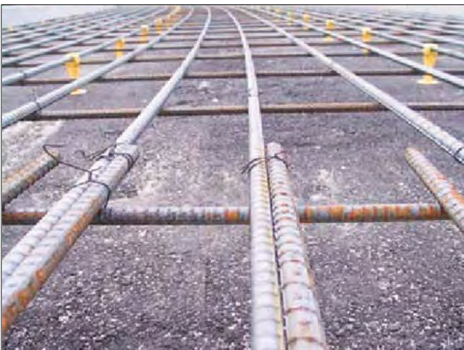
Figure 24. Lap splices.
