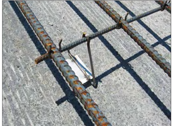
Figure 34. Transverse bar assembly (TBA).
