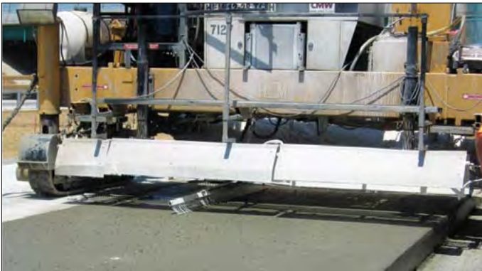
Figure 39. Applying transverse tining on a new CRCP.
