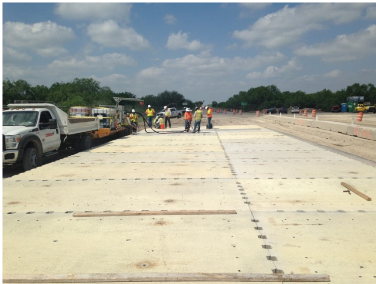
Figure 26. Photo. Stage 1 panel installation along SH 97.
