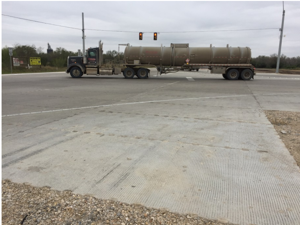
Figure 28. Photo. Completed intersection in use – view from SH 97 (December 8, 2016).
