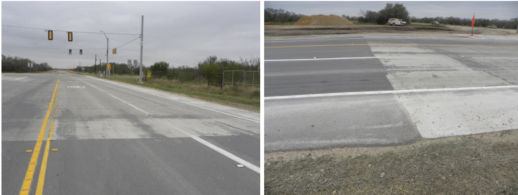
Figure 24. Photos. Views of completed transition areas.
