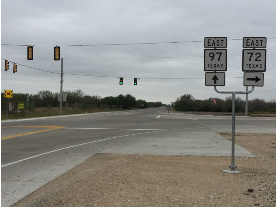
Figure 27. Photo. Completed intersection (December 8, 2016).
