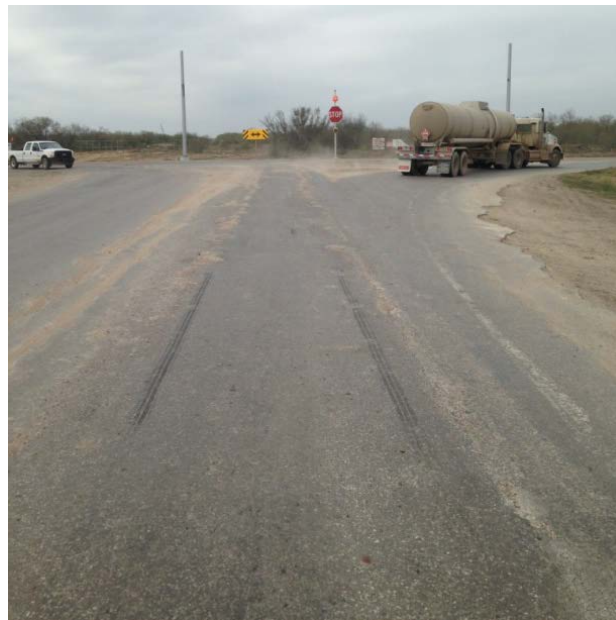
Figure 3. Photo. A view of the AC intersection before rehabilitation.
