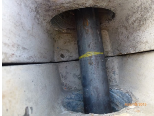
Figure 19. Photo. Dowel bar positioning in ducts of adjoining panels.
