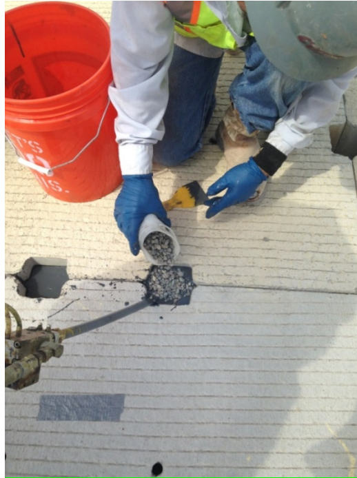
Figure 21. Photo. Use of pea gravel at the open slots.
