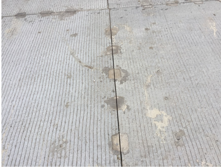
Figure 25. Photo. A sawed and sealed joint (December 8, 2016).
