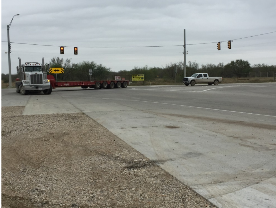
Figure 29. Photo. Completed intersection in use – view from SH 72 (December 8, 2016).
