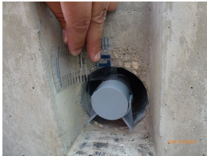
Figure 10. Photo. View of a dowel placed in the duct and resting on a mini-chair.
