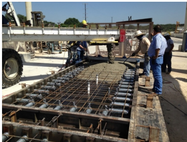
Figure 13. Photo. Concrete placement in the panel formwork.
