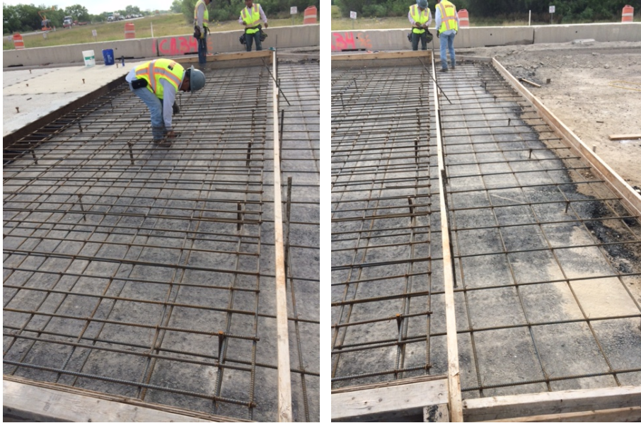
Figure 23. Photos. Formwork for the cast-in-place transition slabs.
