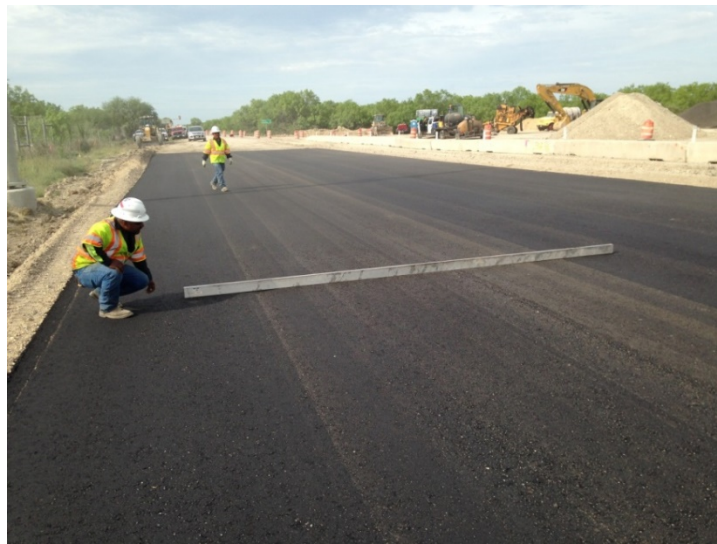
Figure 14. Photo. AC base layer.
