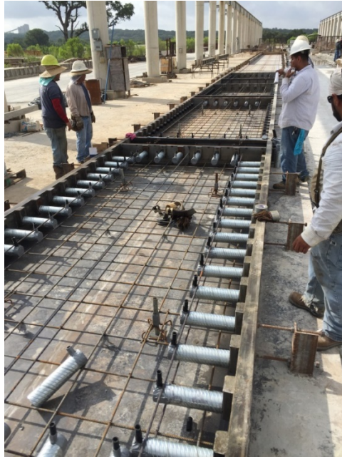
Figure 12. Photo. Panel formwork setup.
