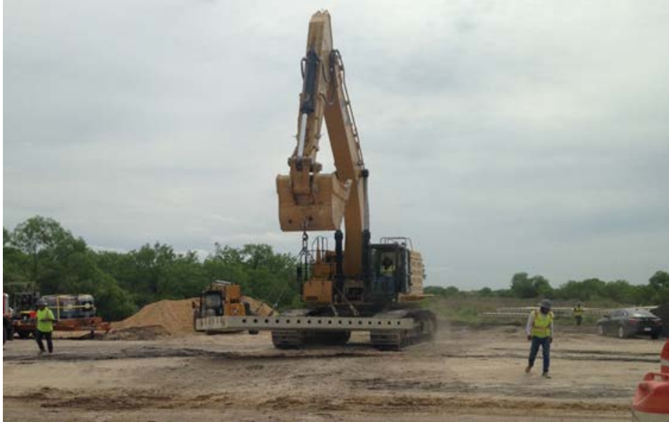
Figure 15. Photo. Panel being moved from the staging area using a backhoe.
