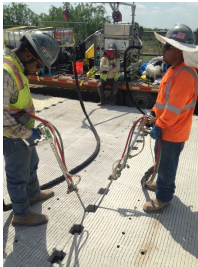
Figure 20. Photo. Grout being injected into the adjoining dowel-bar ducts and open slots.
