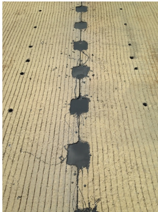
Figure 22. Photo. Completed grout placement along a joint.
