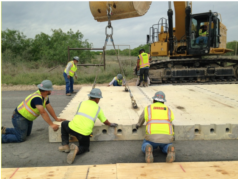
Figure 16. Photo. A panel being placed on the AC base.
