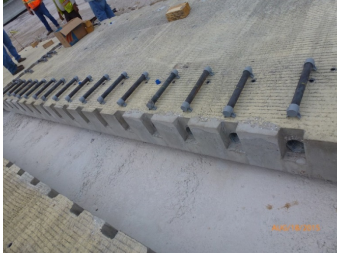
Figure 9. Photo. View of a typical panel with dowel bars ready to be placed in the ducts.
