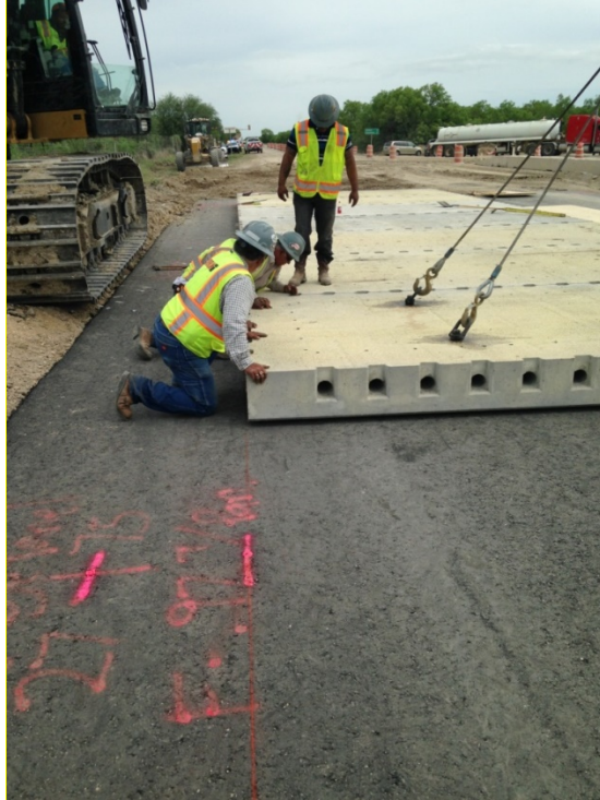
Figure 17. Photo. Panels being aligned with panel location markings on the AC base.
