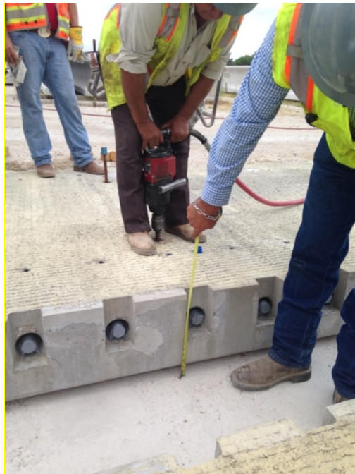
Figure 18. Photo. Engaging of the leveling lift system.
