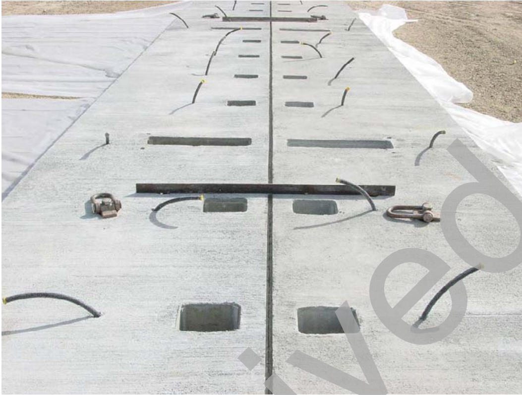
Figure 19. Photo. Typical joint panel at the fabrication plant prior to shipment.
