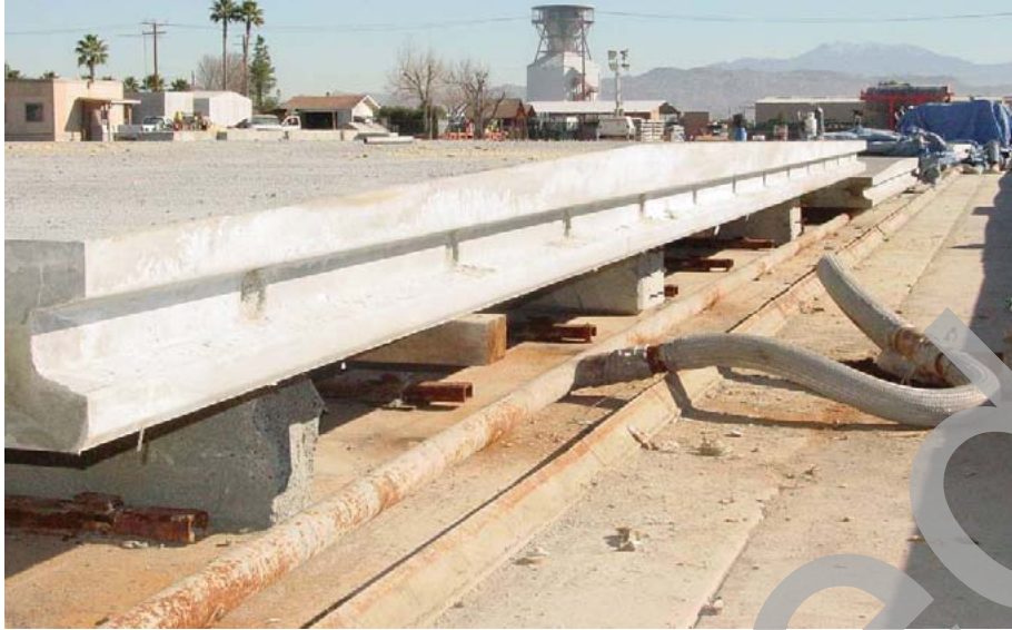
Figure 10. Photo. Precast panel at the fabrication plant after removal from the forms.
