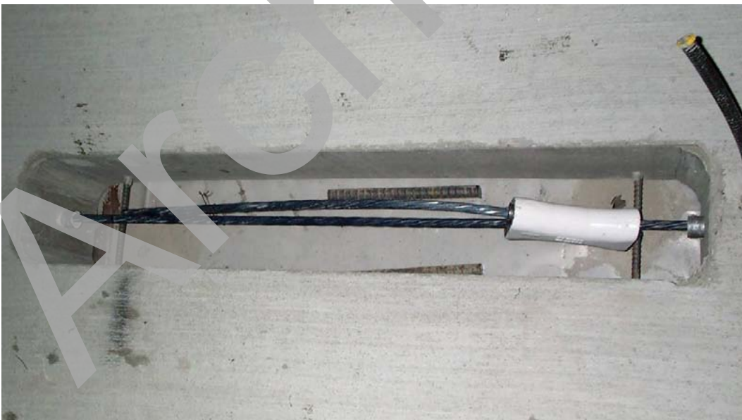
Figure 31. Photo. A “dogbone” coupler is used to splice the post-tensioning tendons together in the stressing pockets. The stressing ram tensions both tendons at the same time through the coupler.
