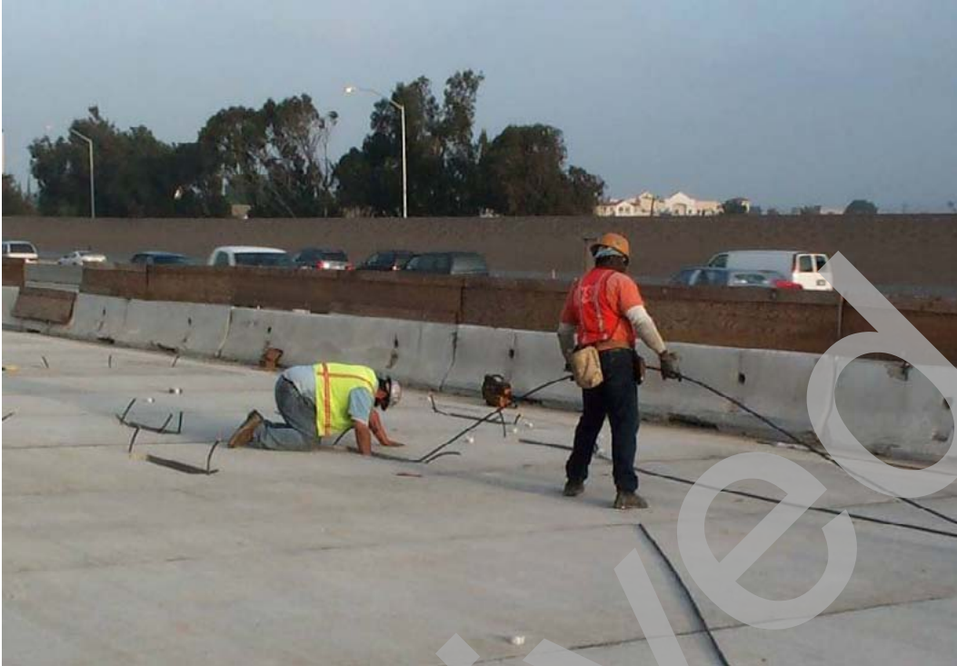
Figure 30. Photo. Workers feed the post-tensioning strands into the ducts at the central stressing pockets and push them through the ducts to the anchors.
