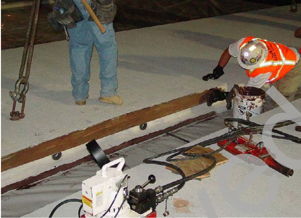
Figure 28. Photo. Workers apply epoxy to the joint prior to assembling the panels.
