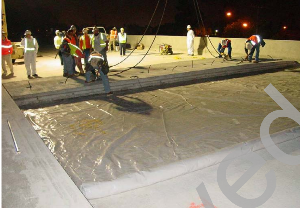
Figure 26. Photo. Workers detach the lifting lines from a precast panel. Note the polyethylene sheeting, rolled out just prior to placement of each panel.
