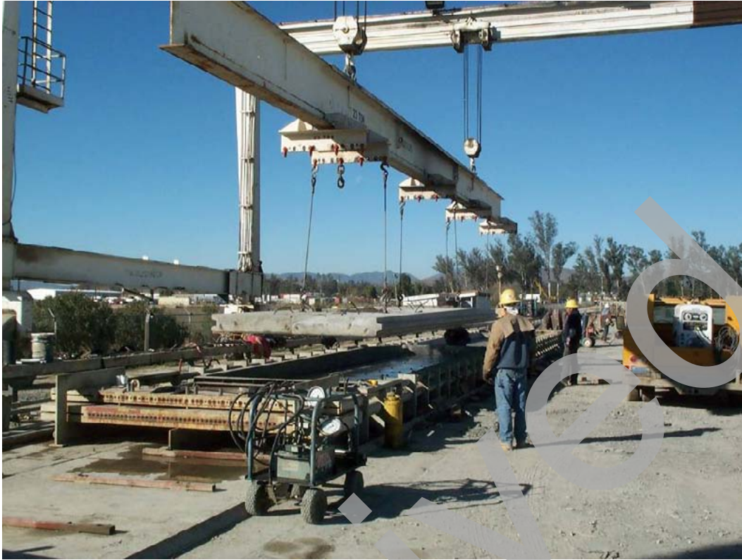
Figure 22. Photo. Removal of a panel from the forms after curing.
