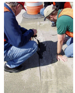
Pavement joint damage on an ASR-affected pavement near Mountain Home, ID
