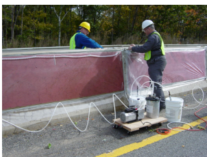
Vacuum impregnation treatment on ASR-affected highway barriers near Leominster, MA
