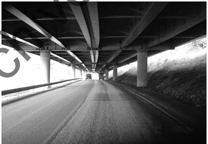
With each application, the county hopes to extend a road's service life another 5 to 6 years.
